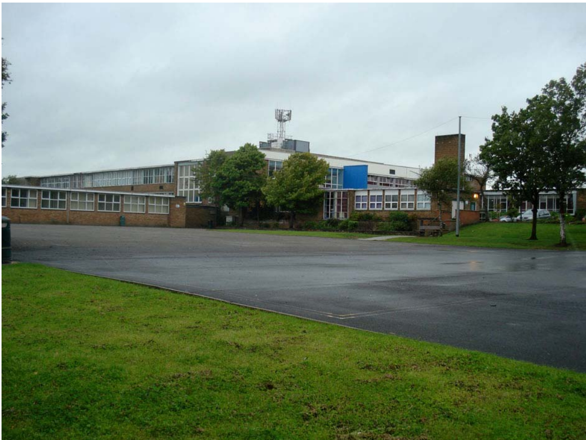
Plate 4: Playground at the south-east end of the school, looking north-west
