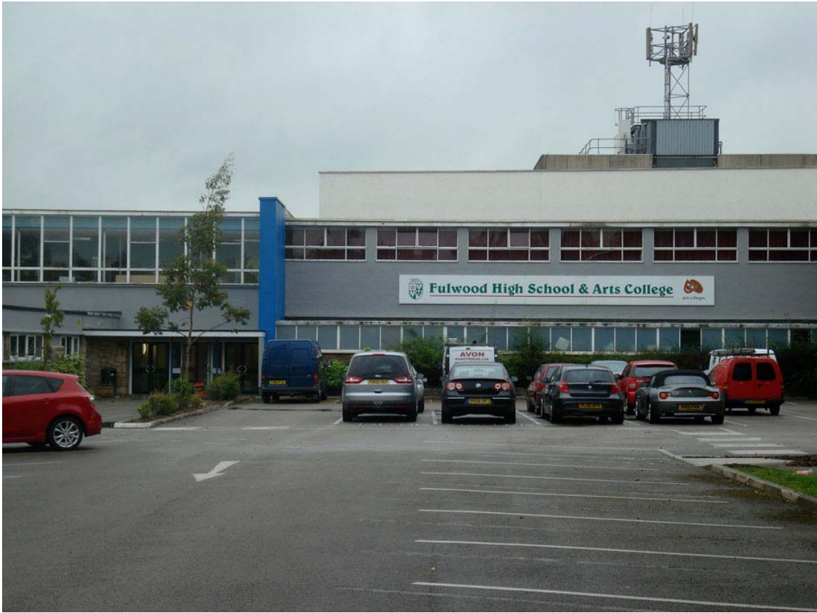
Plate 1: Front of the school, looking west
