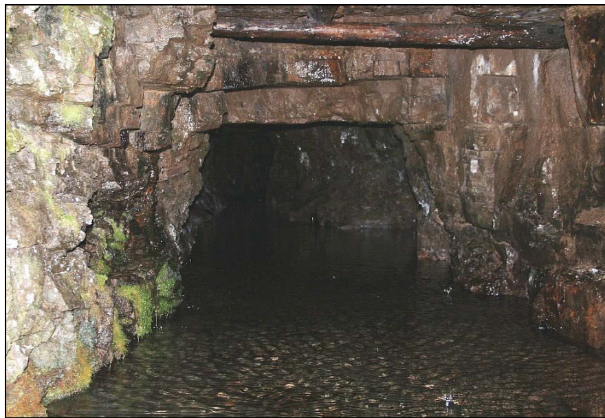
Plate 27: An open adit running into Wynch Bridge lead mine 3019
