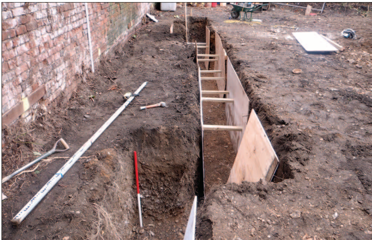
Plate 1: Excavated footings, shot taken from the south-west
