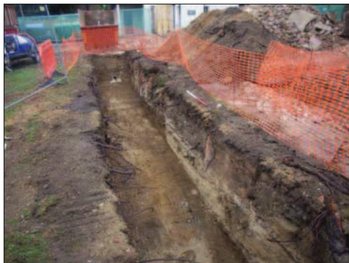
Plate 3: Trench 3 showing modern drains, looking NNE
