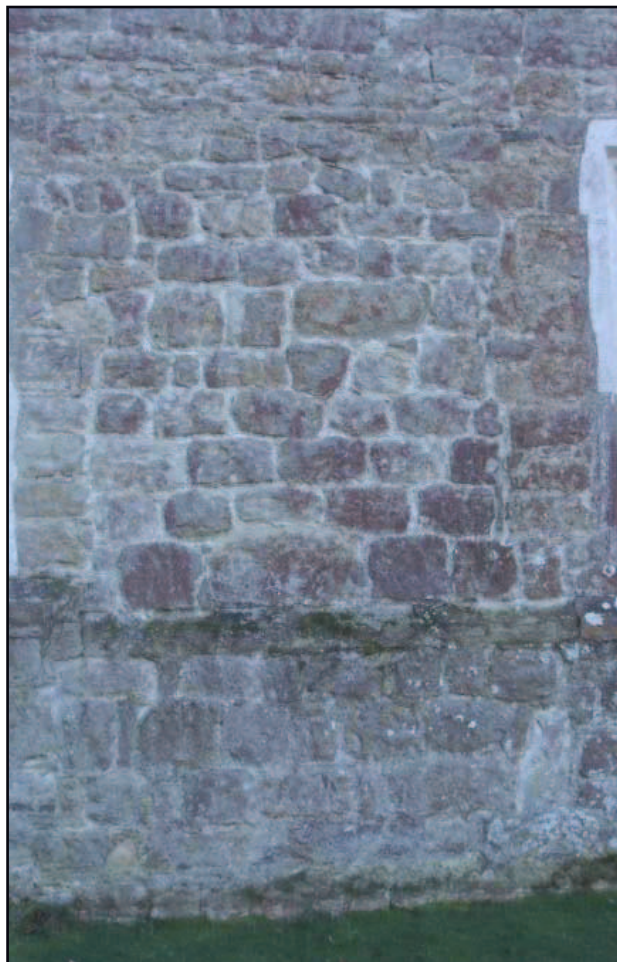
Plate 9: Blocked doorway in the north facade (west)
