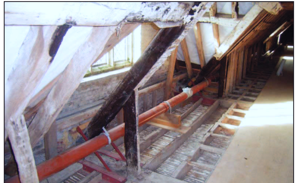
Plate 33: Blackened timbers due to fire
