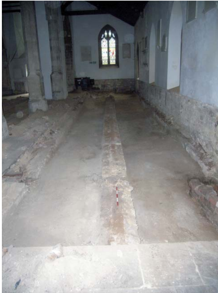
Plate 1: North aisle facing west
