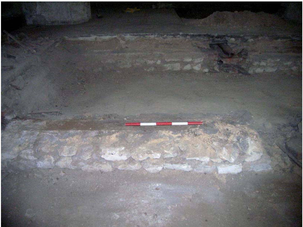
Plate 2: Sleeper wall of north aisle, facing south
