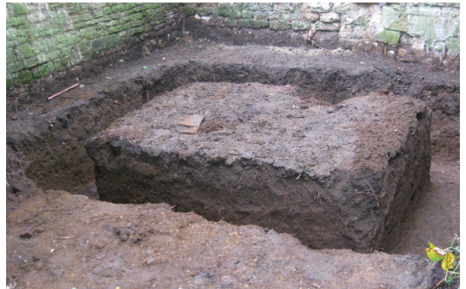
Plate 18: Excavation for Argonite store in Holywell Manor garden
