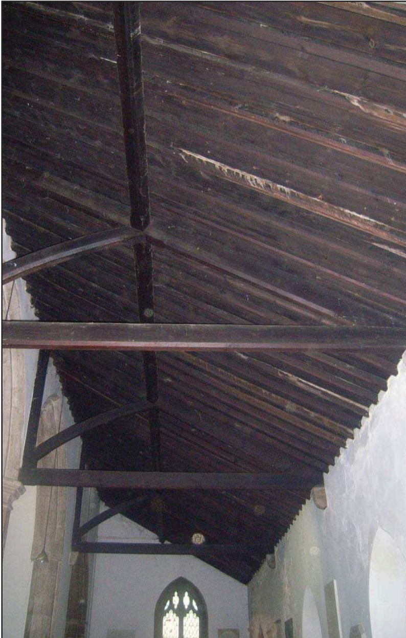
Plate 9: Roof of north aisle
