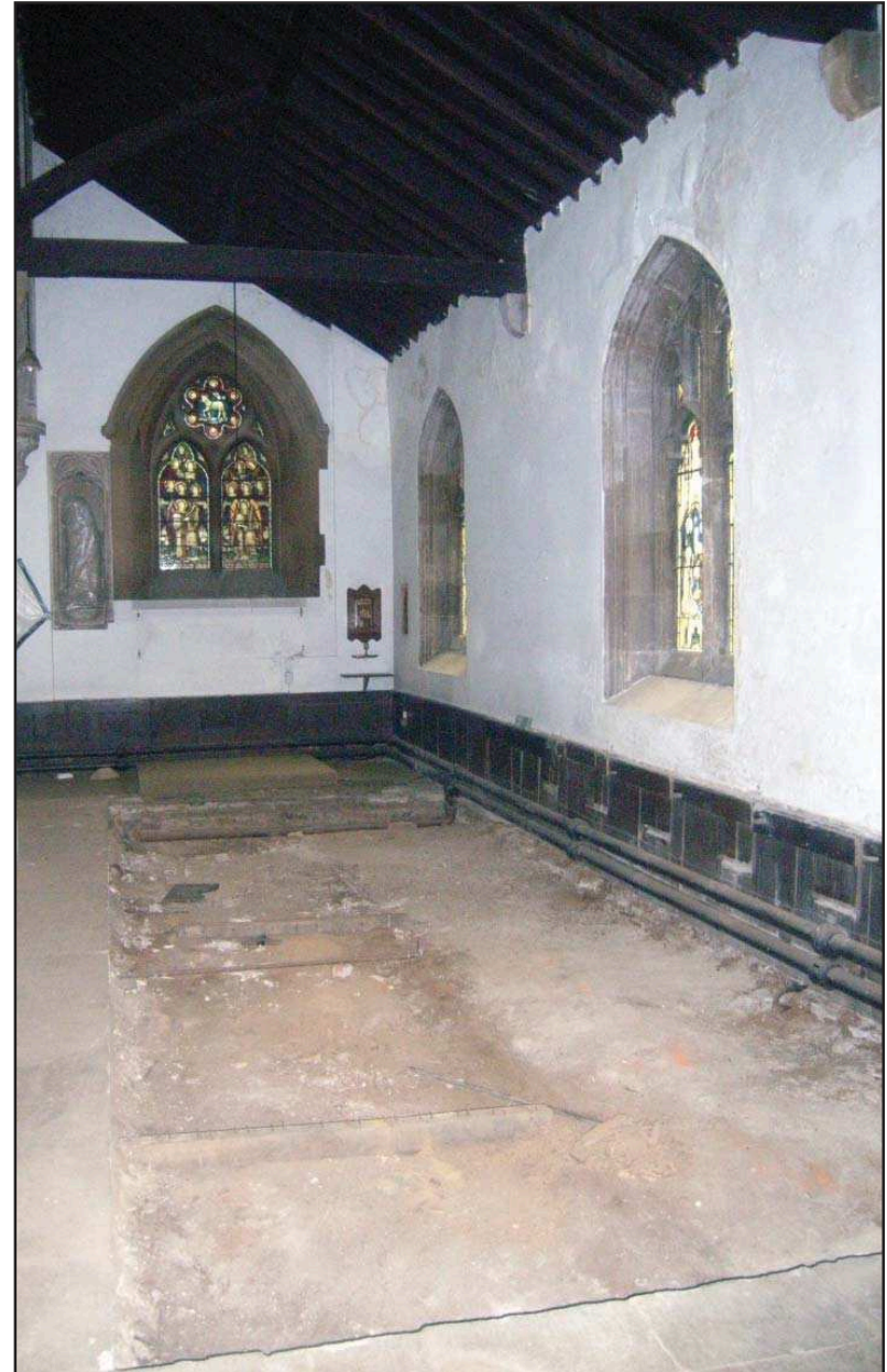
Plate 14: General view in Nave after removal of pews
