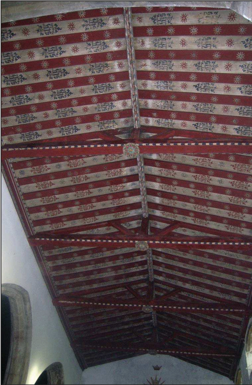
Plate 3: Late Victorian Nave roof
