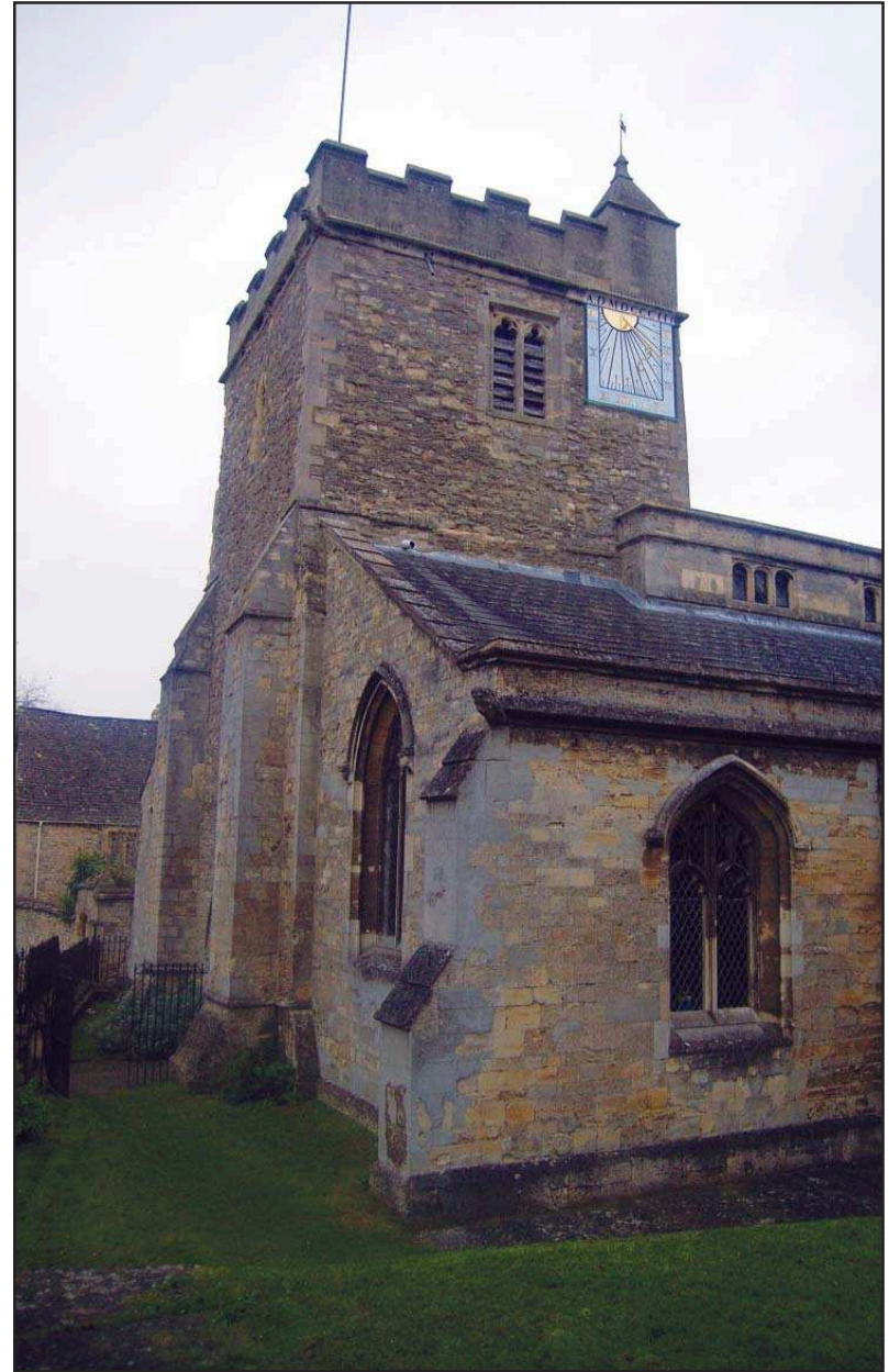
Plate 4: St Cross from the south-west
