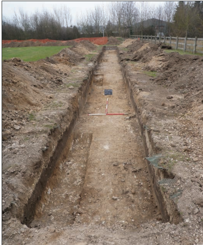
Plate 1: Trench 2, from the north-east, Context (16) in the foreground
