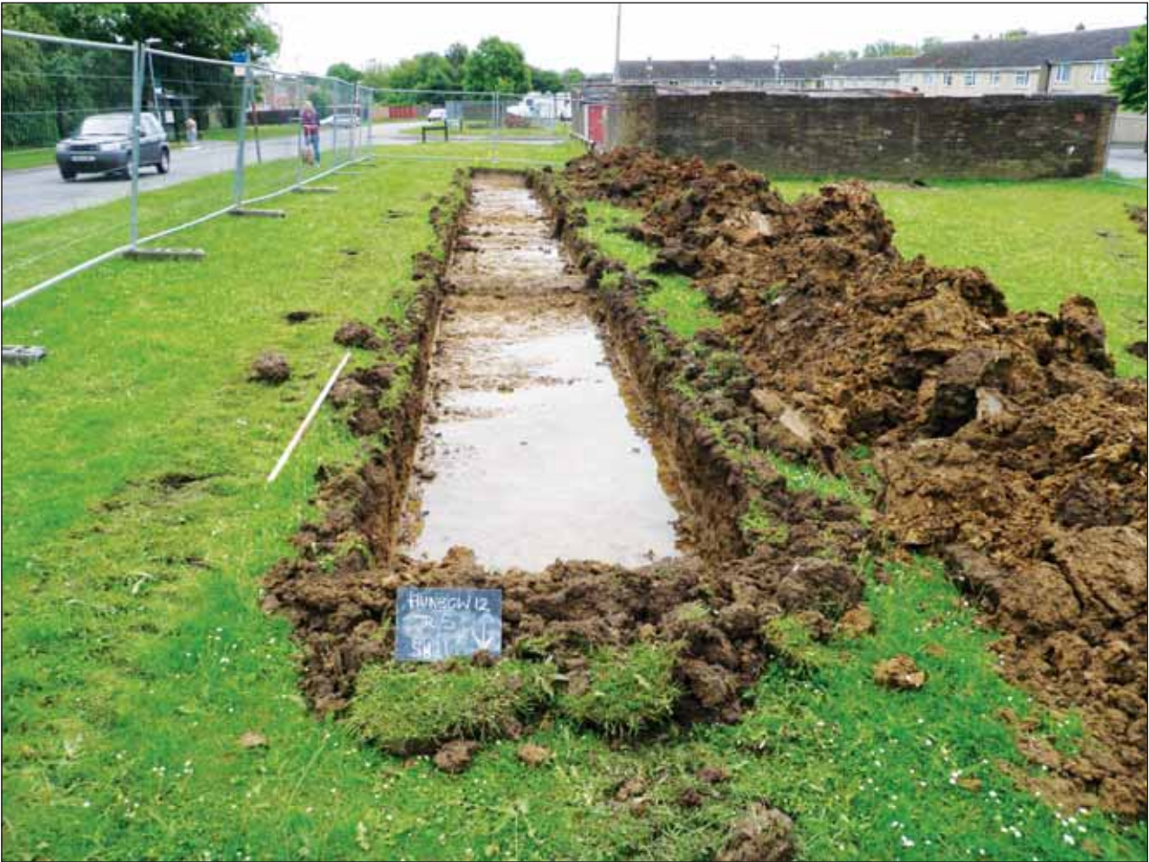
Plate 1: Trench 5, showing site conditions, facing south
