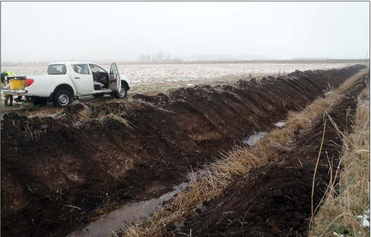
Plate 4: Trench 1 after cleaning northern face of drain, showing marl lake deposits
