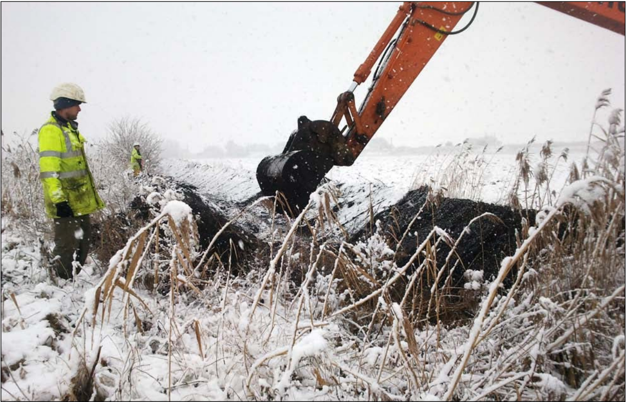
Plate 1: 'Trench' 1, cleaning modern drain to locate former course of Yaxley Lode
