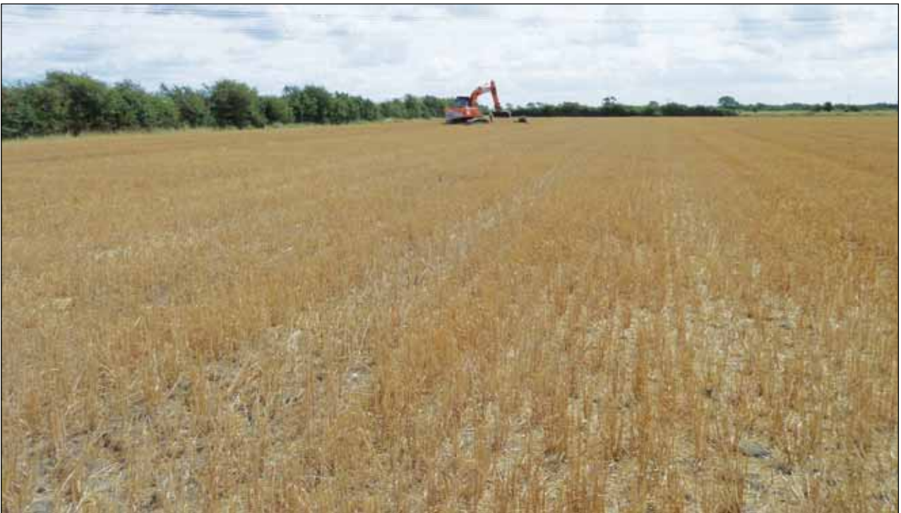
Plate 6: Working shot of site looking east
