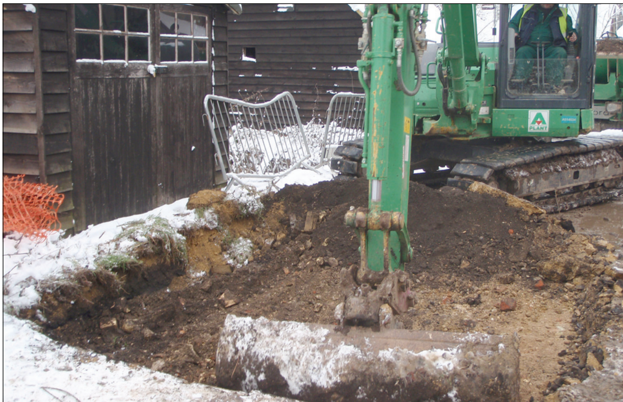
Plate 1: Machine digging area WS14
