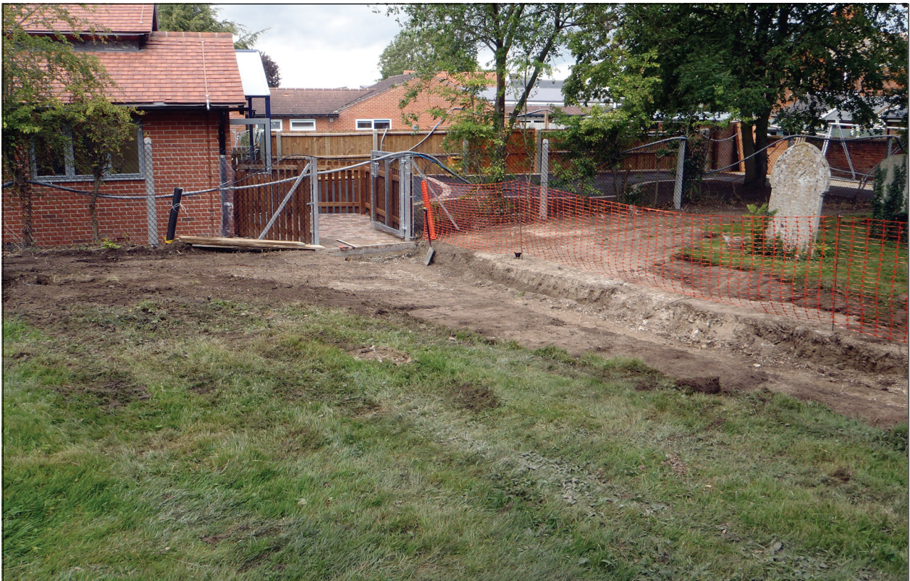
Plate 4: Area of ground reduction and grading of footpath, taken from the south-west.
