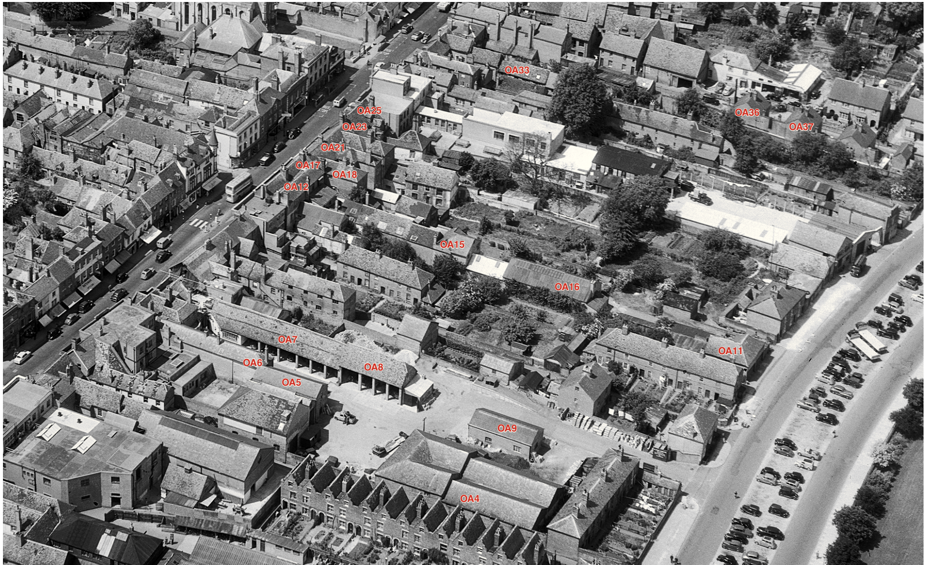
Figure F: Aerial photo of site from 1954
