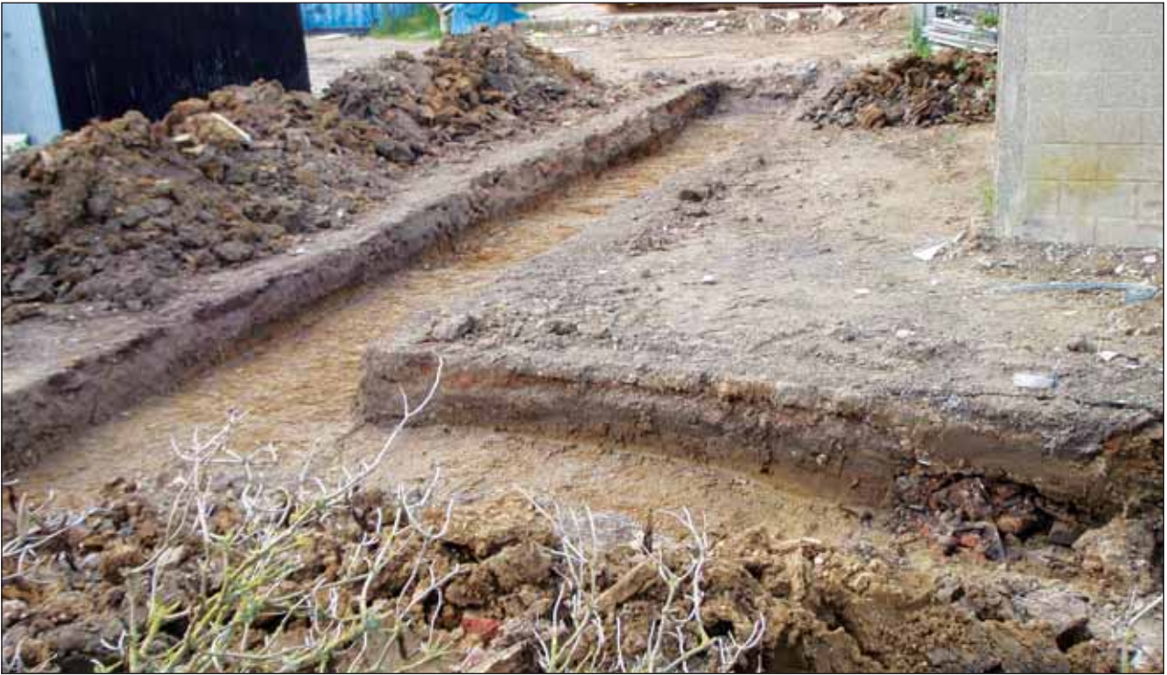
Plate 1: General view of Trenches 1 and 2 looking south-west
