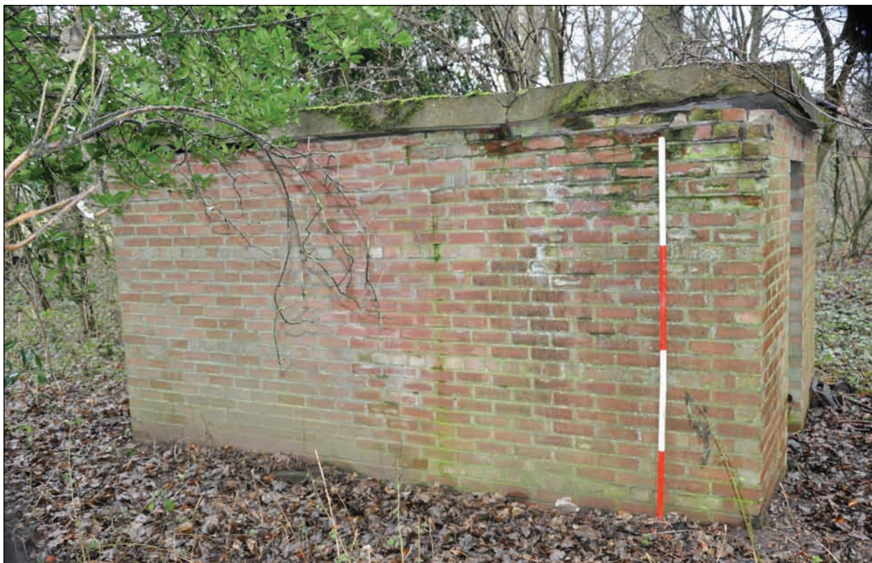
Plate 5: North west facing elevation
