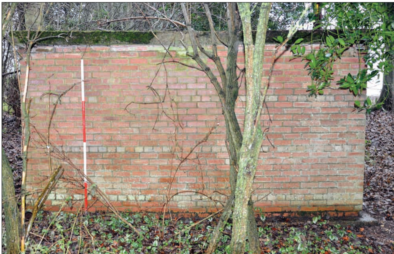
Plate 6: South east facing elevation
