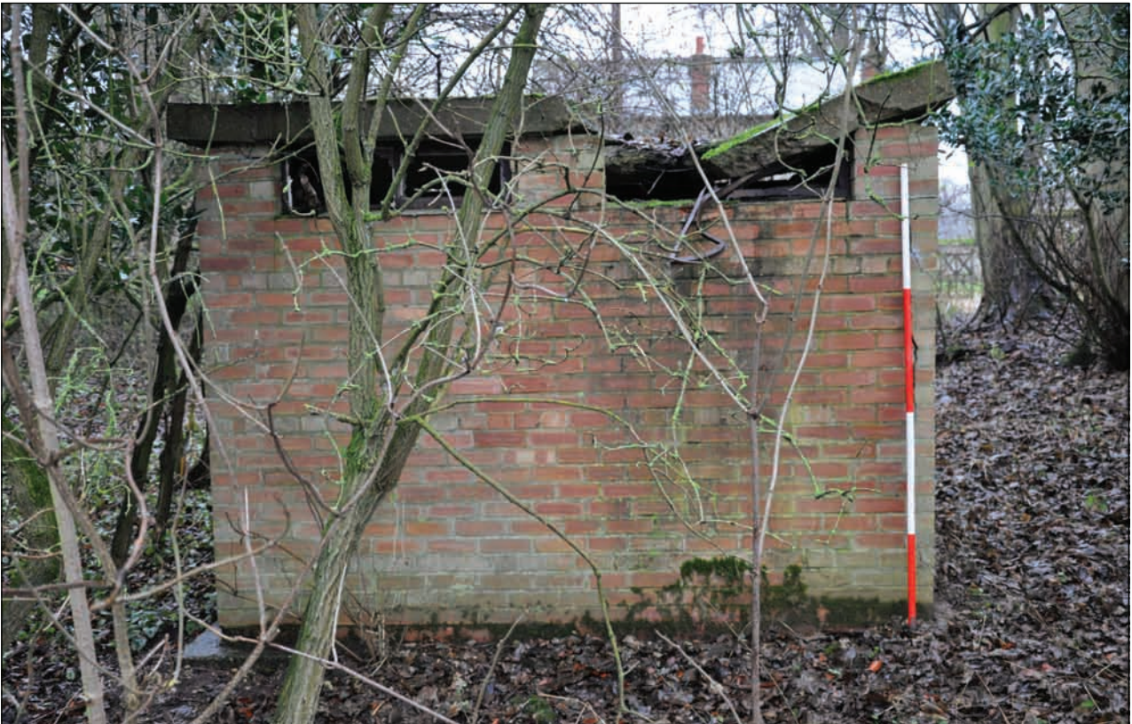
Plate 4: North east facing elevation
