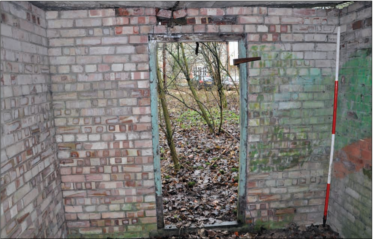
Plate 7: Internal view of brick building
