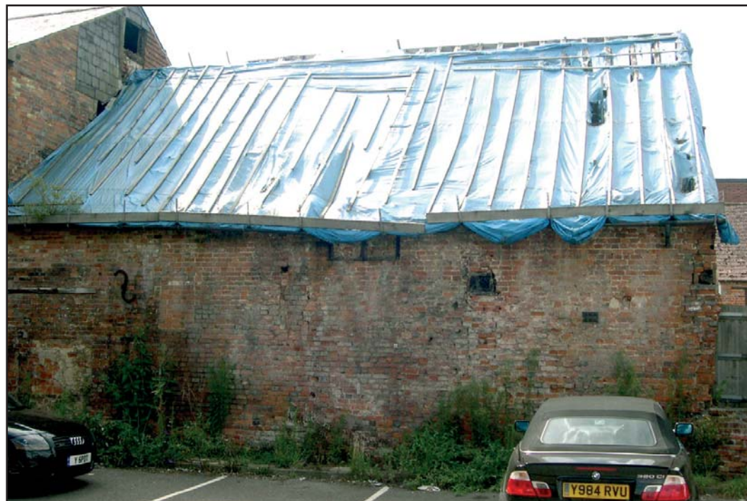
Plate 11: East elevation, two storey range
