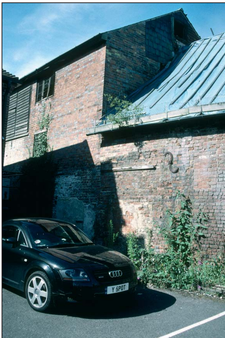
Plate 10: East elevation, three storey range
