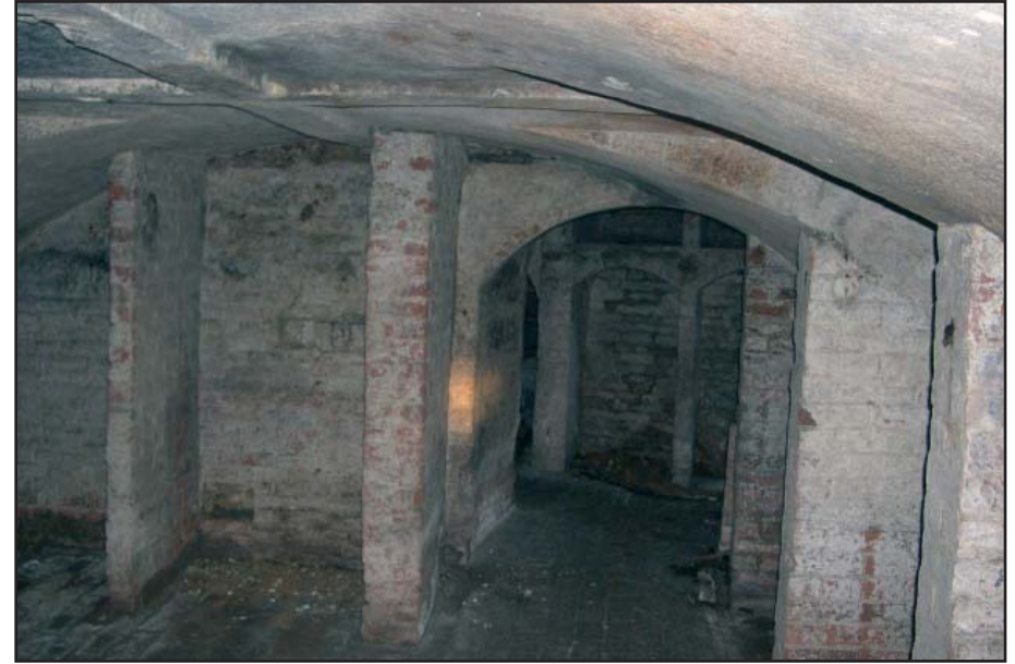
Plate 23: Cellar beneath 2-storey range
