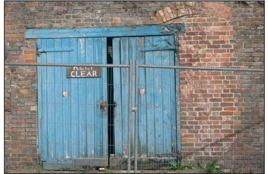
Plate 2: West elevation, three storey range
