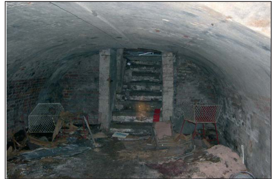
Plate 25: Southernmost cellar with access steps to off-license
