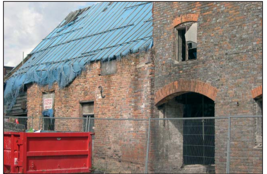
Plate 7: West elevation, two storey range
