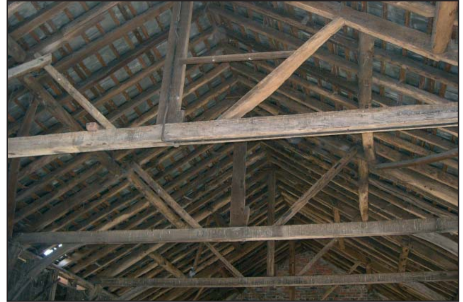
Plate 15: Roof of 3-storey range from north end
