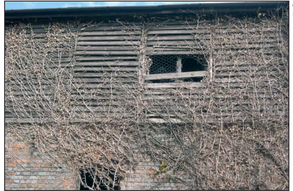
Plate 6: West elevation, wood louvres
