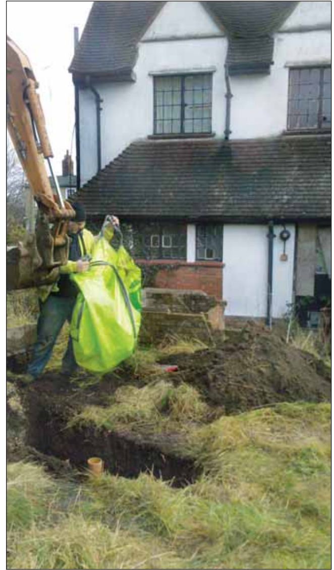
Plate 4: View of infiltration Pit 1 with No. 44 in the background (from west)
