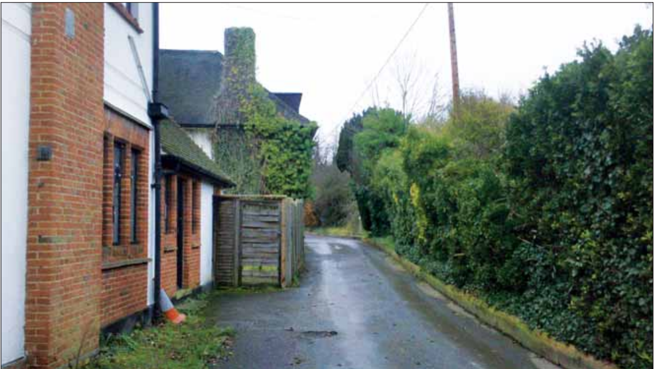
Plate 14: View along main access to/from the maternity ward with the former railway cutting to the north (right of picture)
