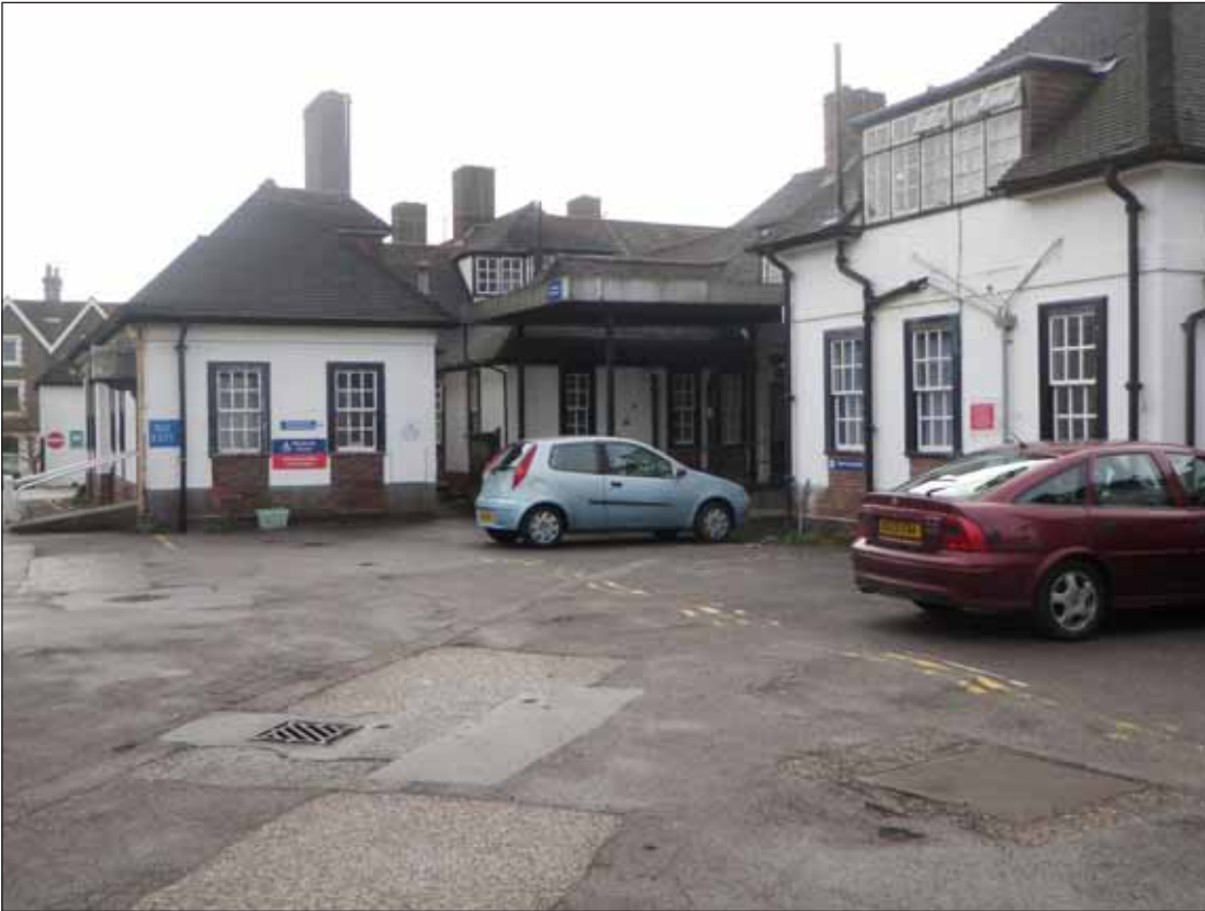
Plate 9: View across parking area to front of main hospital building showing drains etc
