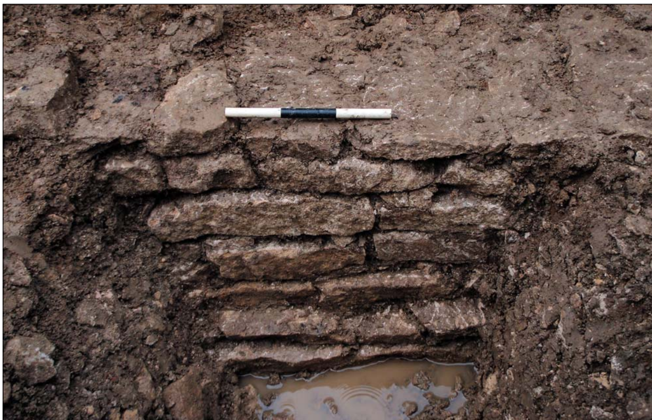
Plate 3: Section of exposed wall (6)
