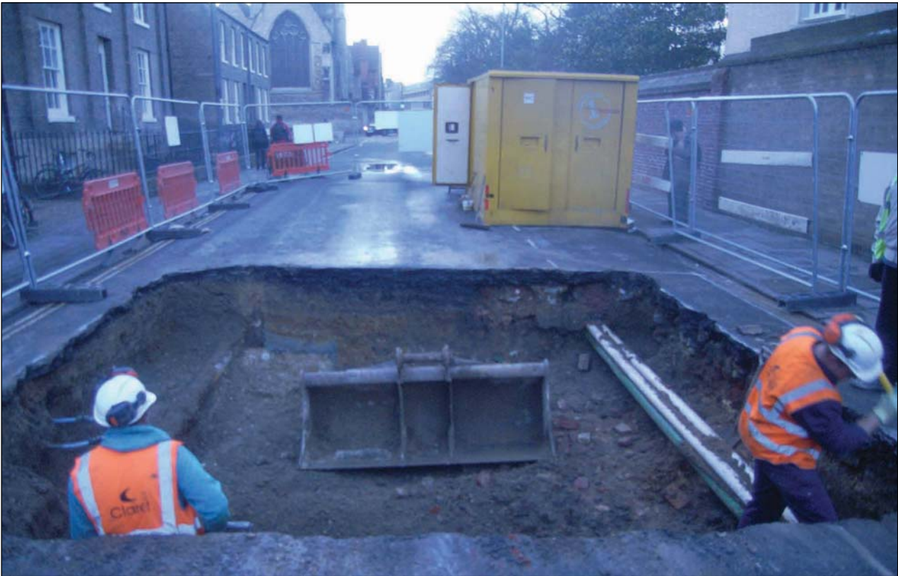
Plate 1: Initial ground investigation (looking west)
