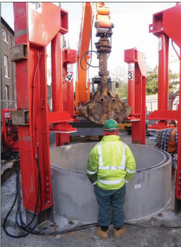
Plate 2: Ground works using a cassion
