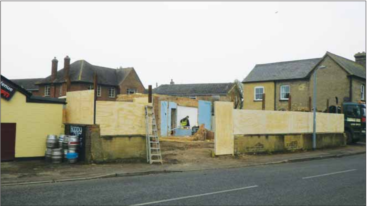
Plate 5: The site looking north-west
