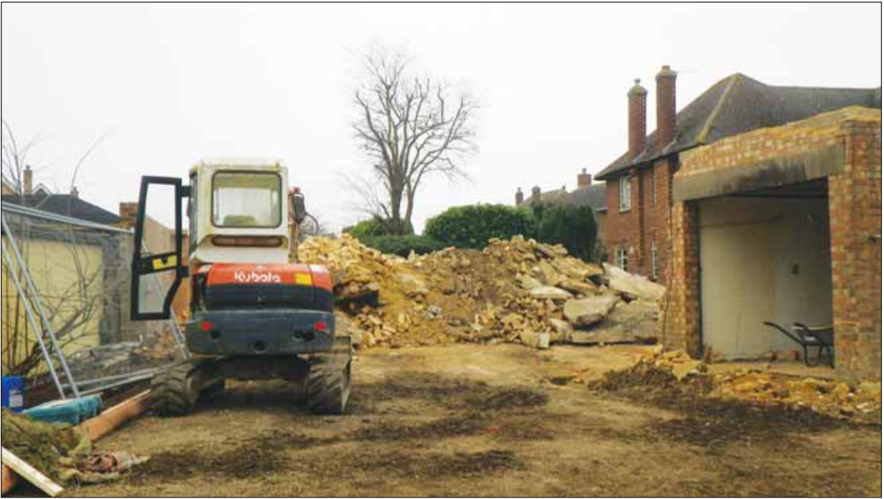
Plate 3: The site looking south
