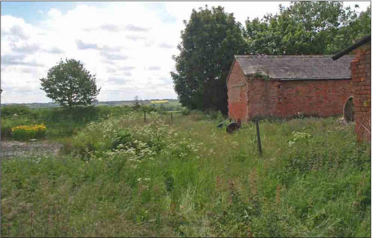
Plate 7: Middle Lodge Farm buildings and pond. From the west
