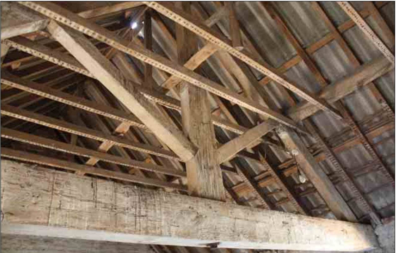
Plate 22: Detail of king-post roof, Building B (ii)
