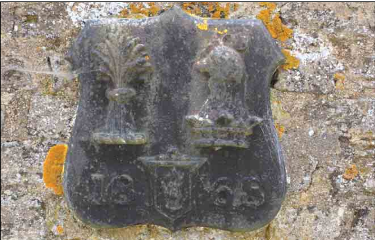
Plate 4: Date plaque with Fermor-Hesketh crest on Building B, north-facing elevation
