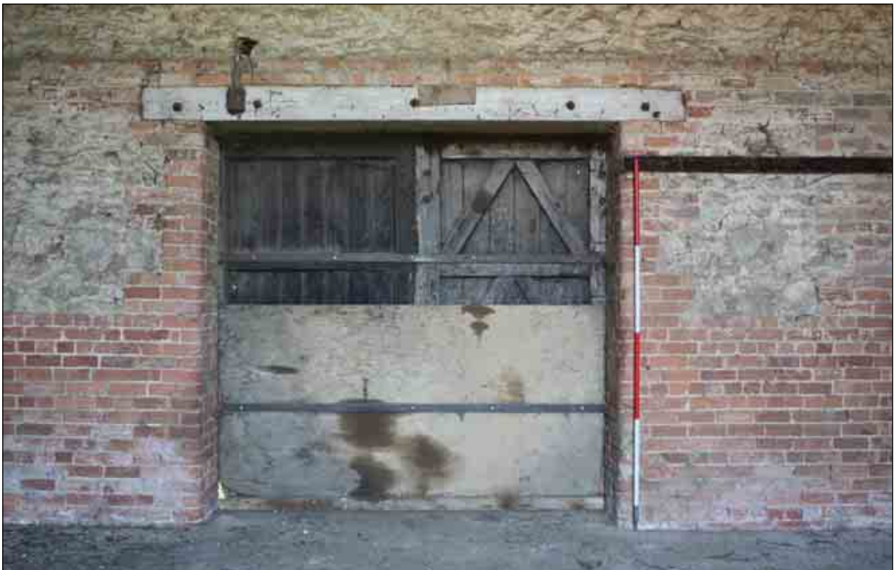
Plate 27: Interior view of loading doors, Building B (iii)
