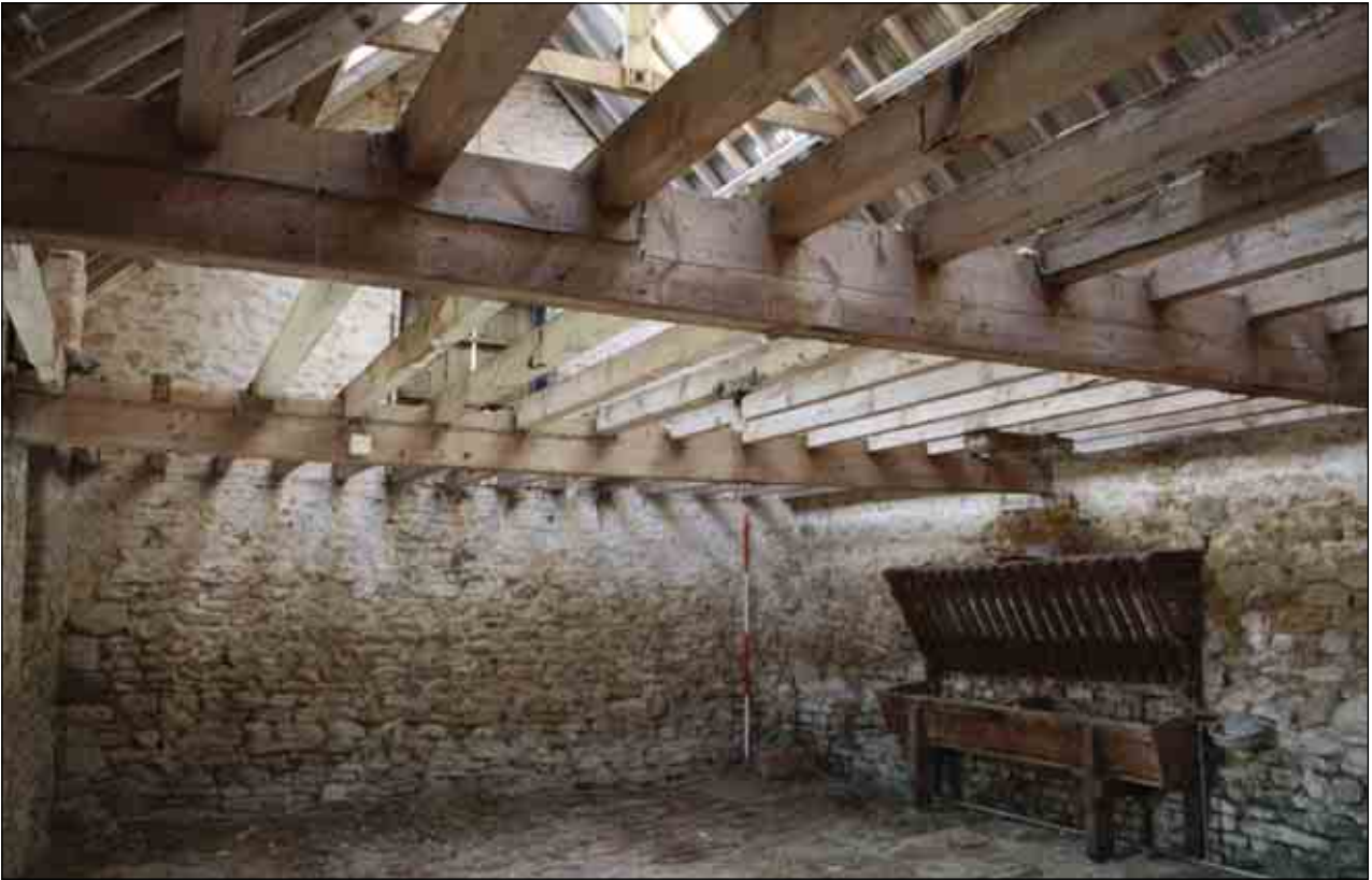
Plate 44: Interior view, Building D (i), southern end
