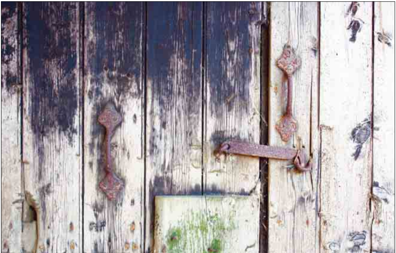
Plate 7: Detail of iron fittings on doors, Building B
