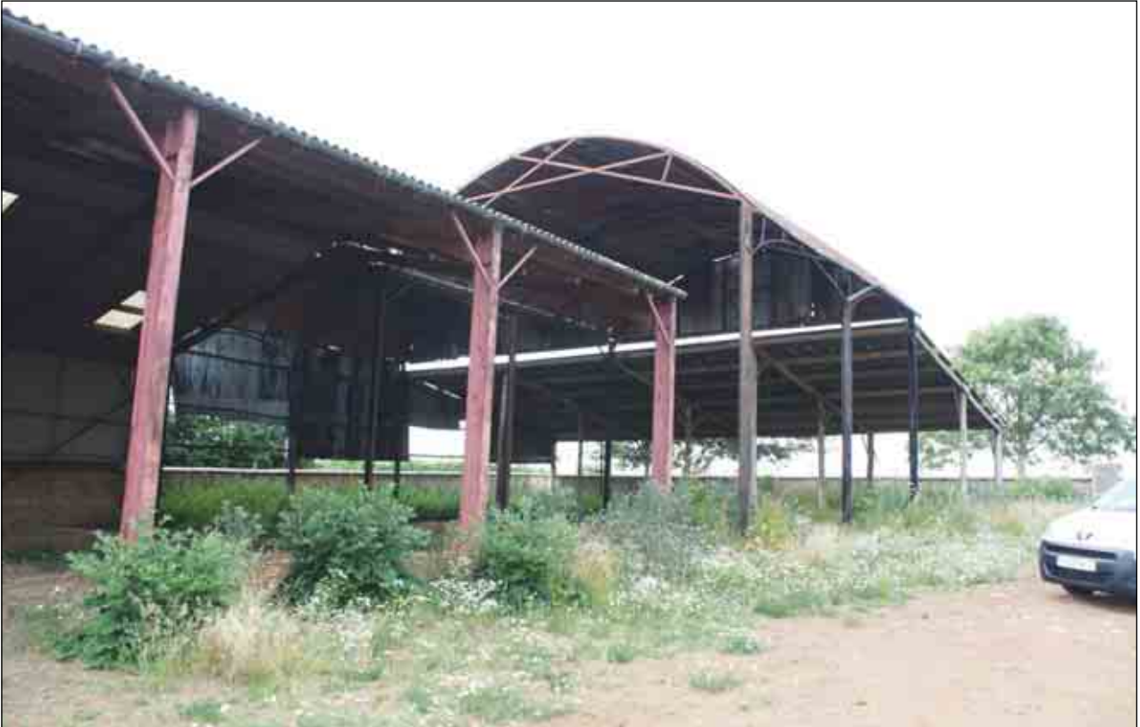
Plate 1: Building A, from south-east
