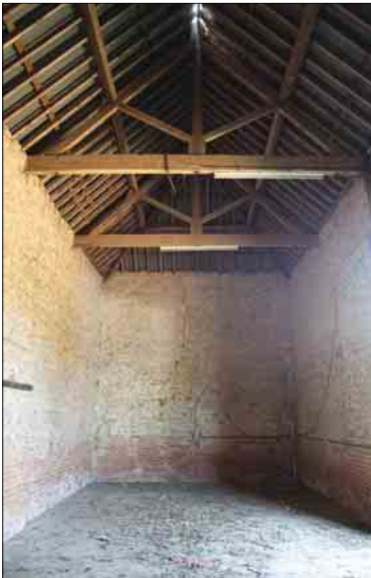
Plate 25: Interior view, Building B (iii)
