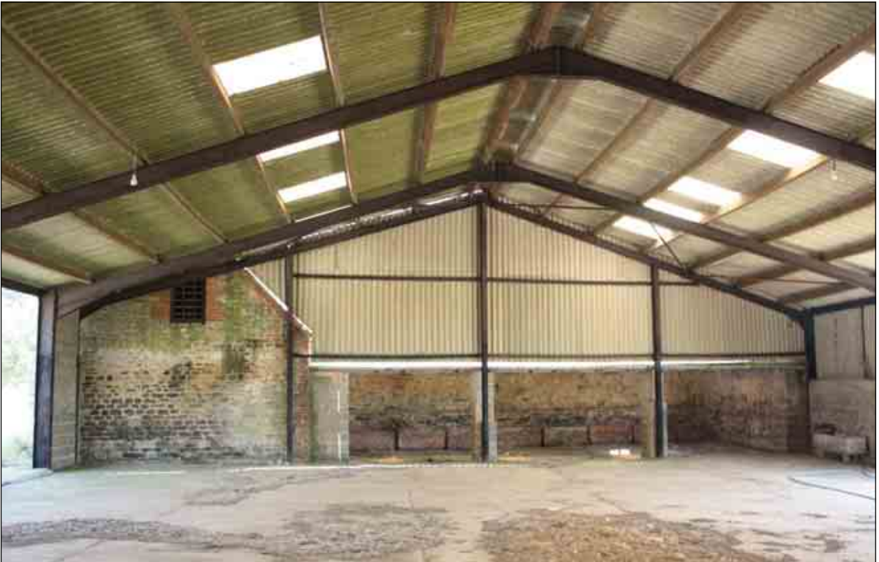
Plate 62: Building E, west-facing elevation as viewed from within Building F
