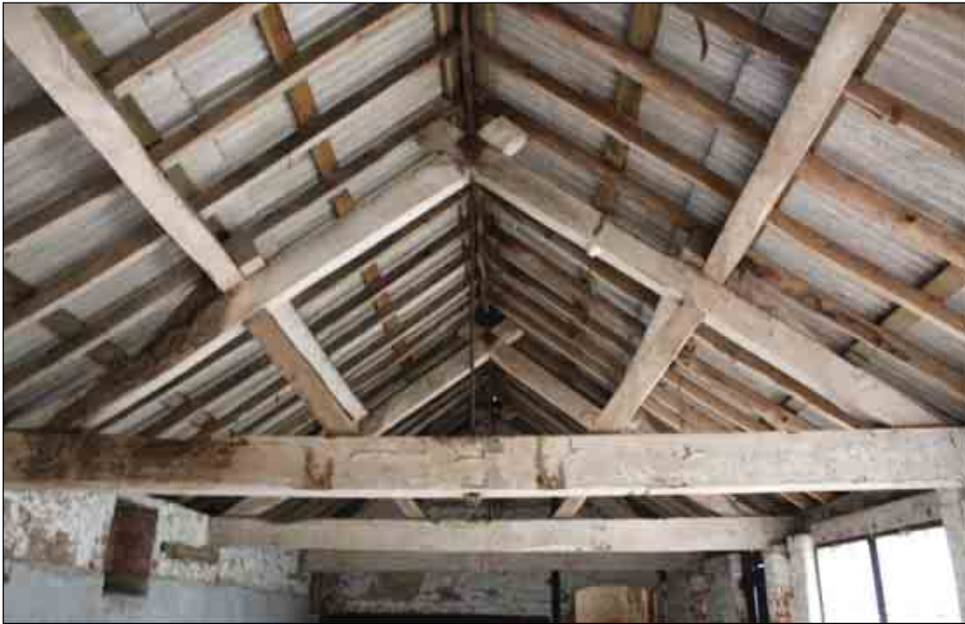
Plate 50: Detail of roof structure, Building D (ii)
