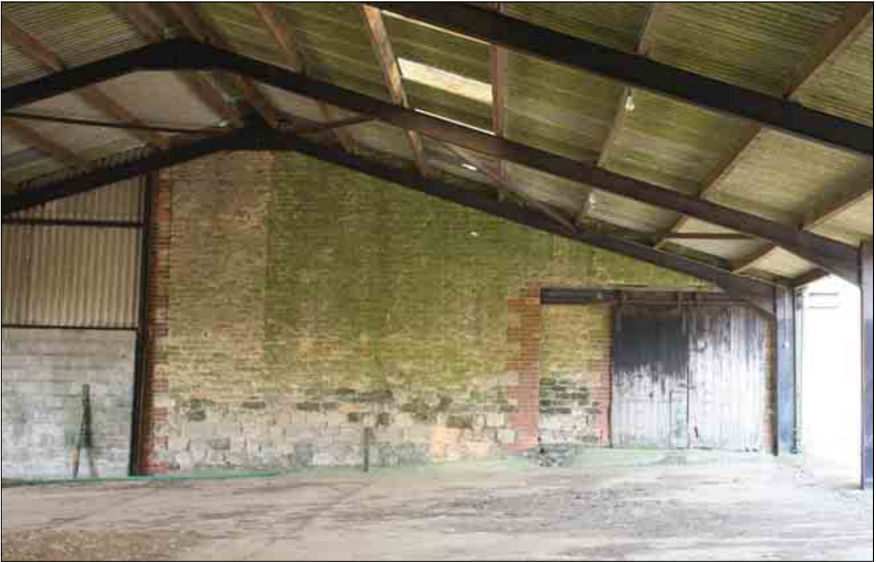
Plate 5: Building B, southern end of east-facing elevation
