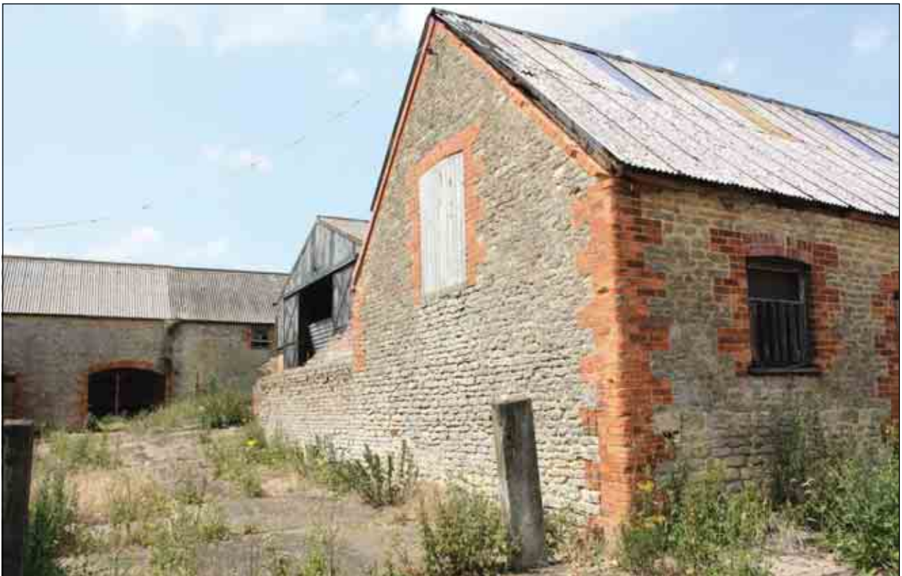
Plate 39: Building D, south-facing elevation of north-south range
