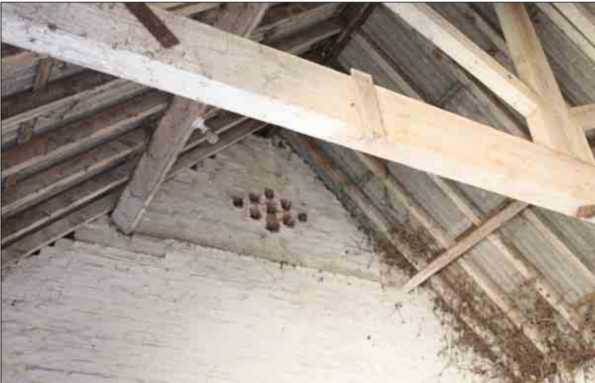
Plate 67: Detail of ventilation voids, Building E (i)
