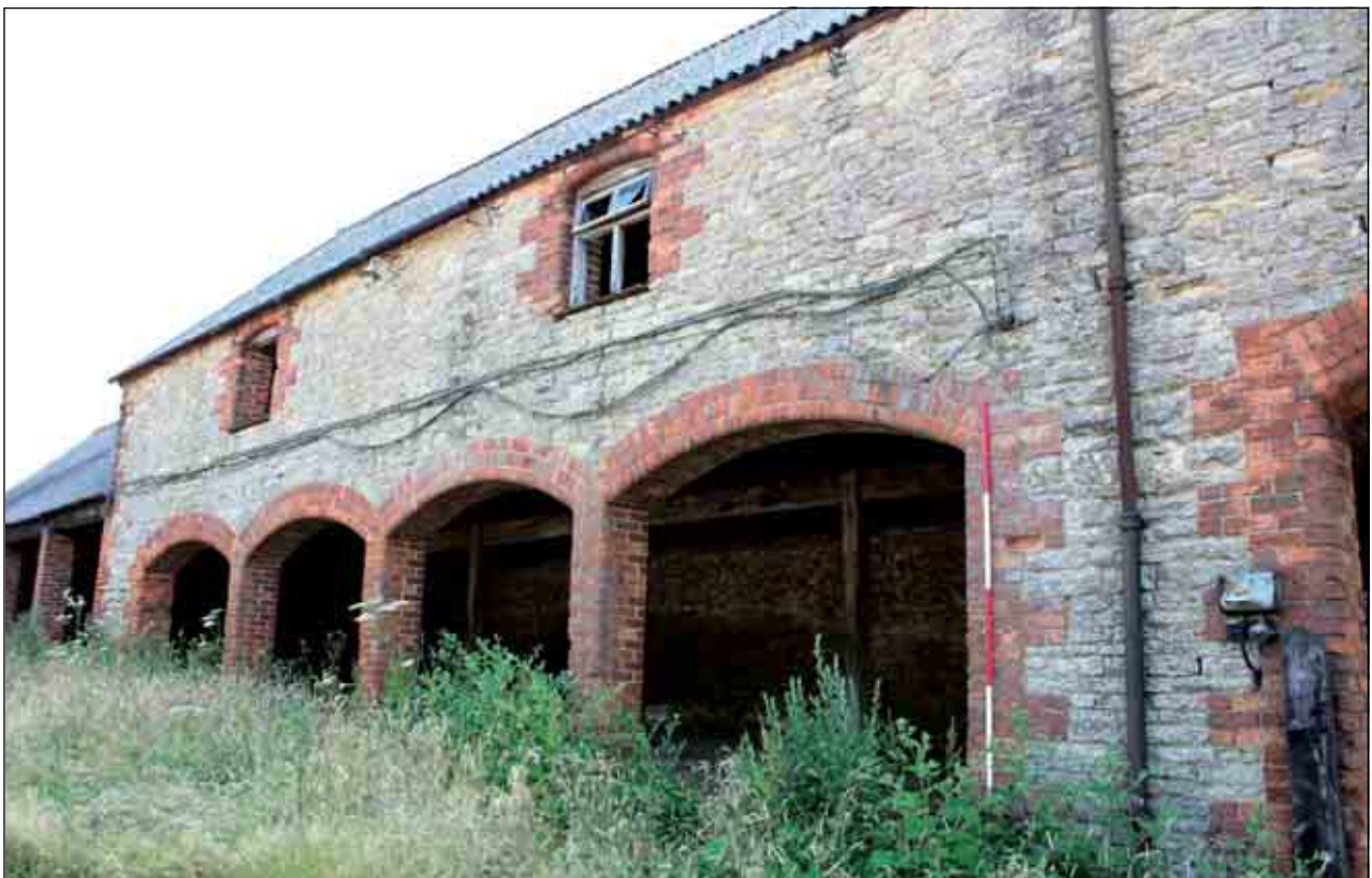
Plate 12: Building B, west-facing elevation
