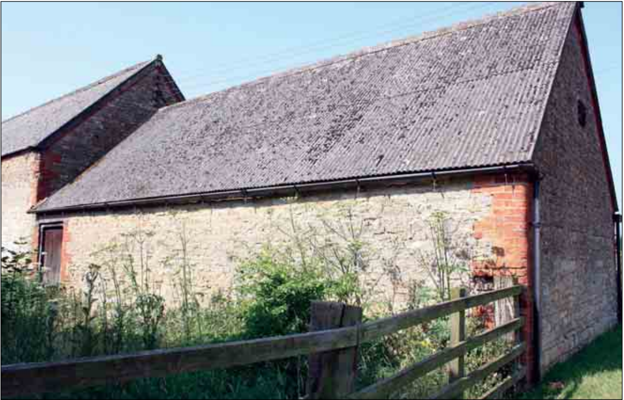
Plate 9: Building B, northern end of east-facing elevation
