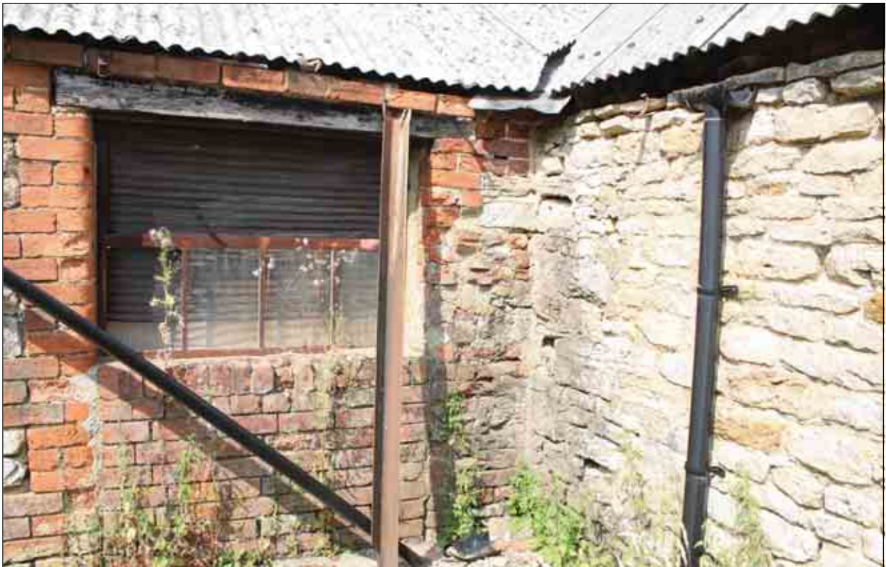
Plate 38: In-filled doorway, Building D, south-facing elevation
