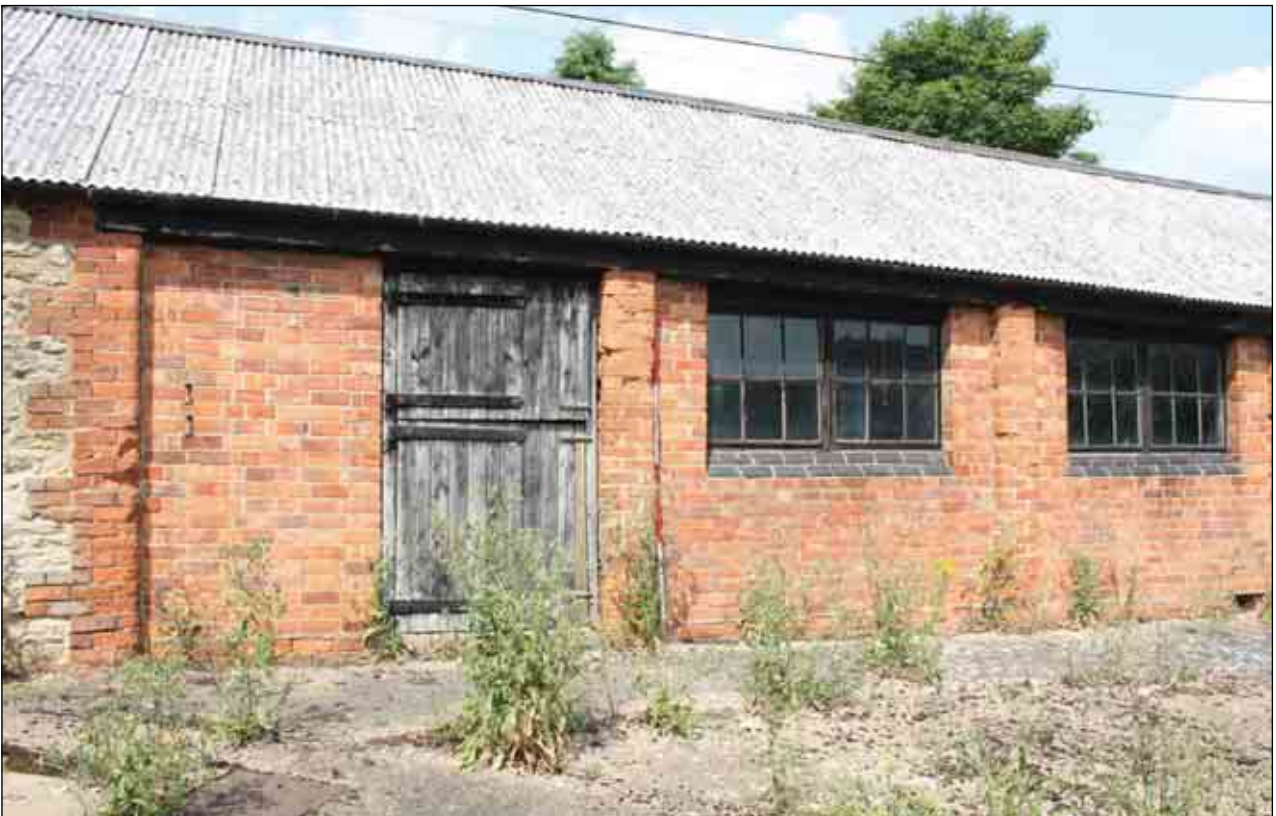
Plate 41: Brick in-fill, Building D south-facing elevation
