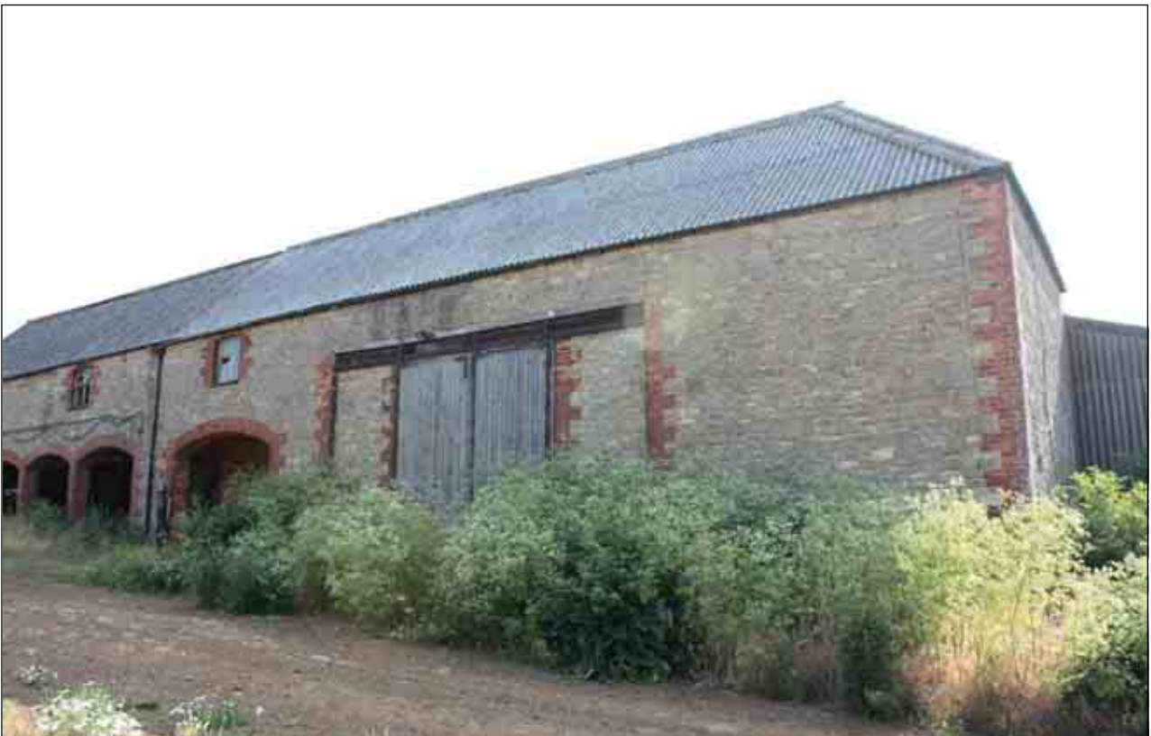
Plate 14: Building B, southern end of west-facing elevation
