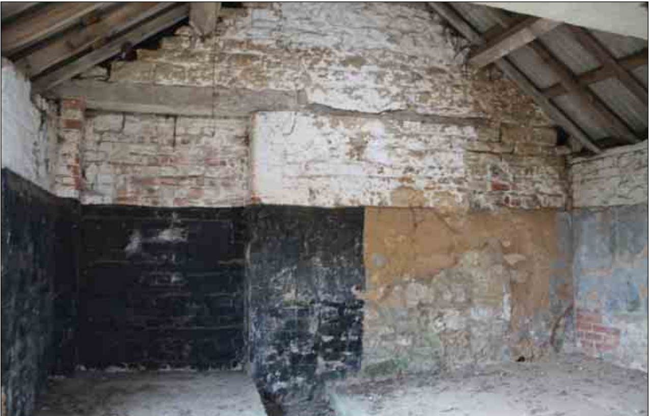
Plate 57: Blocked-up doorway, western end of Building D (iii)
