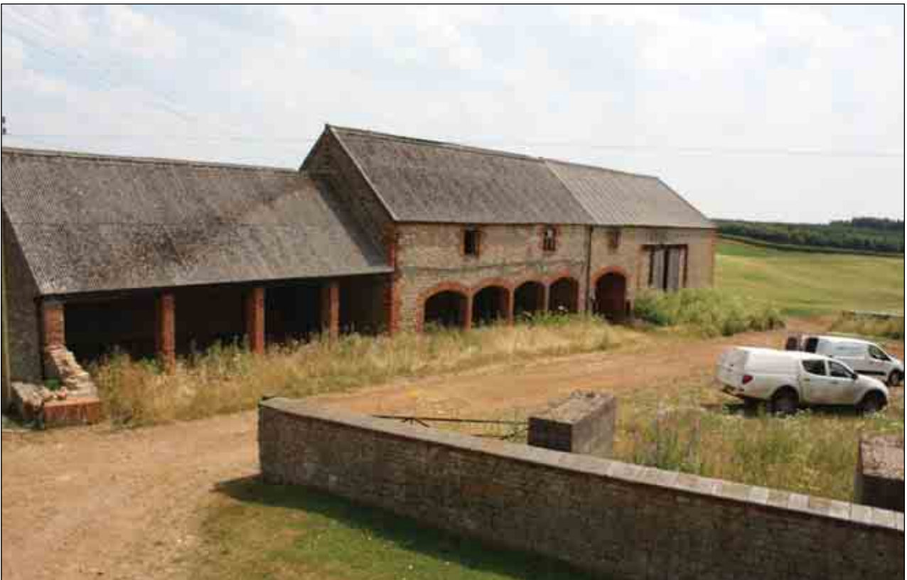
Plate 2: Building B, west-facing elevation
