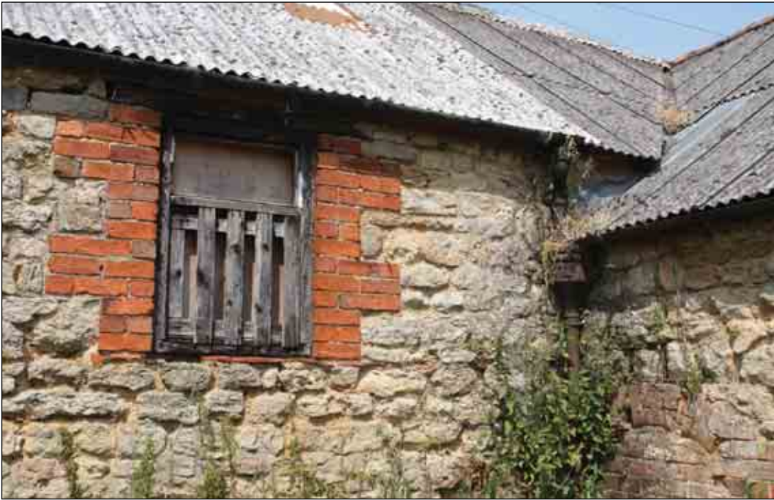
Plate 42: Ventilation opening on Building D, south-facing elevation
