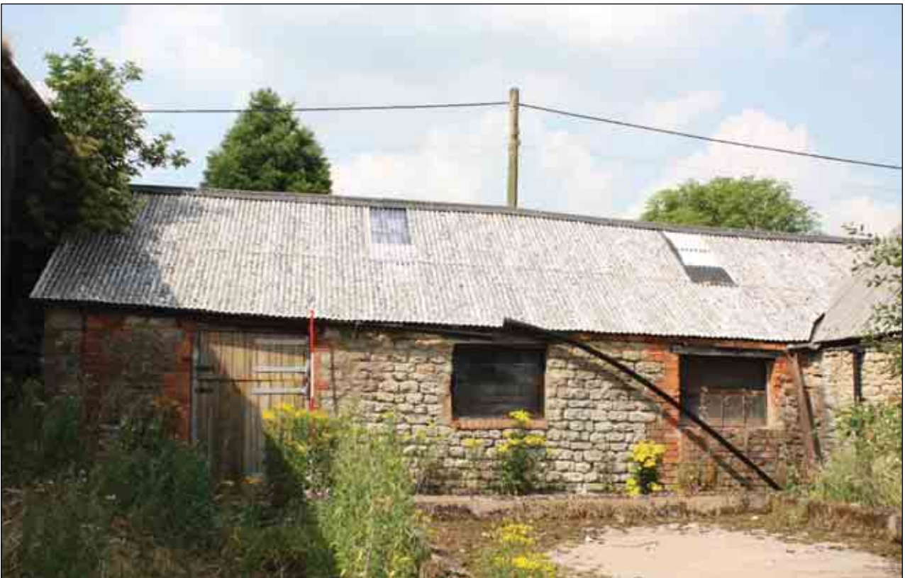
Plate 37: Building D, western end of south-facing elevation
