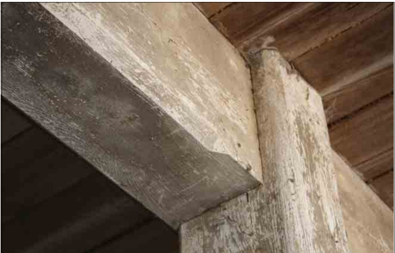
Plate 18: Detail of chamfered beam, Building B (ii)
