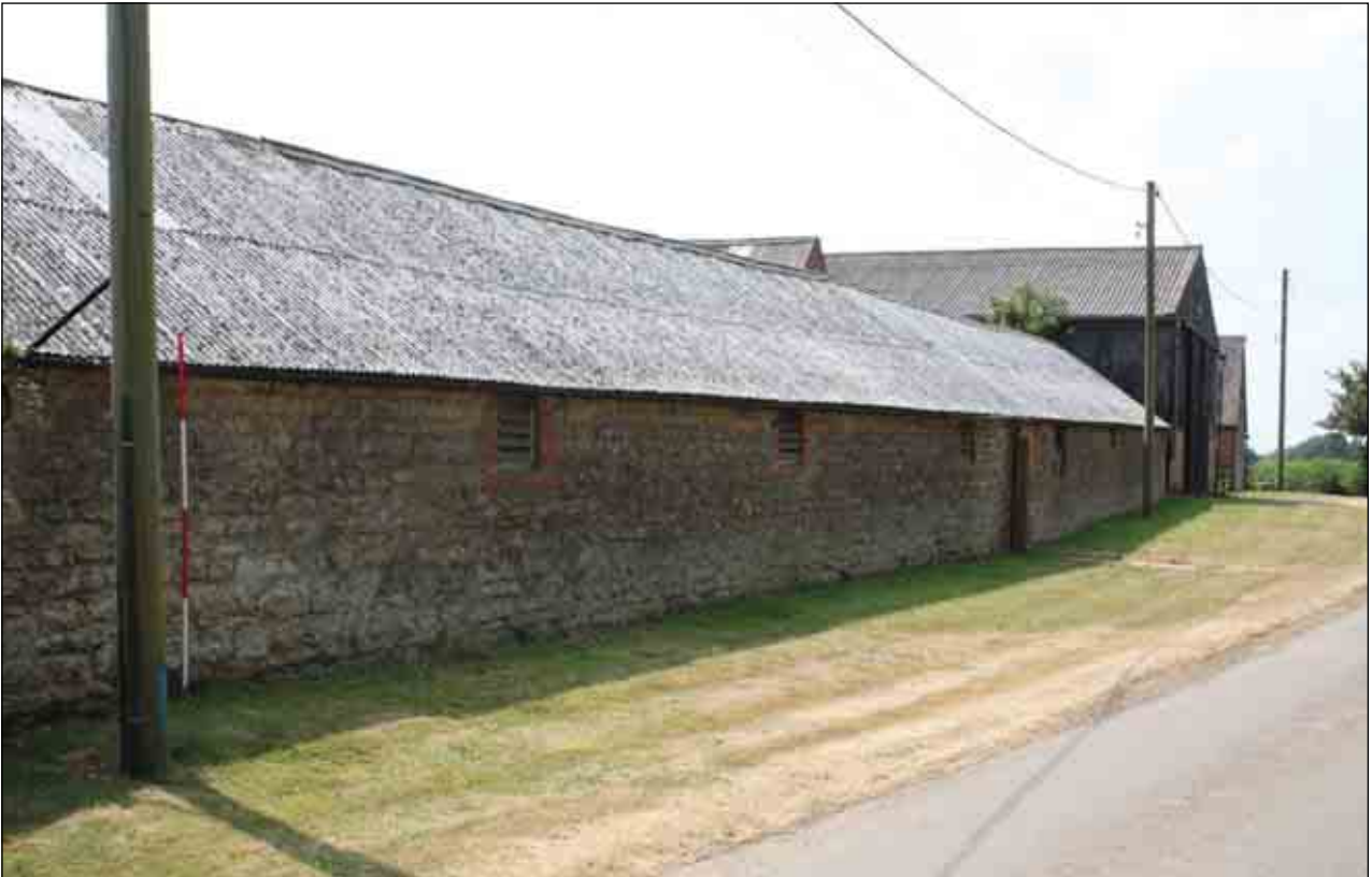
Plate 30: Building D, north-facing elevation
