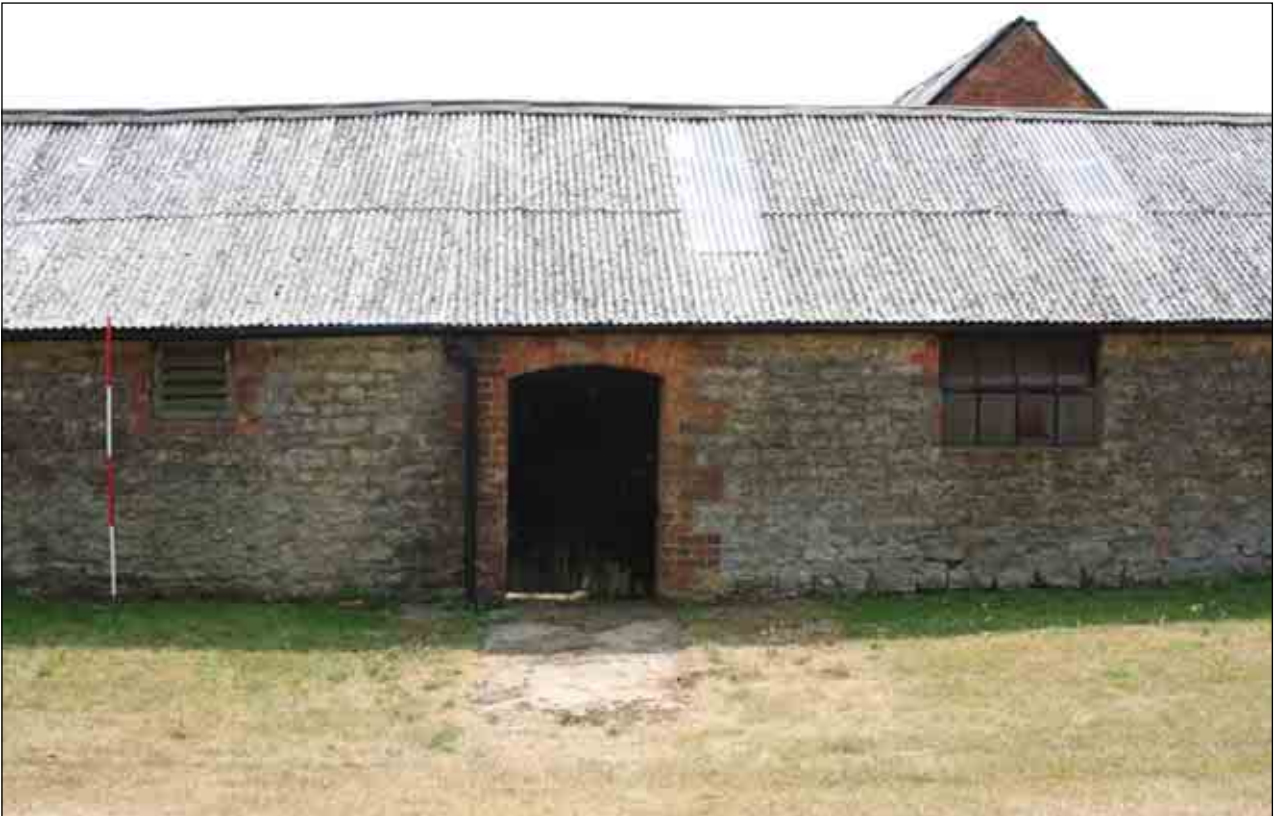
Plate 32: Doorway, window and ventilation opening on Building D, north-facing elevation
