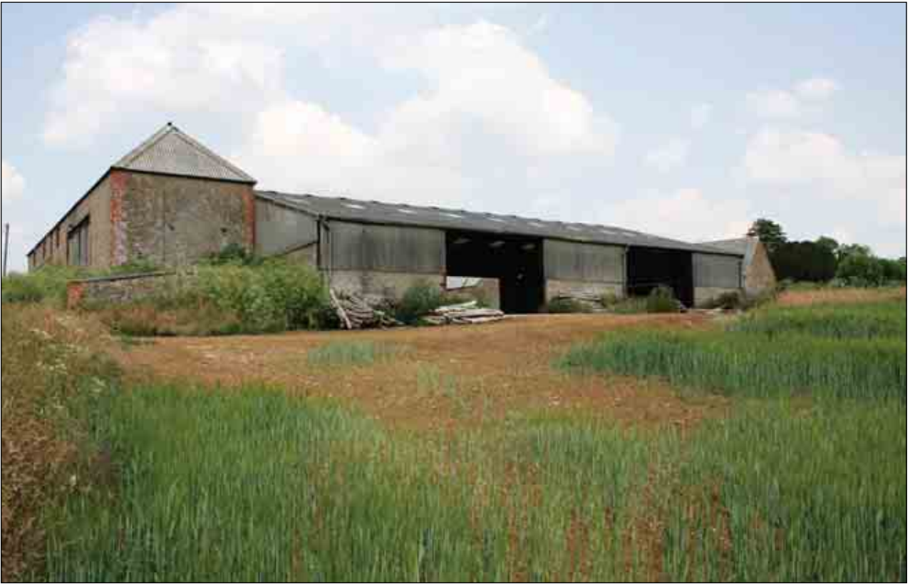
Plate 72: Buildings B and F, south-facing elevations
