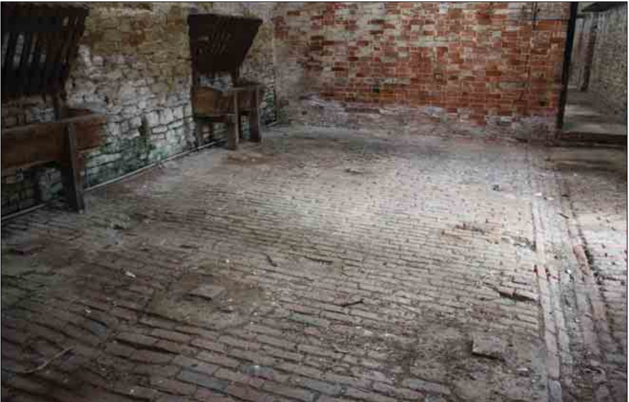
Plate 45: Brick floor, Building D (i)
