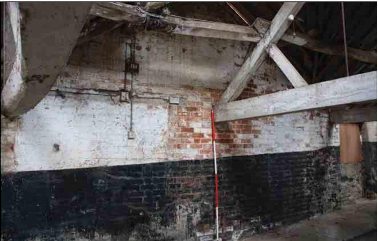
Plate 55: Blocked-up opening, Building D (iii)
