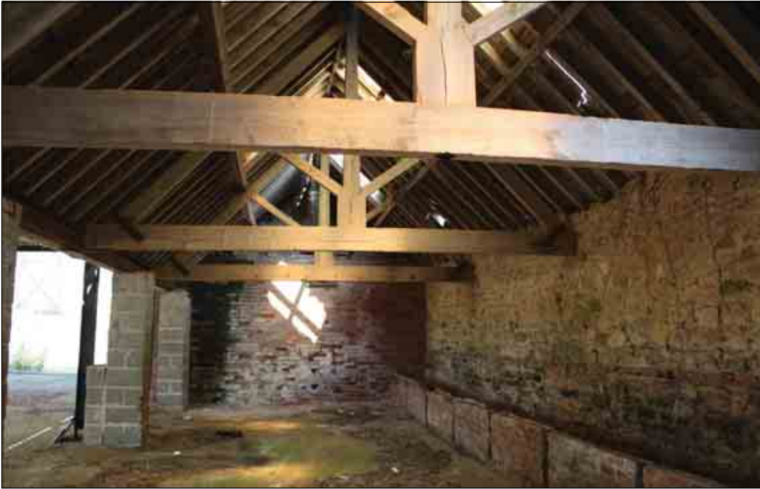
Plate 68: Interior view, Building E (ii)
