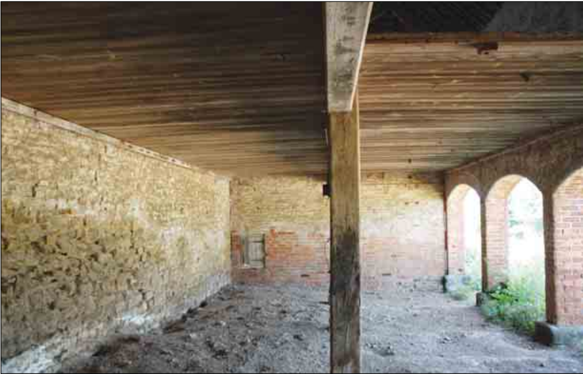
Plate 19: Interior view, Building B (ii)
