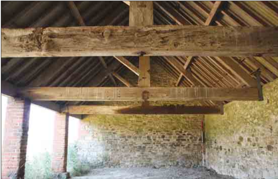
Plate 15: Interior view, Building B (i)
