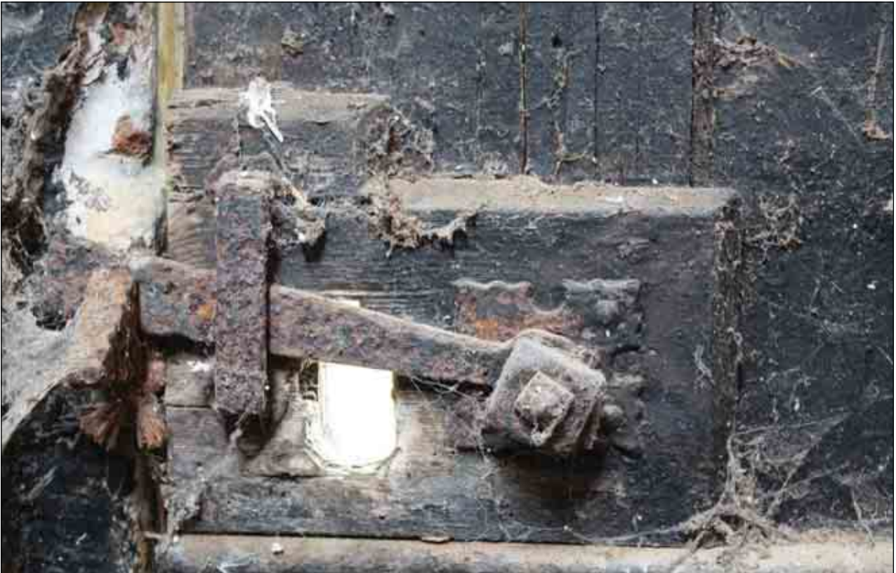
Plate 54: Detail of iron door latch, Building D (iii)
