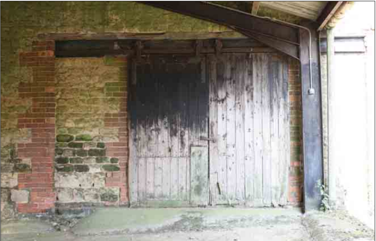
Plate 6: Loading doors, Building B, east-facing elevation
