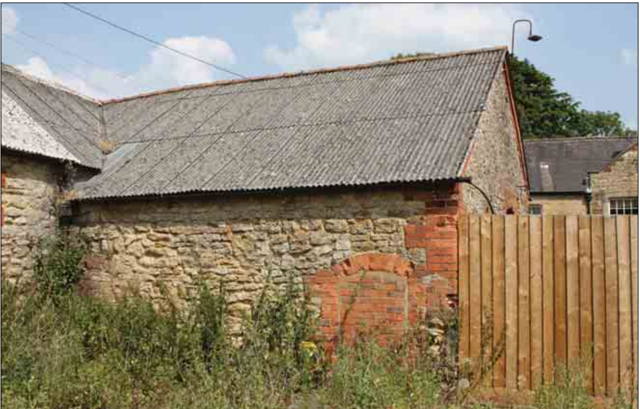
Plate 35: Building D, west-facing elevation (not part of survey)
