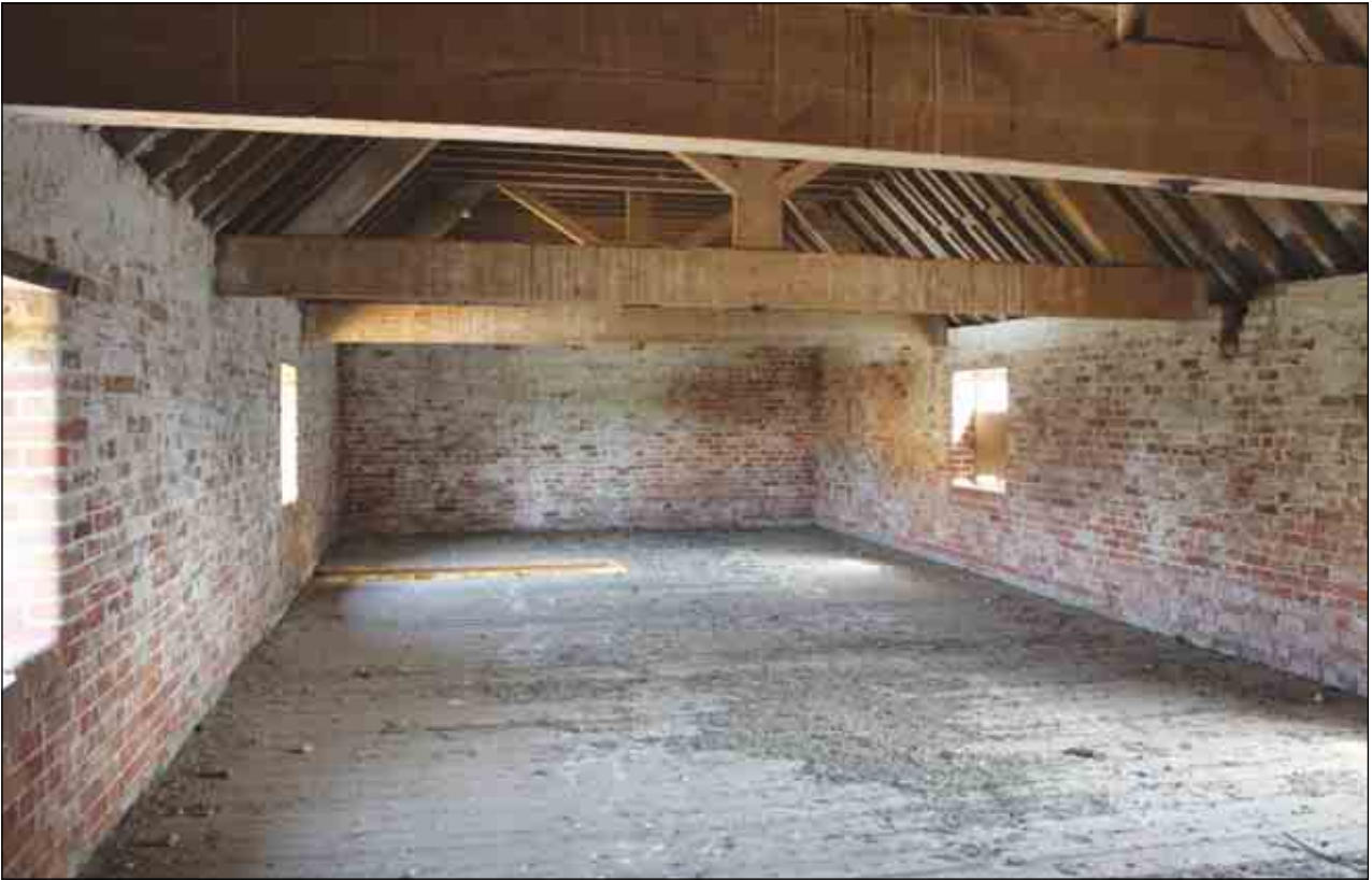
Plate 21: Interior view, first floor, Building B (ii)
