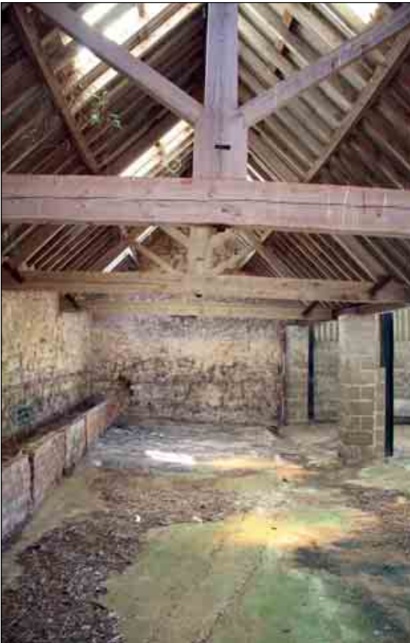
Plate 69: Interior view, Building E (ii)
