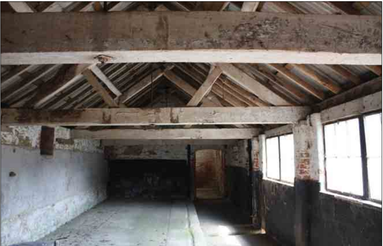
Plate 49: Interior view, Building D (ii)
