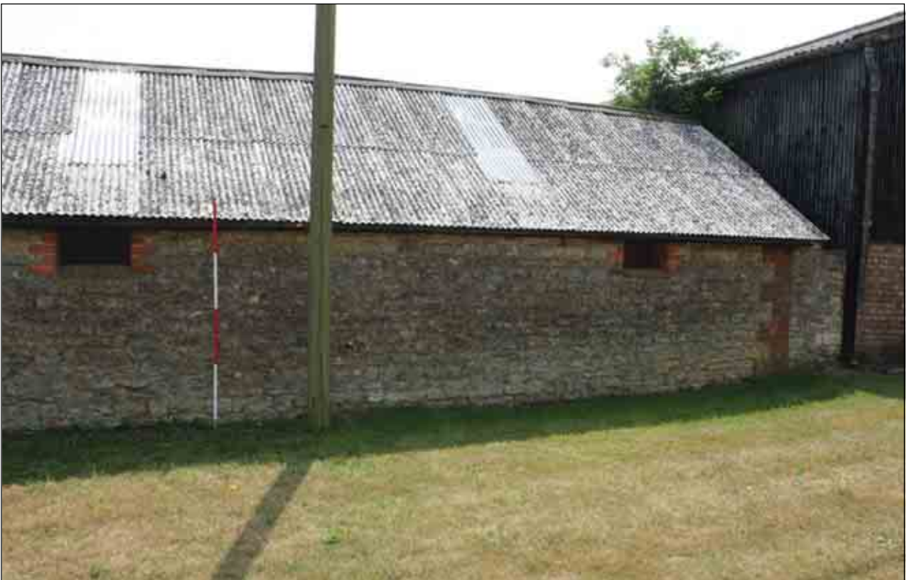
Plate 33: Building D, western end of north-facing elevation
