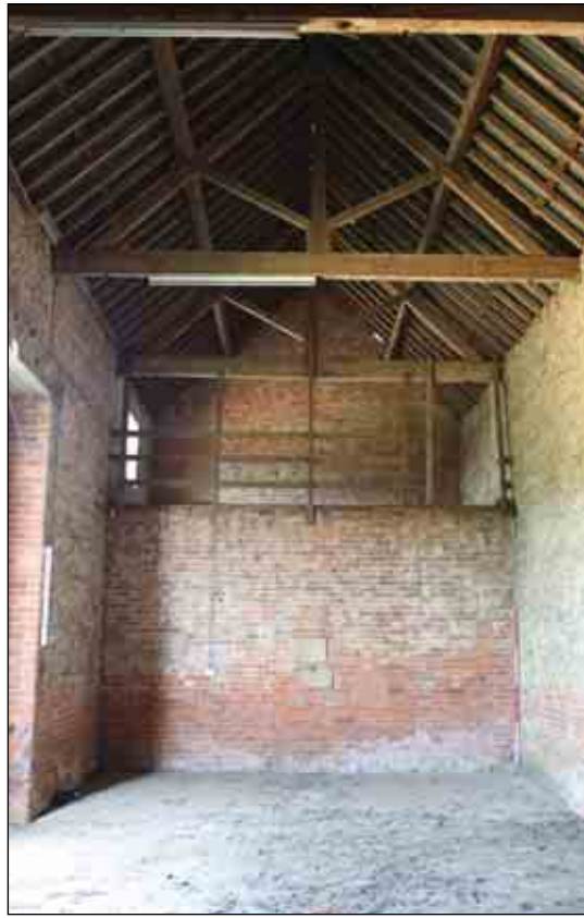
Plate 26: Interior view, Building B (iii)
