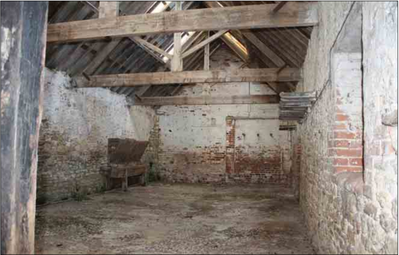
Plate 48: Interior view, Building D (i), northern end
