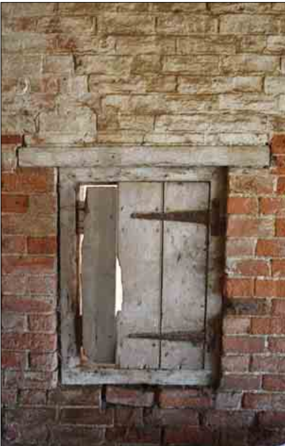
Plate 20: Detail of small doorway/hatch, Building B (ii)
