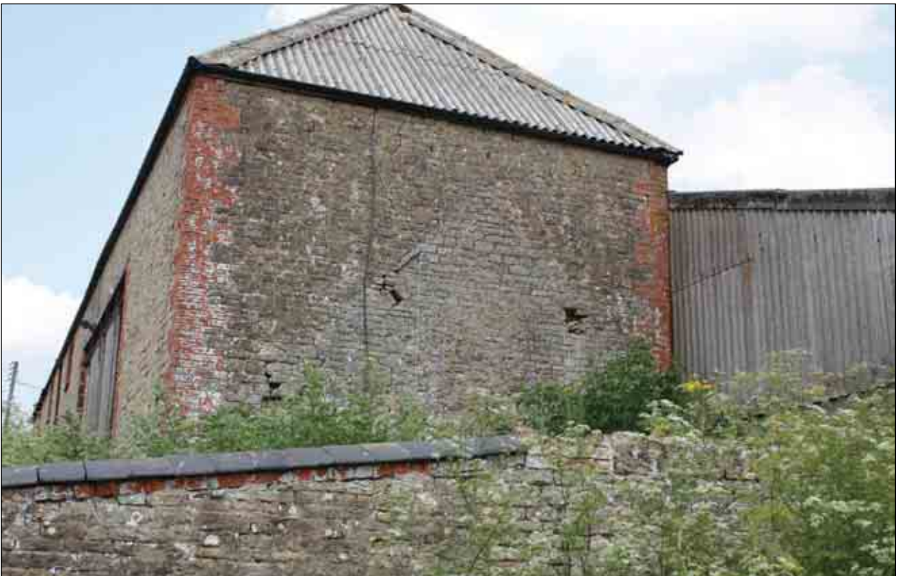
Plate 10: Building B, south-facing elevation
