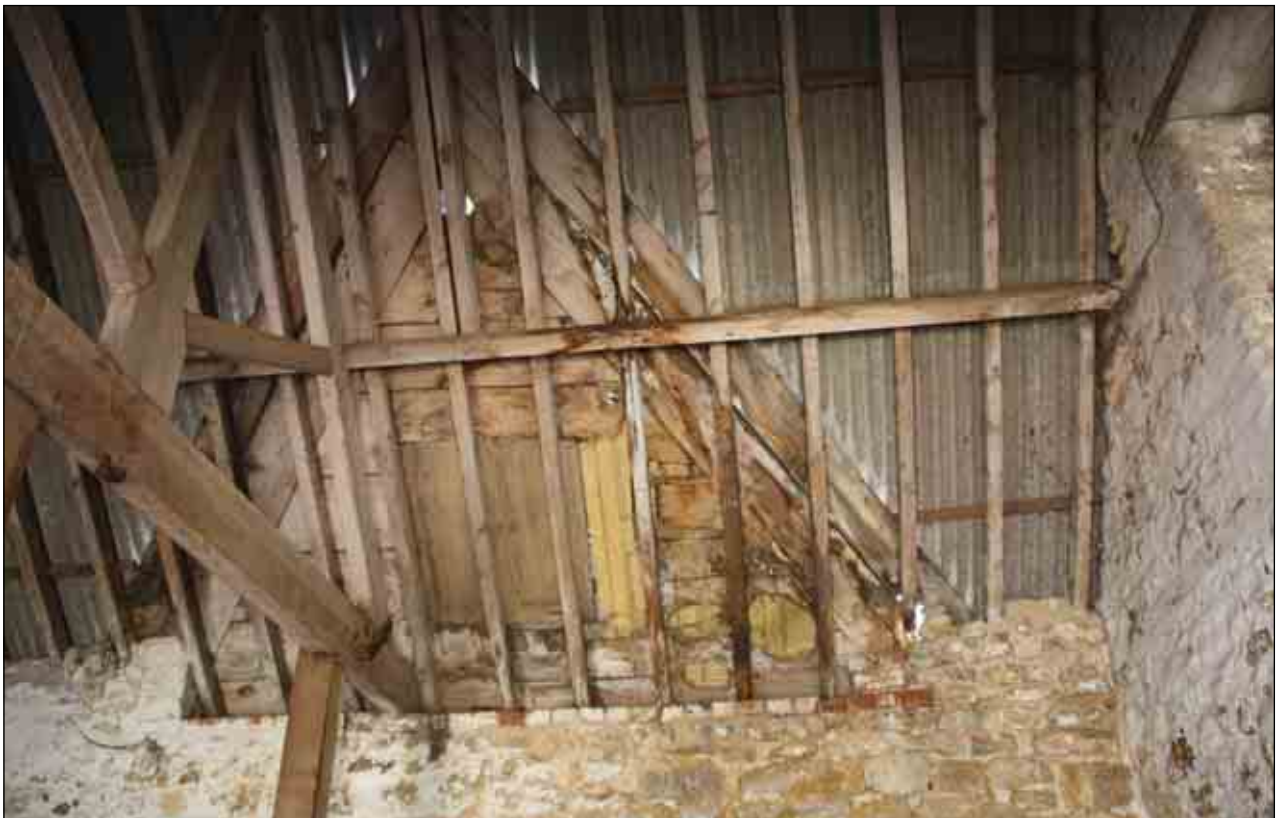
Plate 65: Detail of roof, Building E (i)
