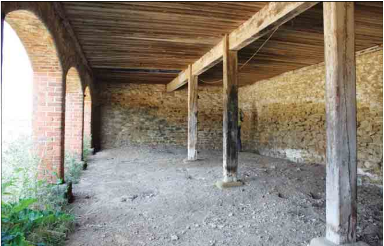
Plate 17: Interior view, Building B (ii)
