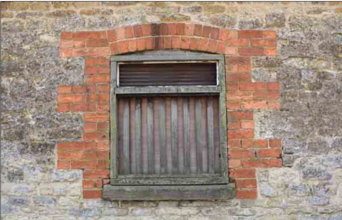
Plate 61: Building E, ventilation opening on north-facing elevation
