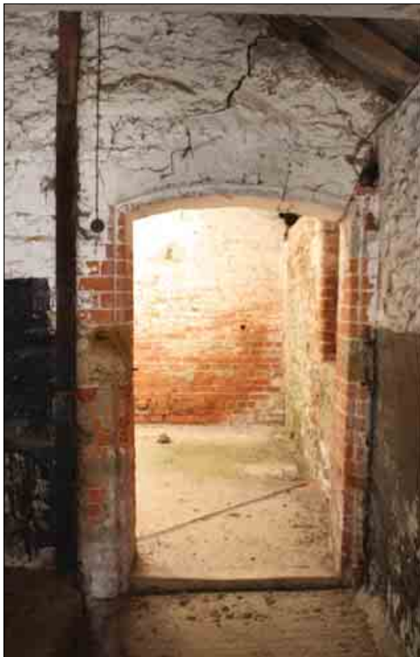
Plate 51: Internal doorway with recessed brick surround, Building D (ii)
