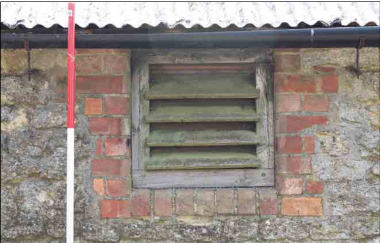
Plate 31: Detail of ventilation opening on Building D, north-facing elevation
