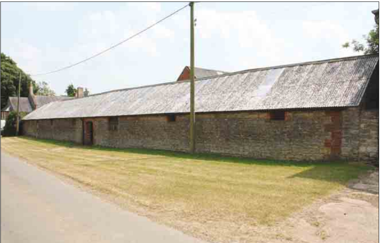
Plate 29: Building D, north-facing elevation
