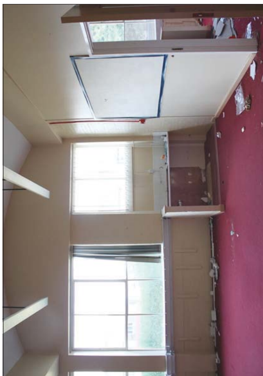
Plate 69: Location of former doorway with a later inserted window and sink (122)
