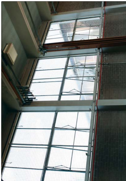
Plate 36: Windows on eastern elevation of boys gym (06)
