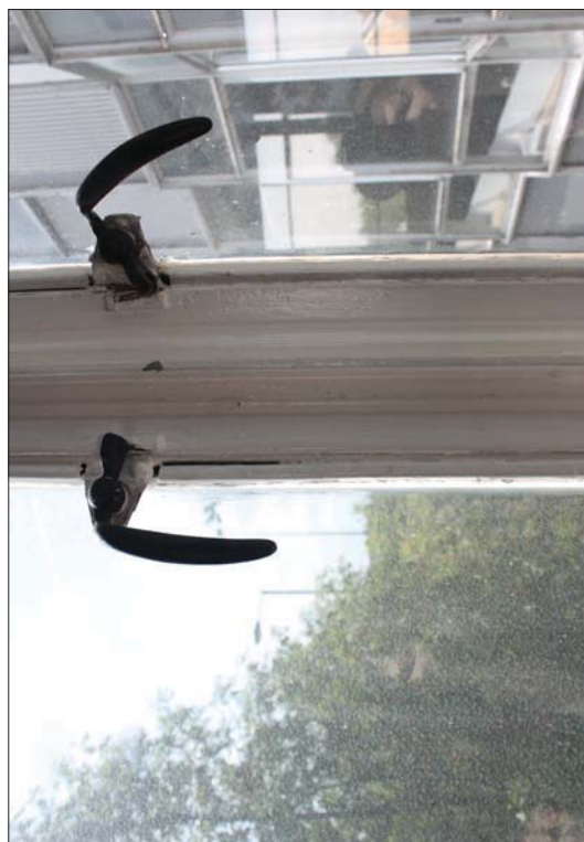
Plate 75: Detail of drop handles
