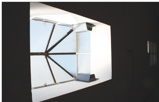
Plate 45: Raised skylight above library reception area (68)
