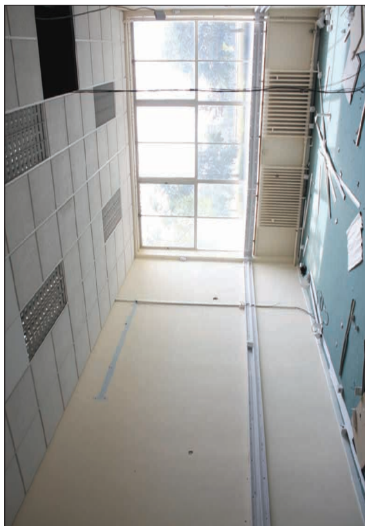
Plate 56: General view of conference room (84)
