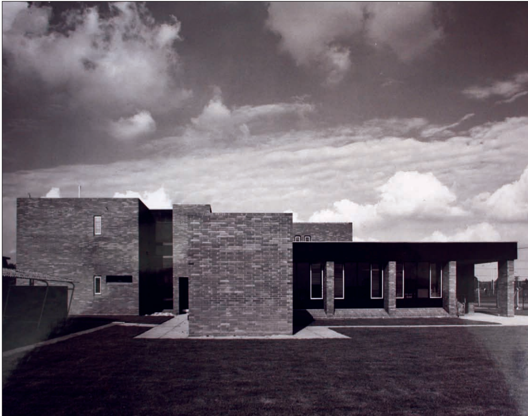
Figure 19a: Photograph of the Ward's Bridge "RSLA", 1986 (WAVE Ref. P/2523)
