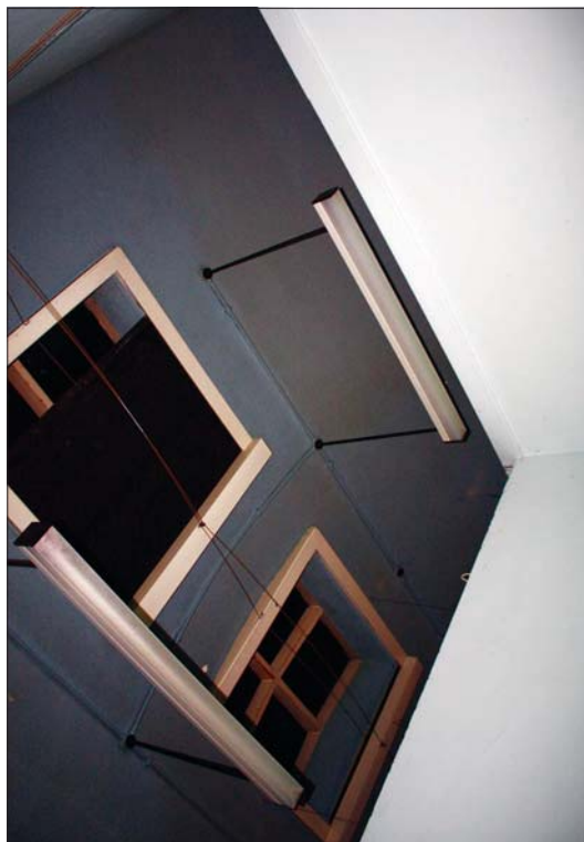
Plate 68: Original ceiling above inserted partition walls in store room (120)
