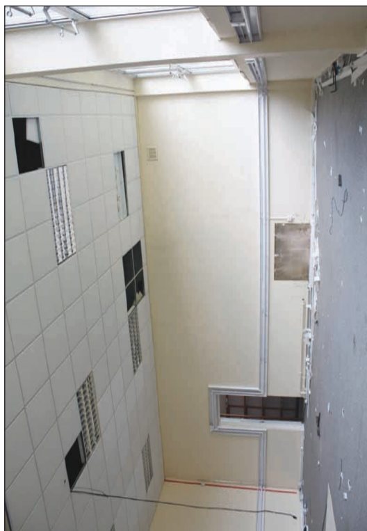
Plate 55: General view of conference room (82)
