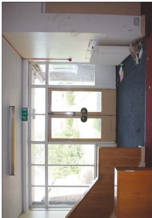
Plate 44: Detail of entrance doors on north-facing elevation from within library reception area (68)
