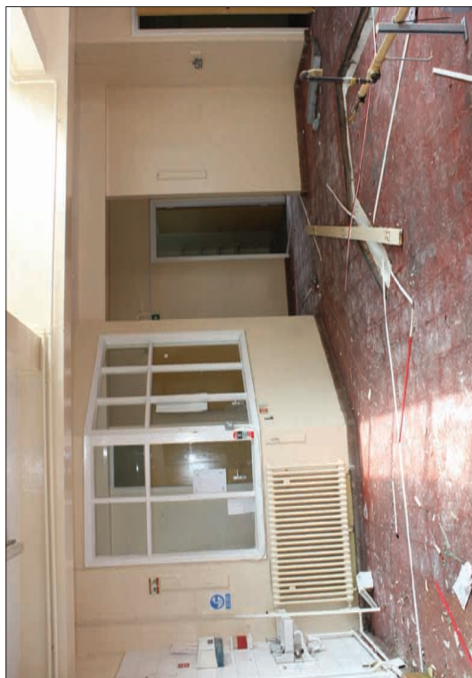
Plate 40: Office within kitchen area (43)
