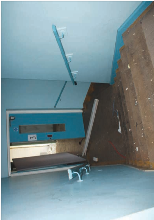
Plate 81: Central staircase, Tower 2, second floor (171)
