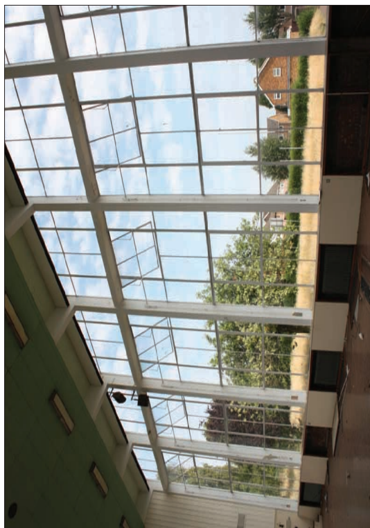
Plate 26: Windows on northern elevation of hall (28)
