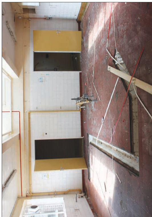
Plate 38: General room view of kitchen (43)
