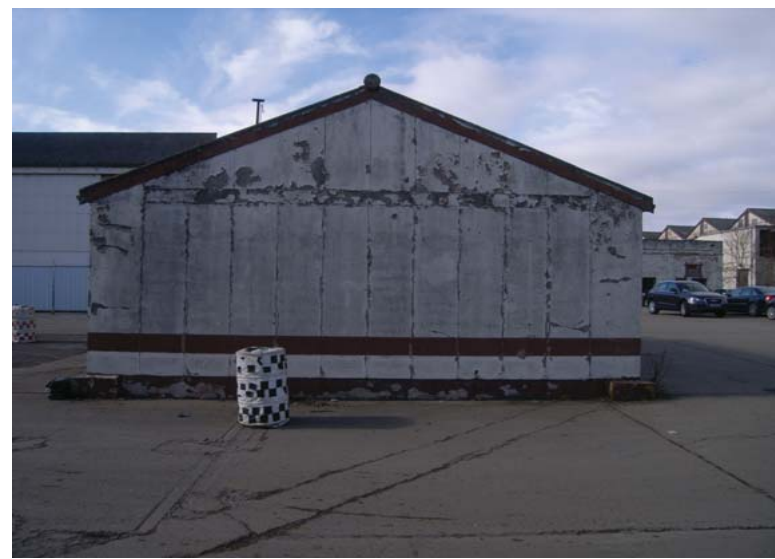
Plate 4: Building 81 East Elevation
