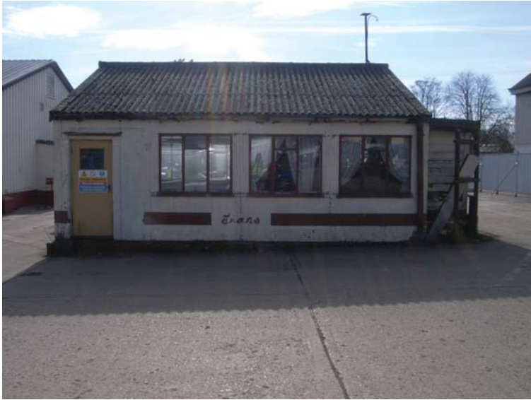
Plate 1: Building 81 North Elevation
