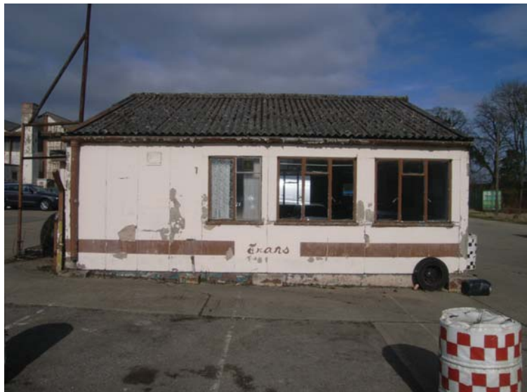
Plate 3: Building 81 South Elevation
