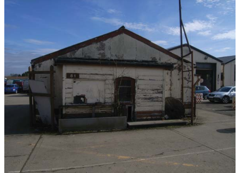
Plate 2: Building 81 West Elevation
