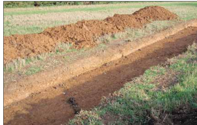
Plate 4: Trench 4 from south-west showing slag-filled drain
