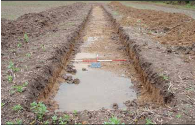
Plate 45: Trench 45 from north
