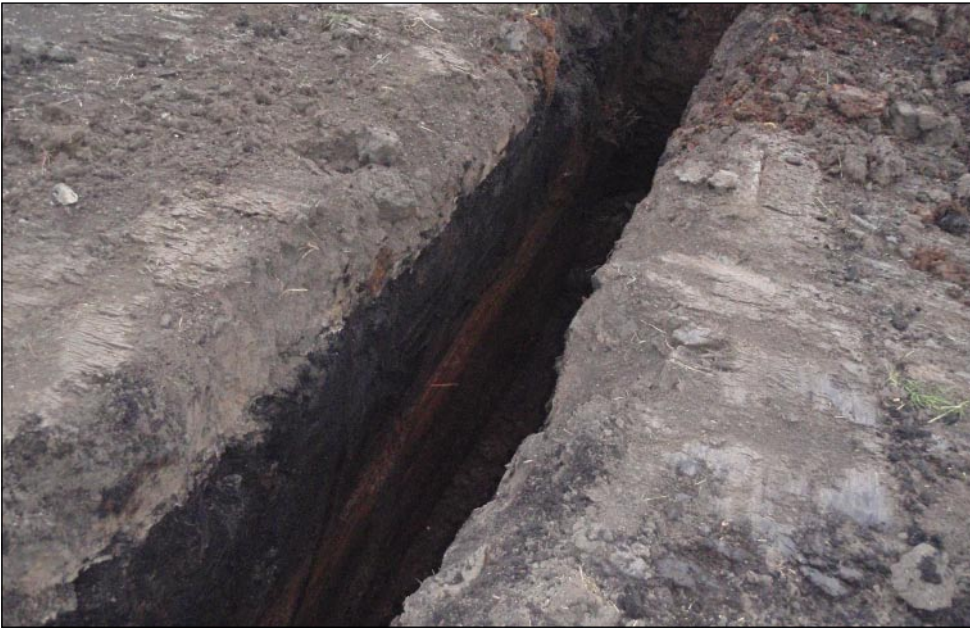
Plate 7: Pond A 'key trench'
