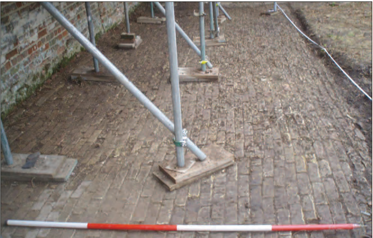
Plate 6: Brick courtyard surface 70 (Area 1) after cleaning, viewed from south-east
