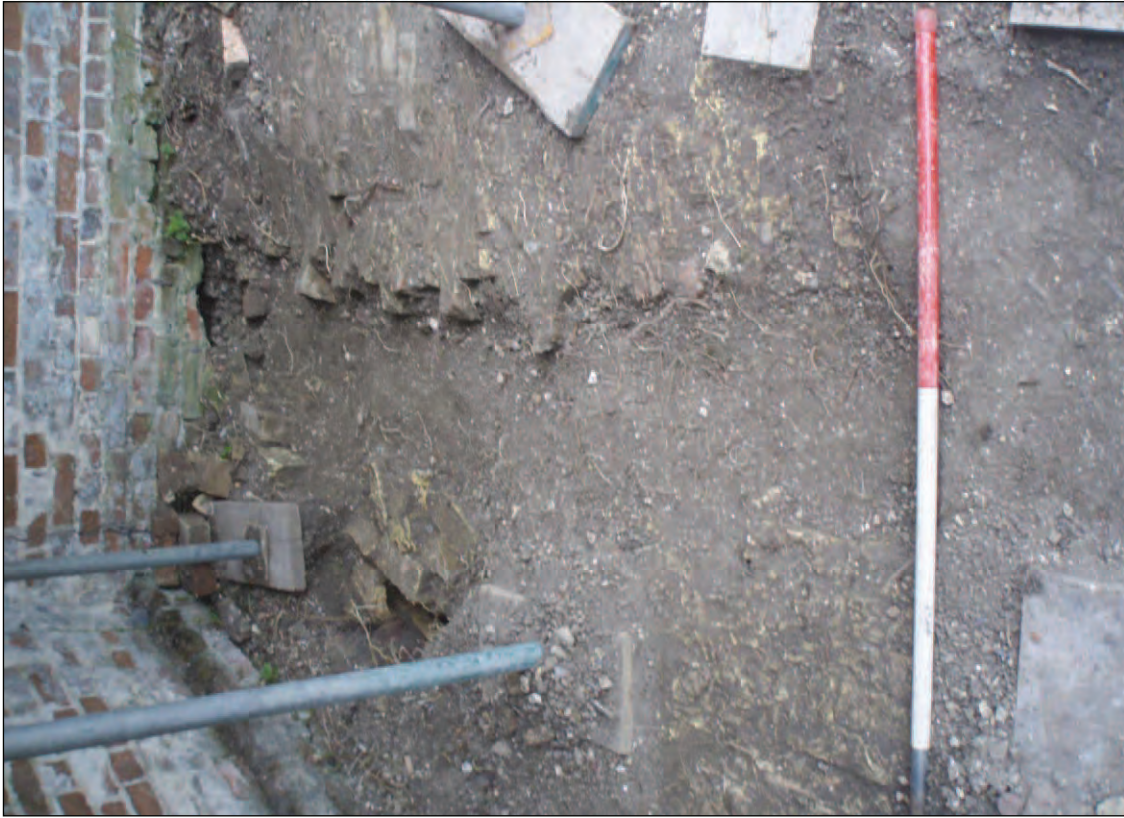
Plate 8: Drain 81 cutting surface 80 and discharging beneath wall, north-east side of north-west tower (Area 1)
