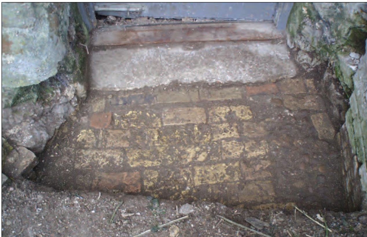
Plate 28: Detail of brick floor 34 adjacent to basement door to south tower (Area 4), viewed from north
