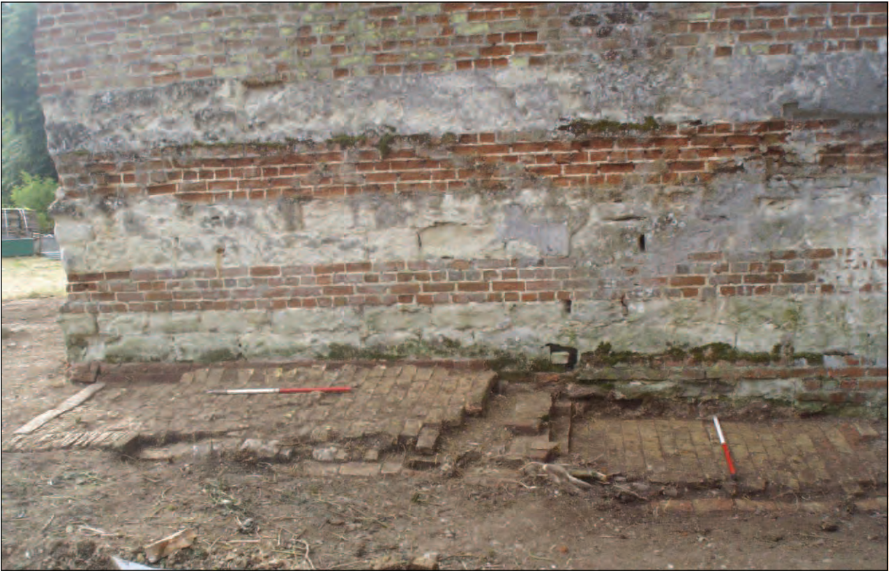
Plate 26: View of south-east Folly wall showing evidence of former stairs (Area 3/4), viewed from north-west
