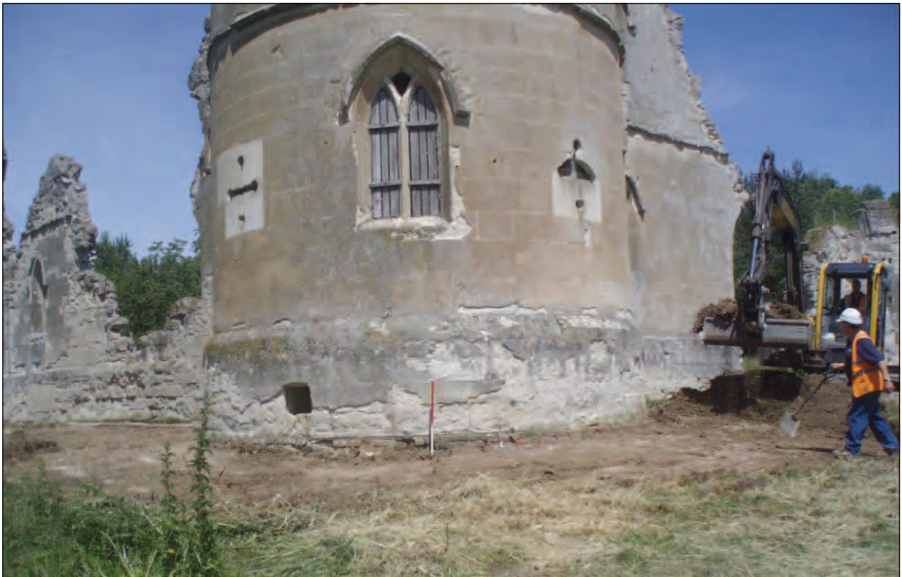
Plate 1: General shot of vegetation stripping by machine around base of the Folly
