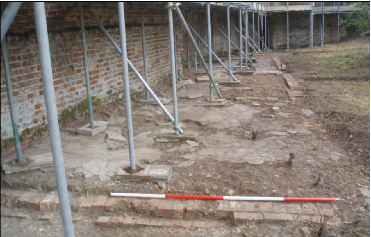
Plate 10: Area of building foundations (Rooms 1, 2, 3 and 4; Area 1) after cleaning, viewed from south-east
