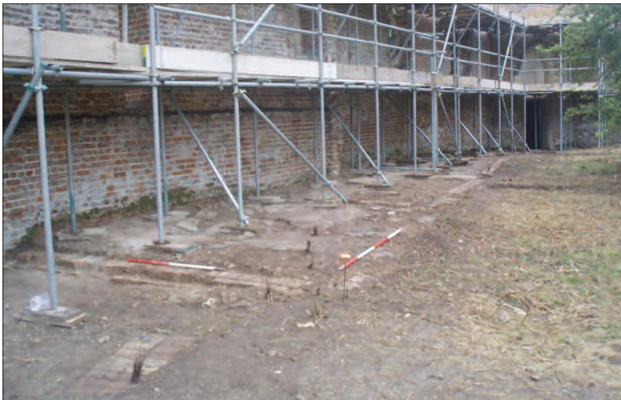
Plate 18: Detail of partially exposed brick path 72 (in foreground; Area 2), viewed from north
