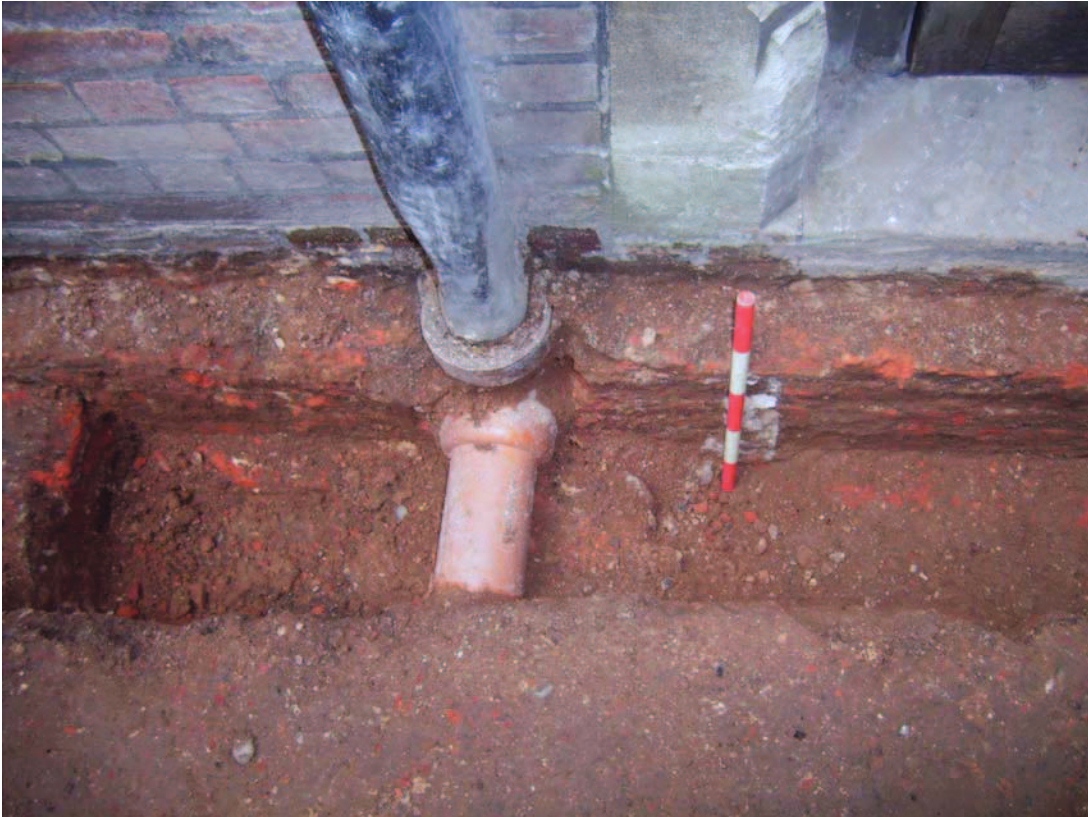
Plate 4: East - brick footing and ceramic pipe
