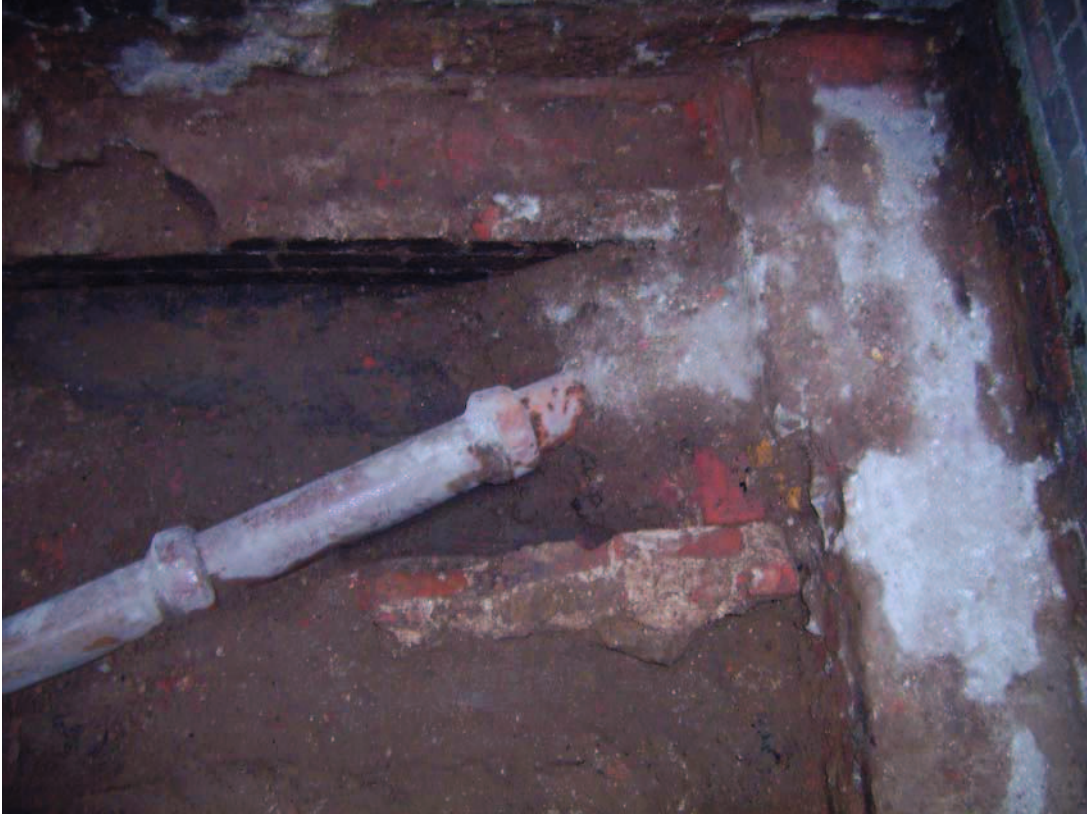
Plate 7: South east corner of excavation
