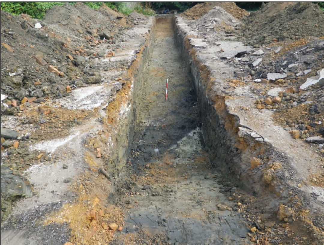
Plate 4: General shot of Trench 4, showing modern channel
