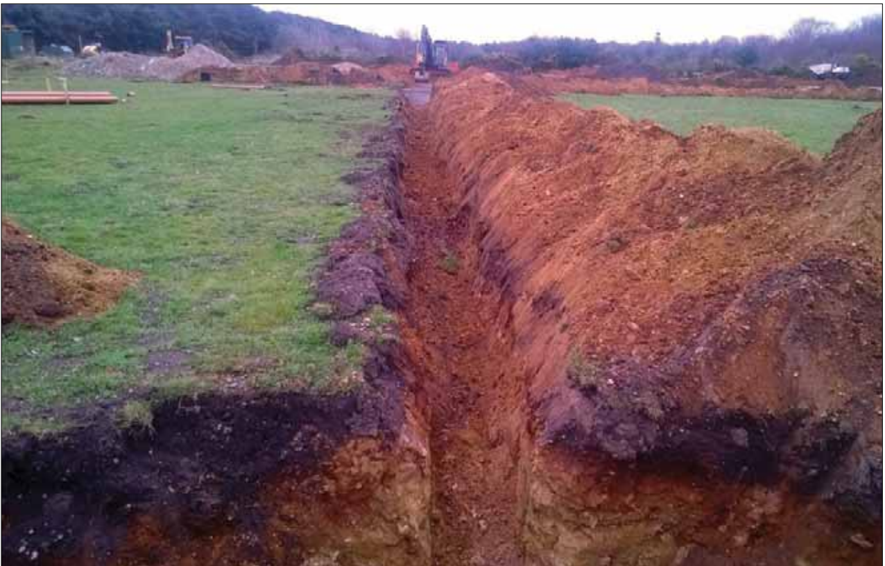
Plate 2: Service trench under excavation showing impact depth
