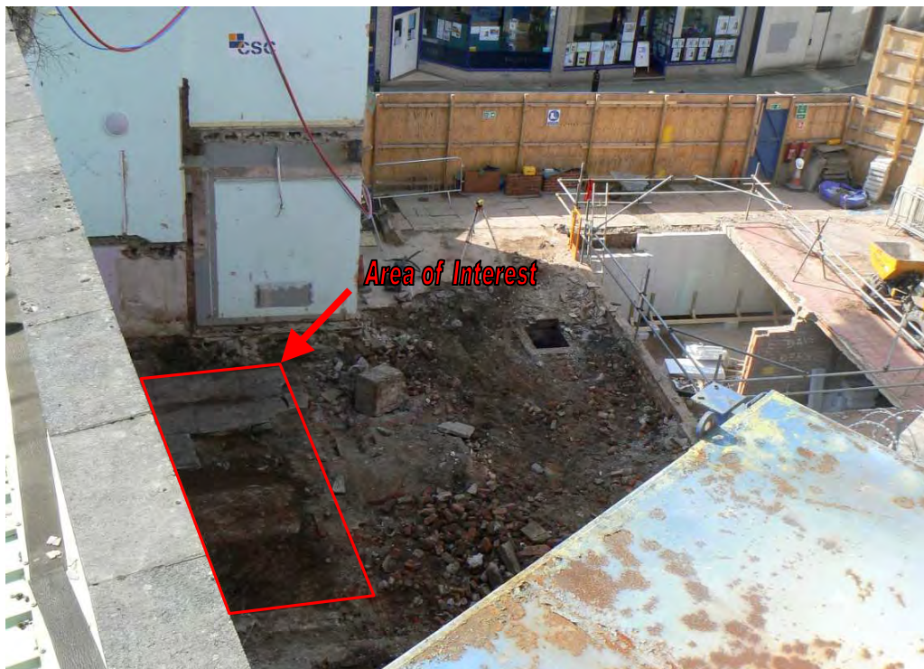
Figure 1: View across the development site, marking the location of the excavation area
