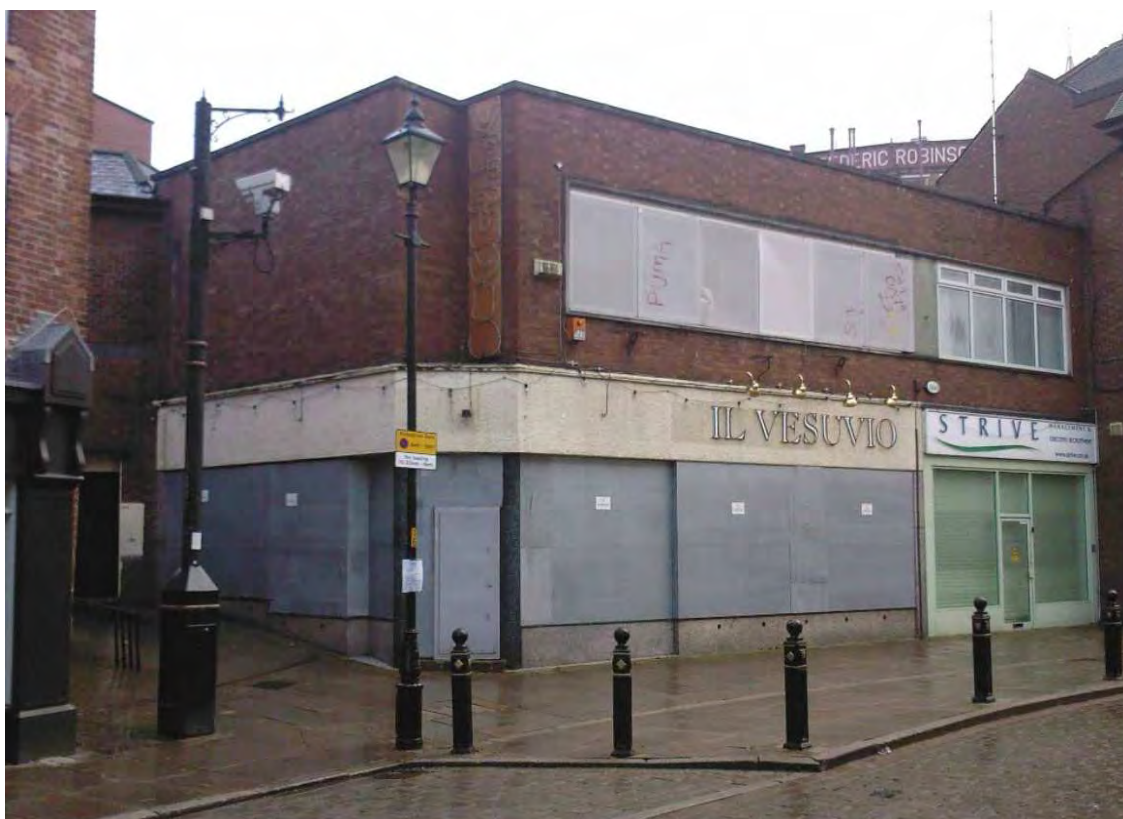
Plate 12: Recent view of 7-9 Lower Hillgate prior to demolition in 2011
