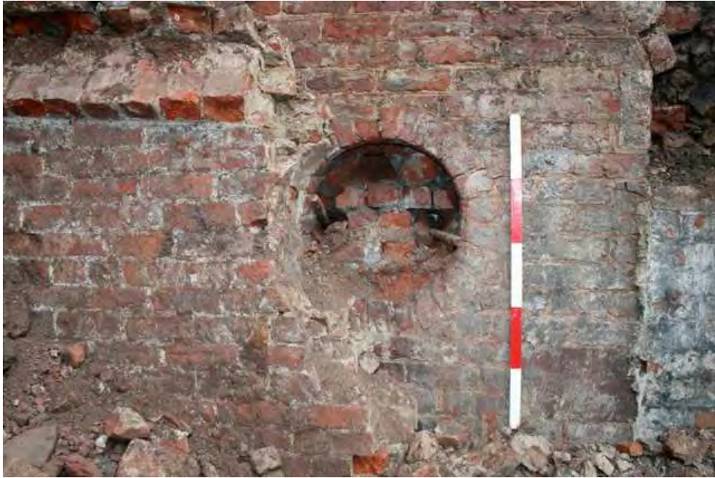
Plate 38: 'Oeil de boeuf' aperture behind later vault wall, with arched door jamb to right, including sandstone pad near exposed base
