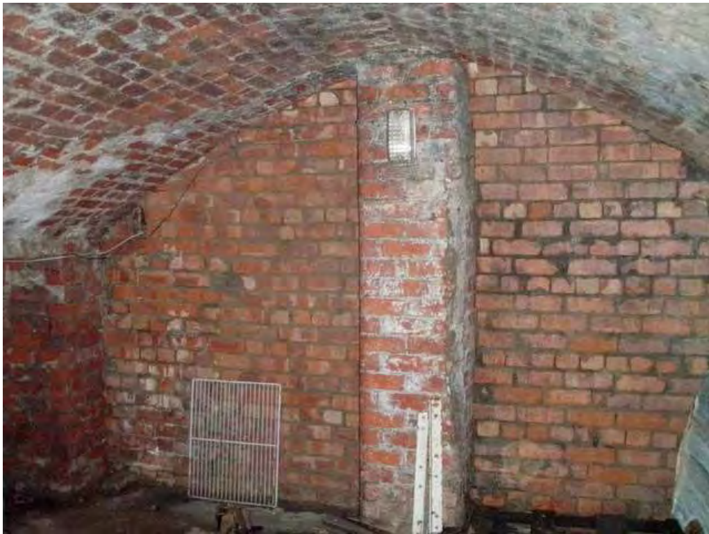
Plate 37: Inserted brick pillar, blocking walls and rebuilt vaulting at west end of undercroft
