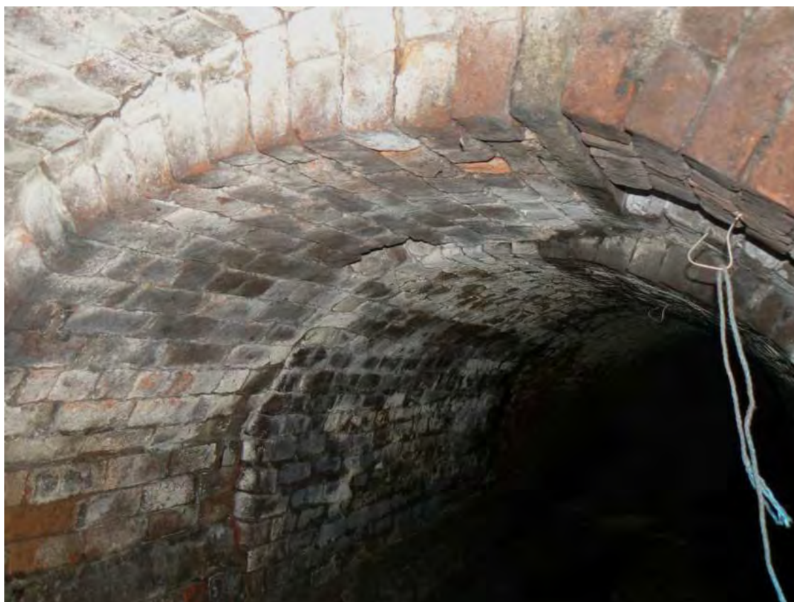
Plate 20: View of the interior of Culvert 106
