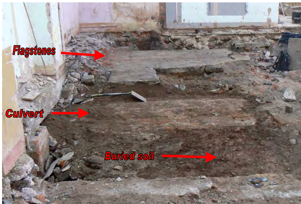
Figure 2: View across the proposed excavation area
