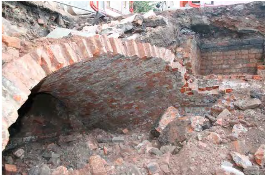
Plate 33: Sloping vault of undercroft observed during groundworks
