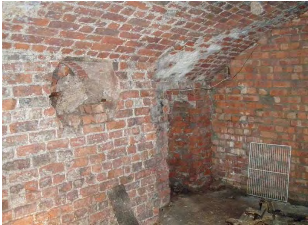
Plate 32: Hand-made brick construction of vaulting, with blocking wall and inserted entrance
