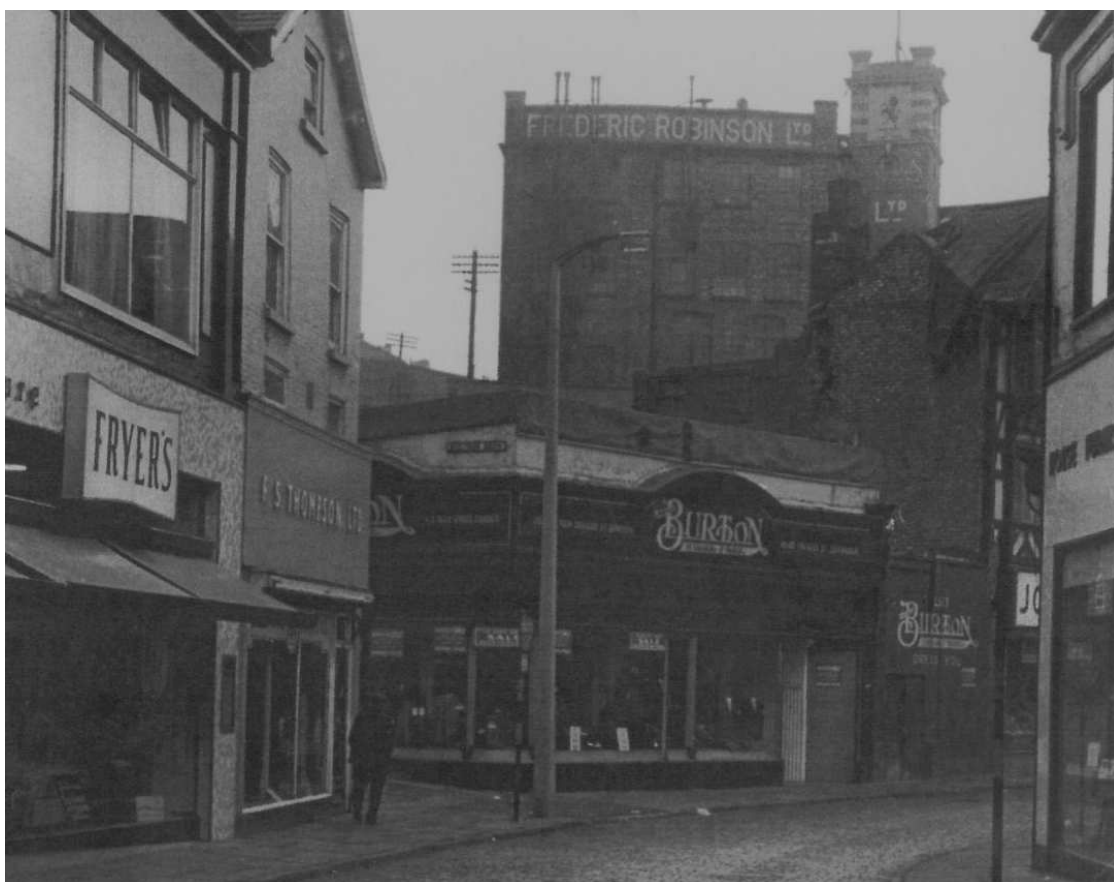
Plate 11: 7-9 Lower Hillgate in 1963, showing the upper floors of the building removed
