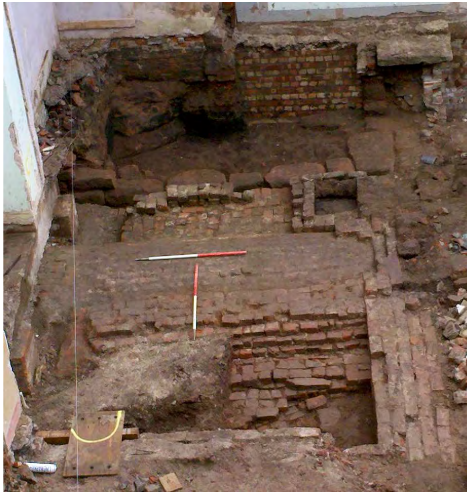
Plate 14: Post-excavation overview of the excavation area, facing west.
