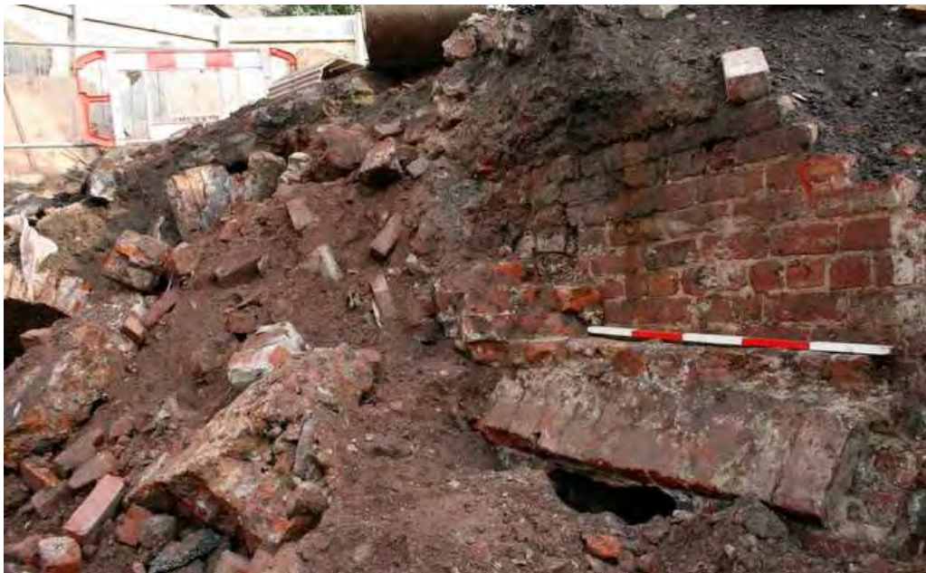
Plate 39: Earlier wall extending above undercroft vaulting, with brick infill between
