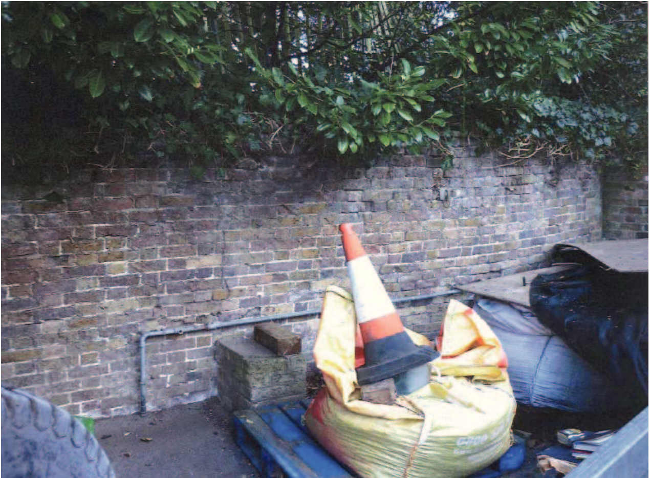
Plate 1: Wall before dismantling (Photo: Emma Simpson, SBC Ltd)
