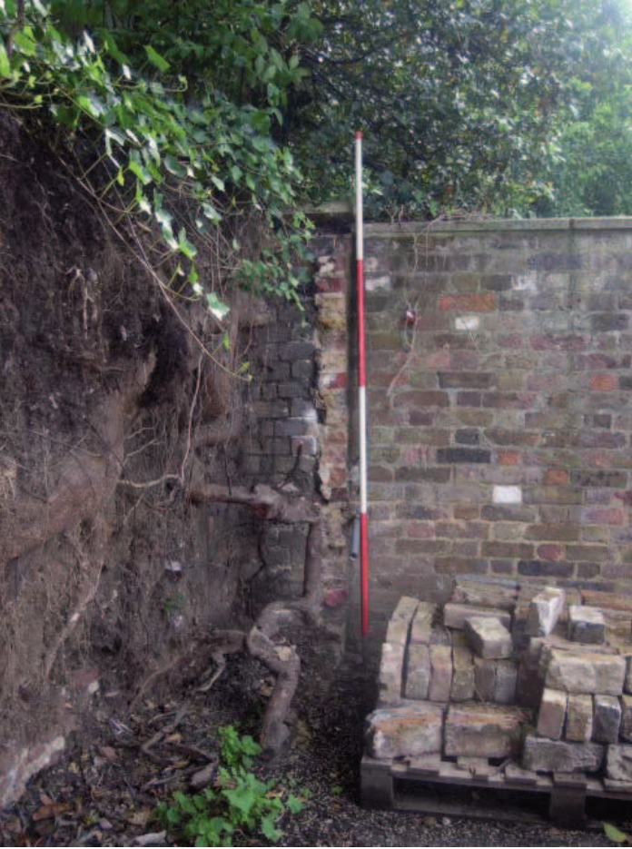
Plate 5: Detail of wall eastern brickwork following dismantling
