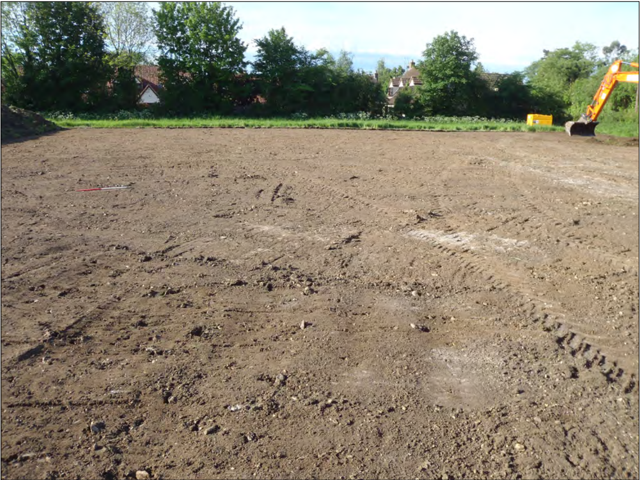
Plate 7: Town Green: Compound topsoil strip looking South
