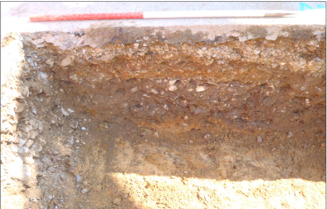
Plate 4: Church Street: Drill pit 13 showing layer (5) looking North East
