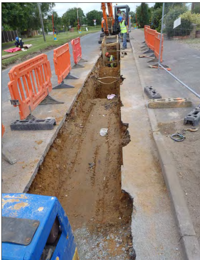
Plate 2: Chequers lane: Open cut 5 looking North
