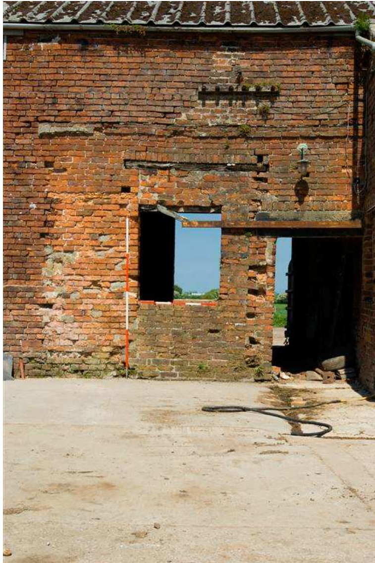
Plate 9: The remodelled door in the south elevation
