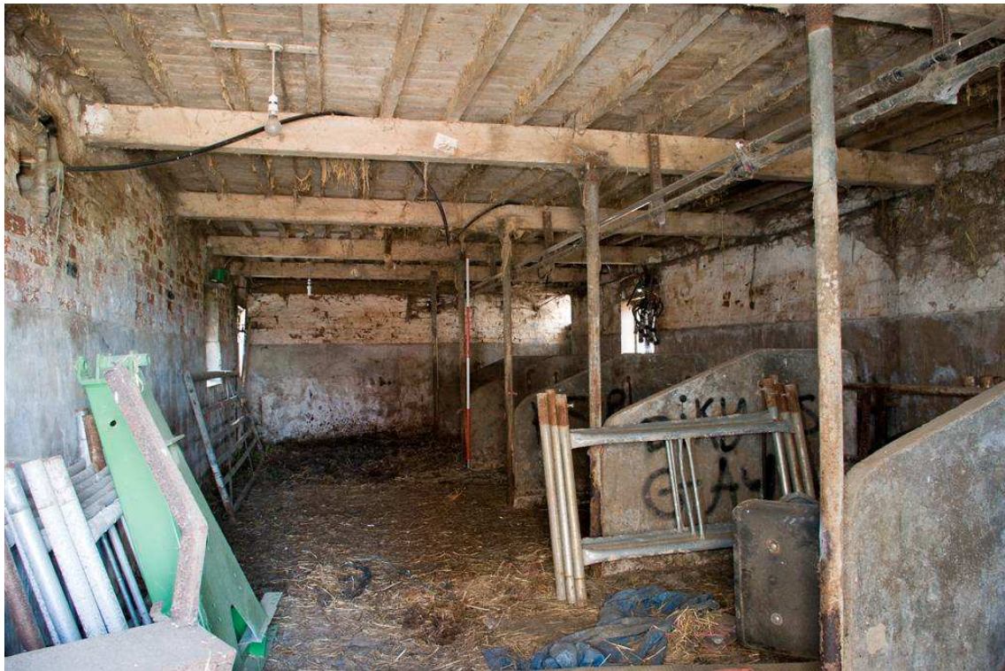
Plate 12: General view of the shippon, facing south
