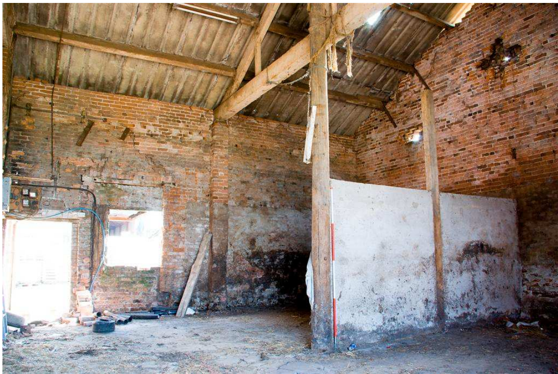
Plate 4: Internal view of the west side of the barn
