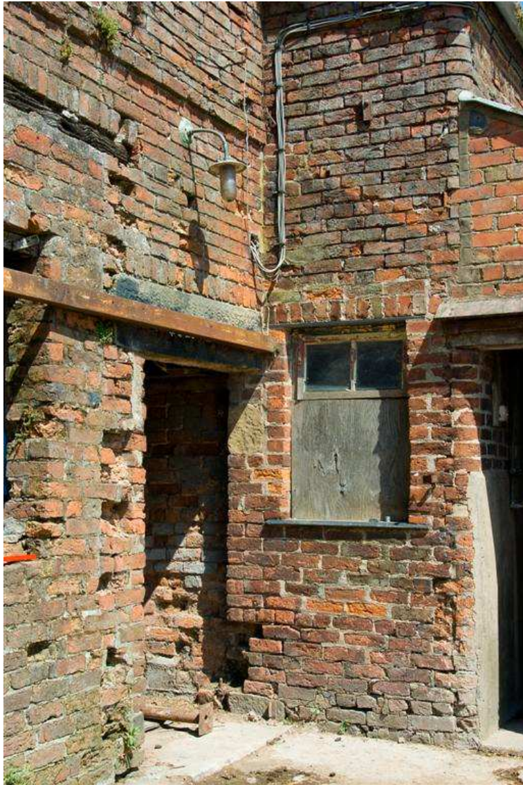
Plate 10: Evidence of the porch on the south side of the barn and join of the outshut
