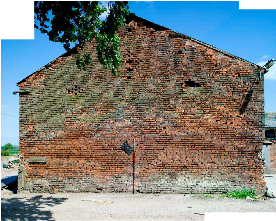
Plate 11: Digitally stitched image of the west elevation, showing cruciform ventilation in the centre
