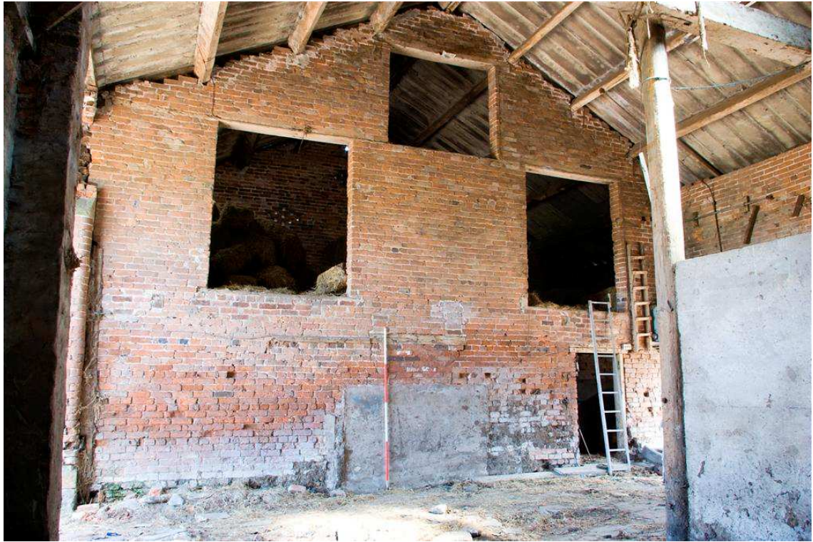
Plate 5: Brick cross wall in the barn
