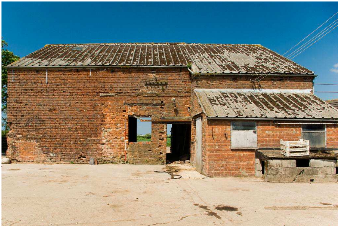
Plate 8: The south elevation of the barn
