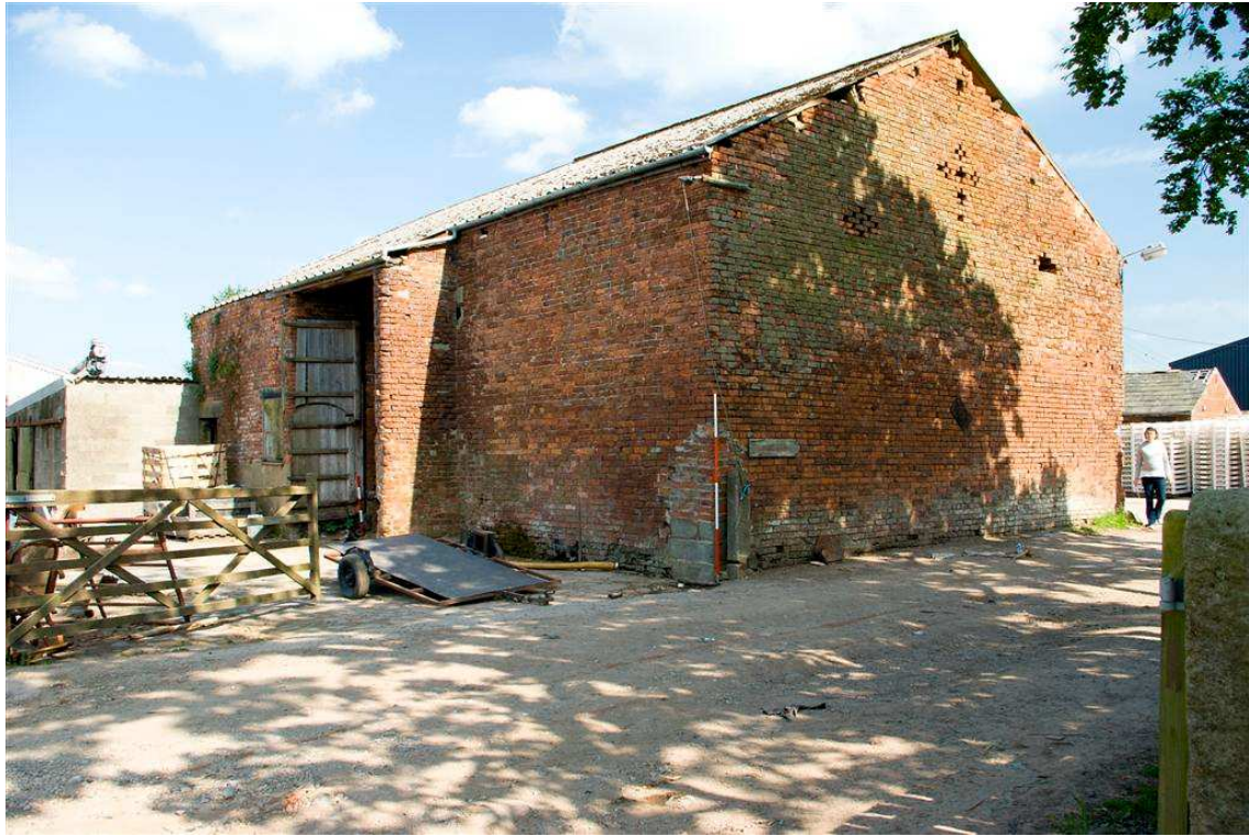
Plate 1: The barn at Hankinson's Farm, from the north-west
