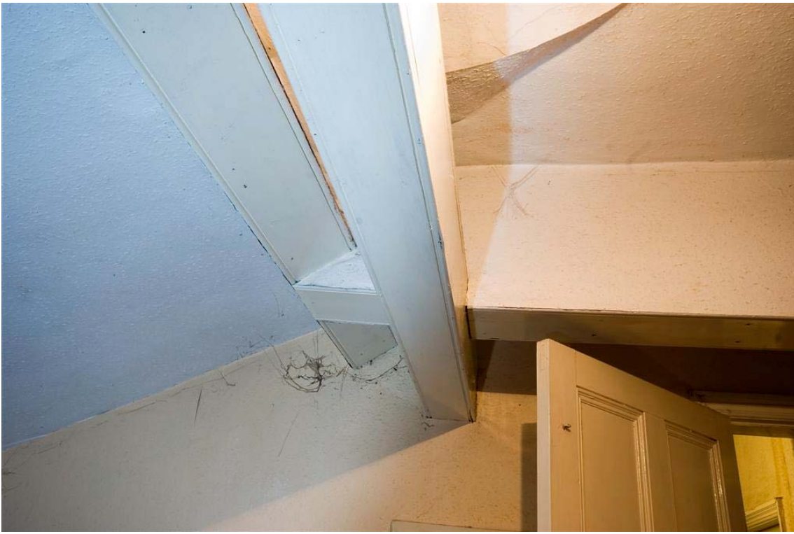
Plate 19: The exposed roof timbers in the bathroom comprise the wall beam and a purlin. The purlin is supported by the boxed tie-beam.
