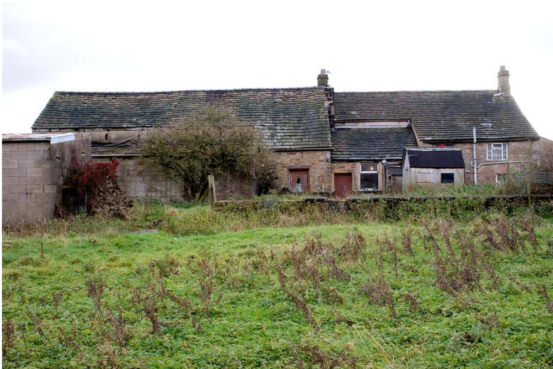
Plate 8: The rear (north) elevation of the building. This illustrates the projections from both the farmhouse and barn, and the kitchen extension to the back of the farmhouse.
