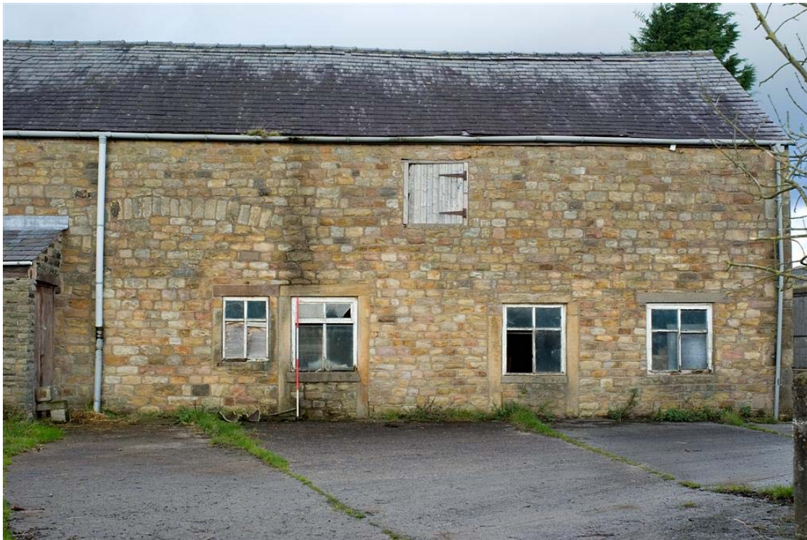
Plate 4: The principal (south) elevation of the barn. The conversion of doorways into windows can be clearly seen. The down-pipe obscures a joint in the masonry, suggesting the extent of the original wagon door.
