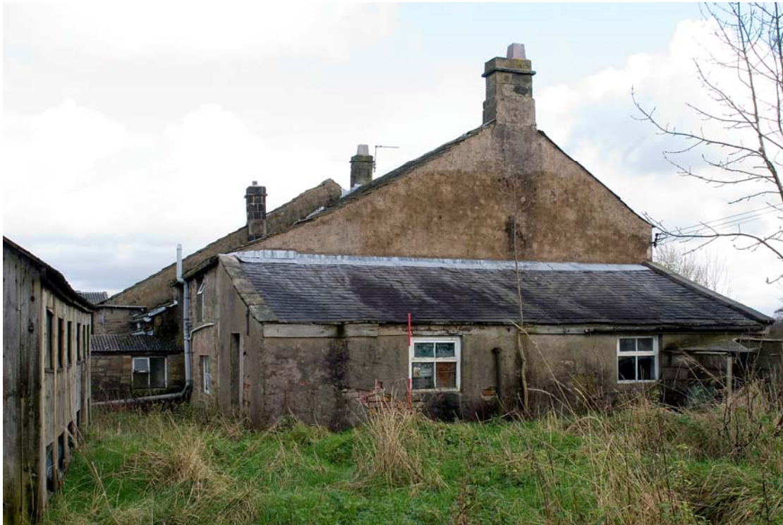
Plate 6: The west gable of the farmhouse with modern extension attached. The difference in the slope of the roof pitches between the farmhouse and barn is evident.
