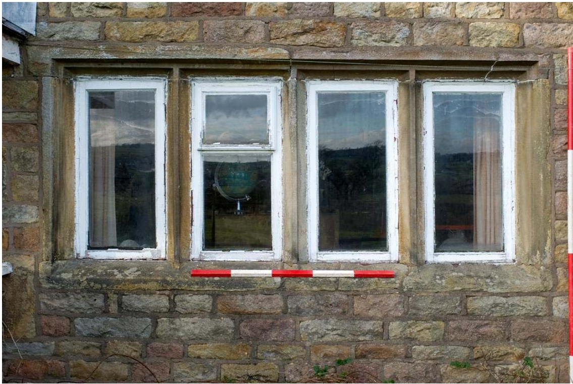
Plate 5: Extant mullion window at ground floor in the front elevation of the farmhouse. The larger of two mullion windows in the elevation, this provided light for the living room.
