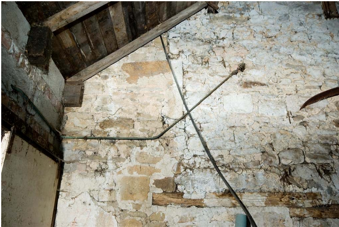
Plate 25: Vertical scar in the west wall of the barn store. This represents the original line of the back wall of the farmhouse.
