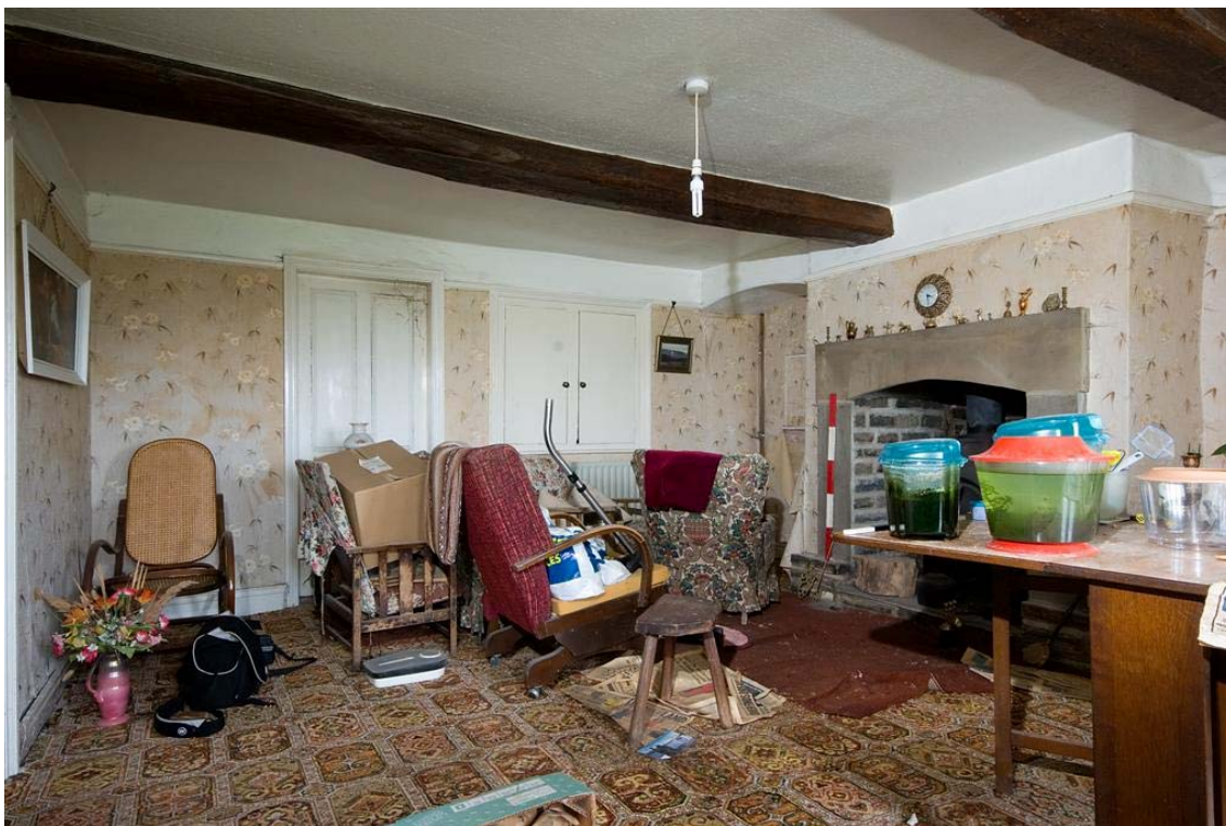
Plate 14: General view of the living room. Two exposed joists are visible below the ceiling, the joist towards the back of the room extends into the chimney-breast. The spice cupboard can be seen between the fireplace and the back wall. The cupboard in the back wall conceals a mullion window.
