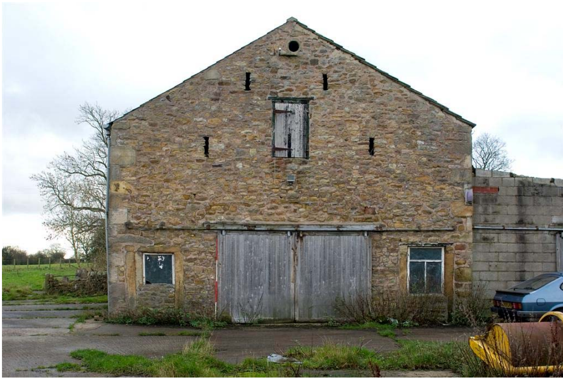
Plate 7: The gable end (east elevation) of the barn. The large doorway is not original. The windows were previously doorways.
