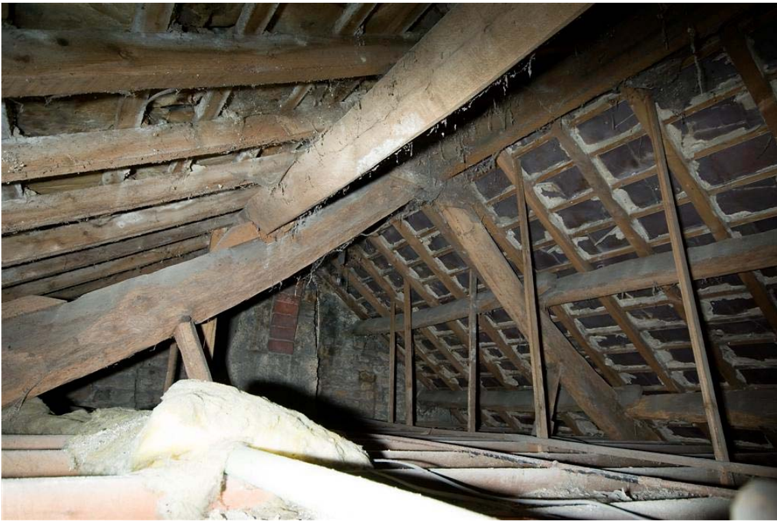
Plate 22: View of the roof space above the farmhouse. The original socket within the principal rafter, for what was a trenched purlin, is visible beneath the current position of the purlin.
