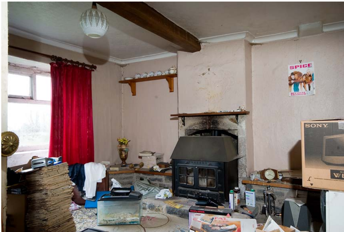
Plate 16: This shows the general arrangement of the parlour. The window is a modern insert, the exposed joist extends into the chimney-breast and the small protrusion to the right of the fireplace, at ceiling height, is possibly a corbel.
