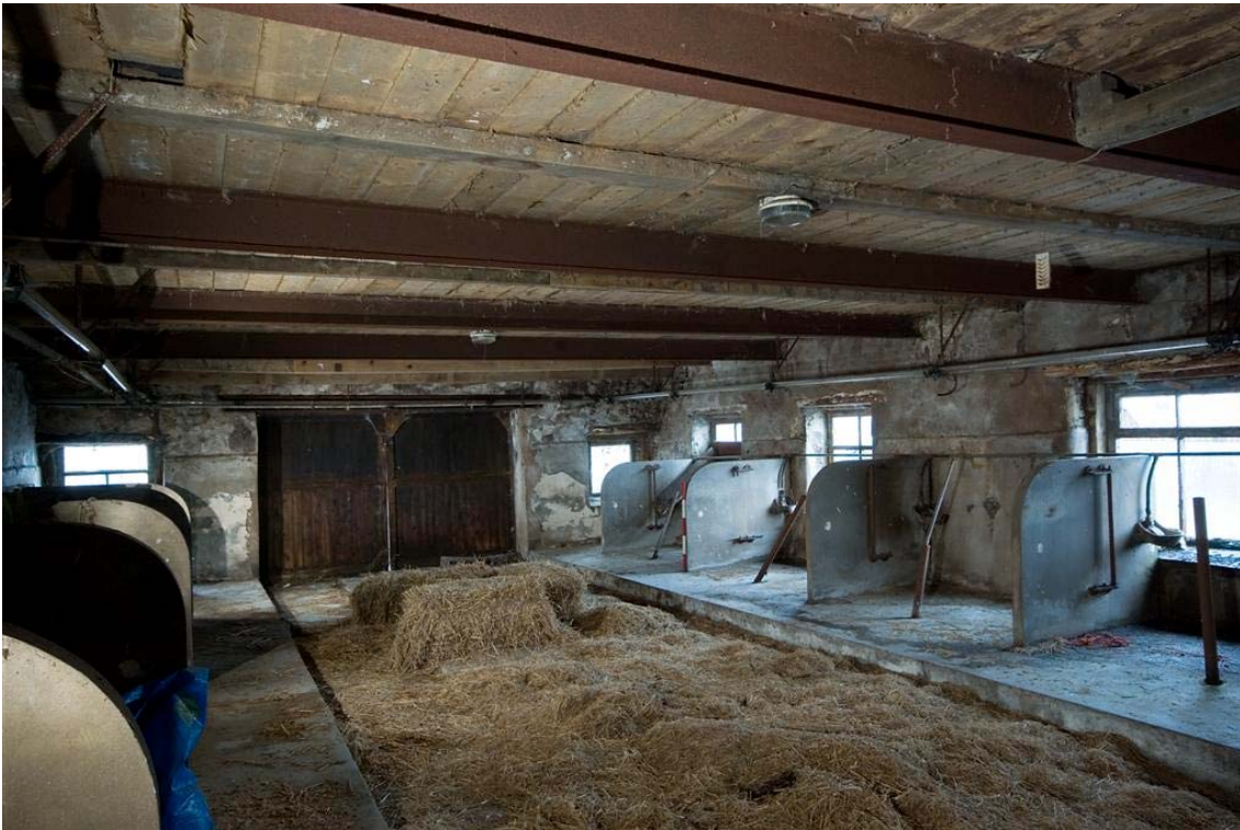
Plate 23: General view of former shippon, facing east. The stall, doorway and RSJ joists are all modern additions.
