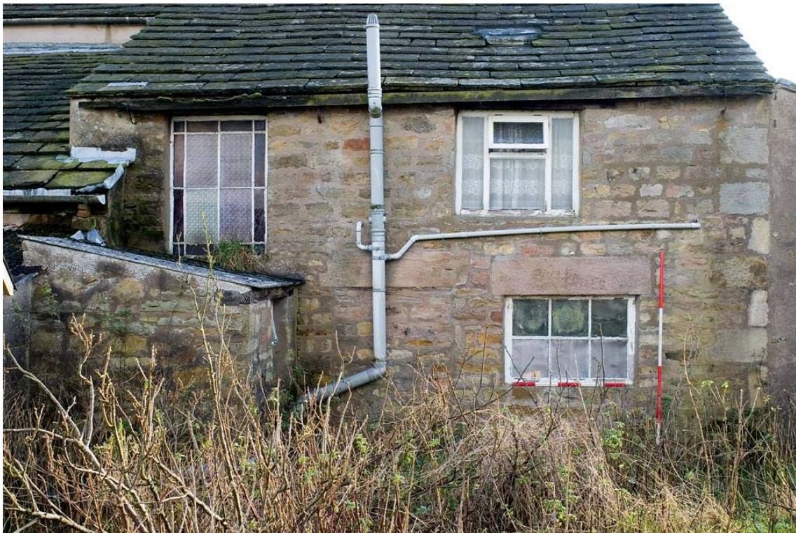
Plate 10: Window arrangements in the rear (north) elevation of the farmhouse. As in the front elevation, the upper window is taller than that at ground floor. A blocked doorway can also be seen behind the down-pipe.
