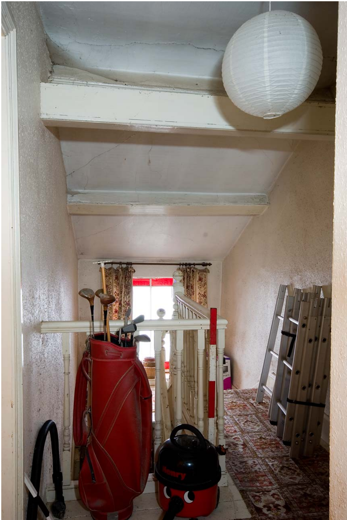
Plate 21: Wall beam and purlin exposed above the stairway. The wall beam indicates the position of the original wall of the farmhouse. The purlin relates to the construction of the rear projection.
