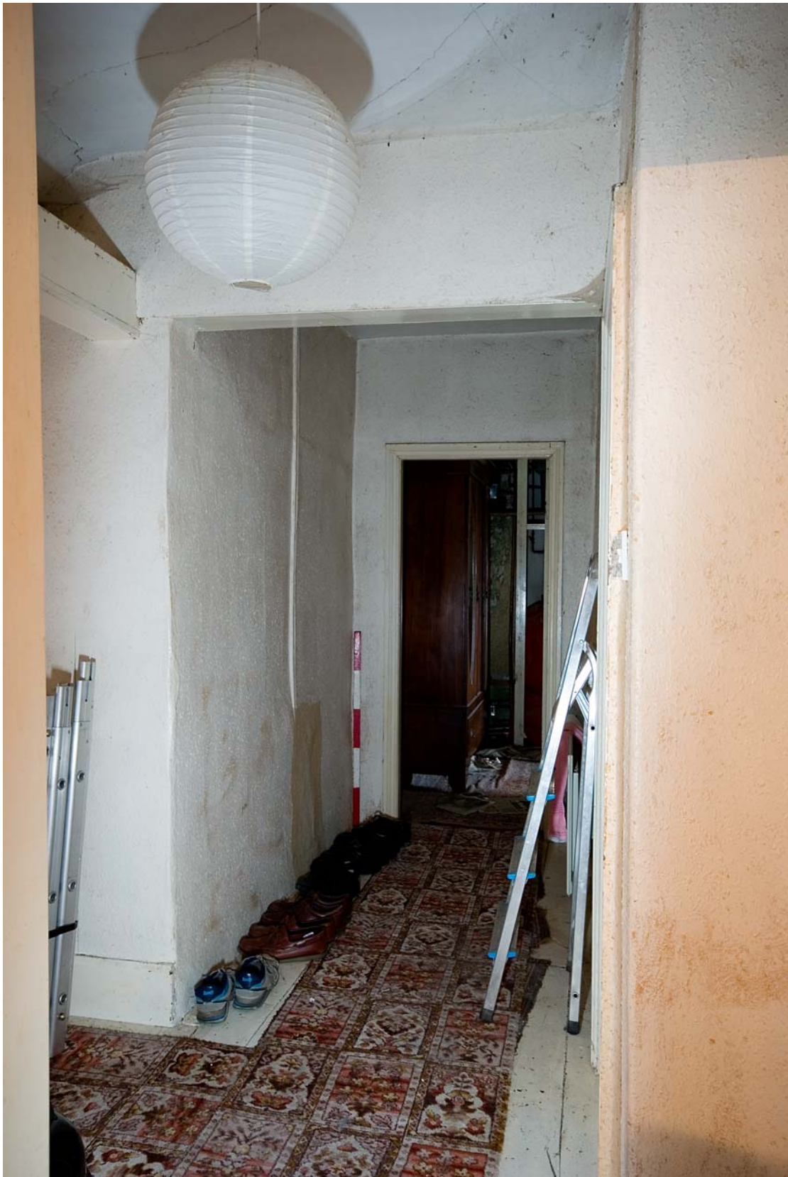
Plate 20: The exposed wall beam is just visible to the left of the picture. The height of the wall beyond this (extending above the wall beam) is evidence for the ceilings having been raised.
