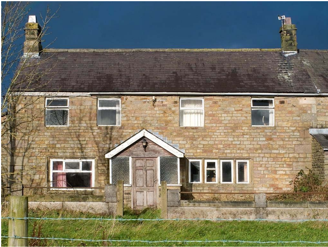
Plate 3: The principal elevation (south) of the farmhouse, showing the varying style of the windows.
