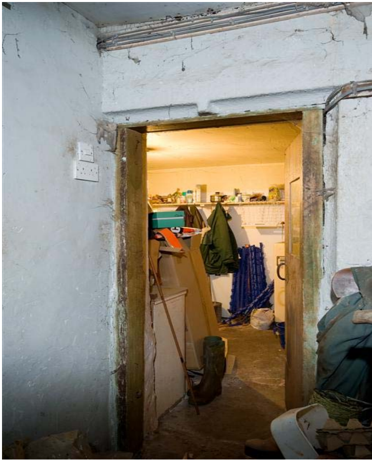
Plate 17: Doorway from the utility into the modern extension at the west end of the farmhouse. The doorway has been inserted into what was originally a two-light mullion window.
