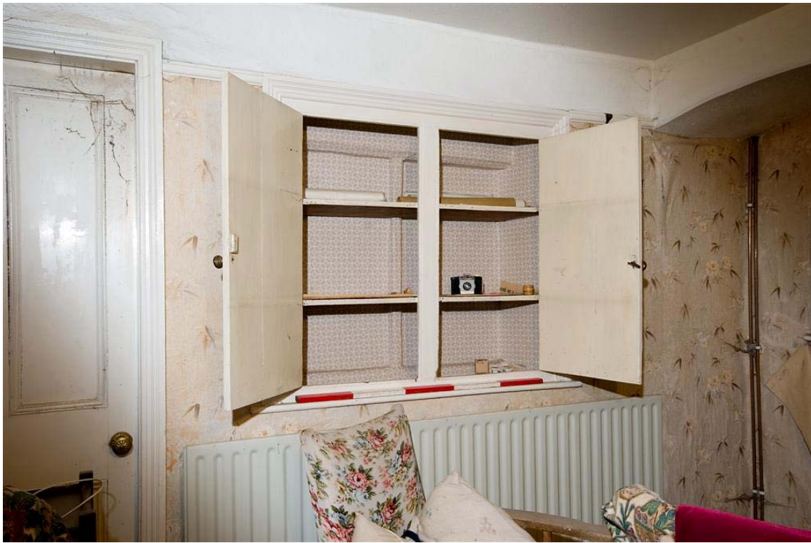
Plate 15: Mullion window concealed within a cupboard in the north wall of the living room.
