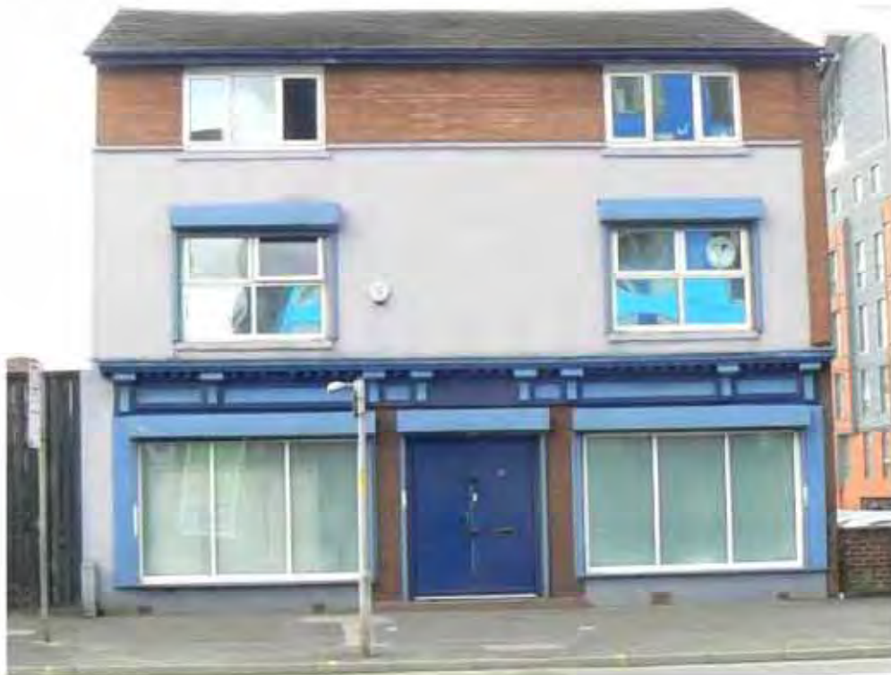
Plate 7: The north-east-facing elevation of 78 Great Ancoats Street
