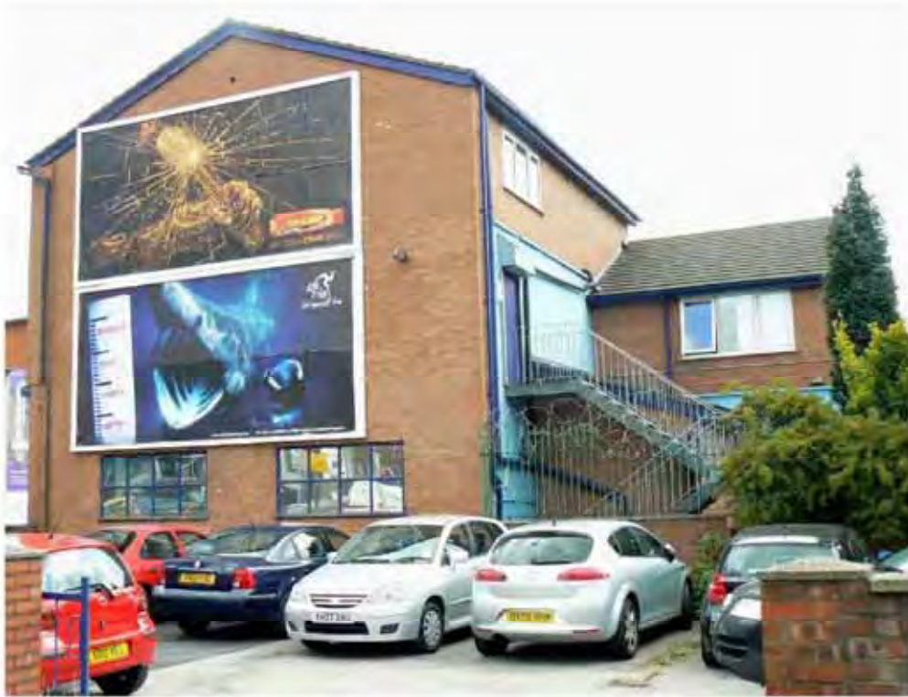
Plate 8: The north-east-facing elevation of 78 Great Ancoats Street
