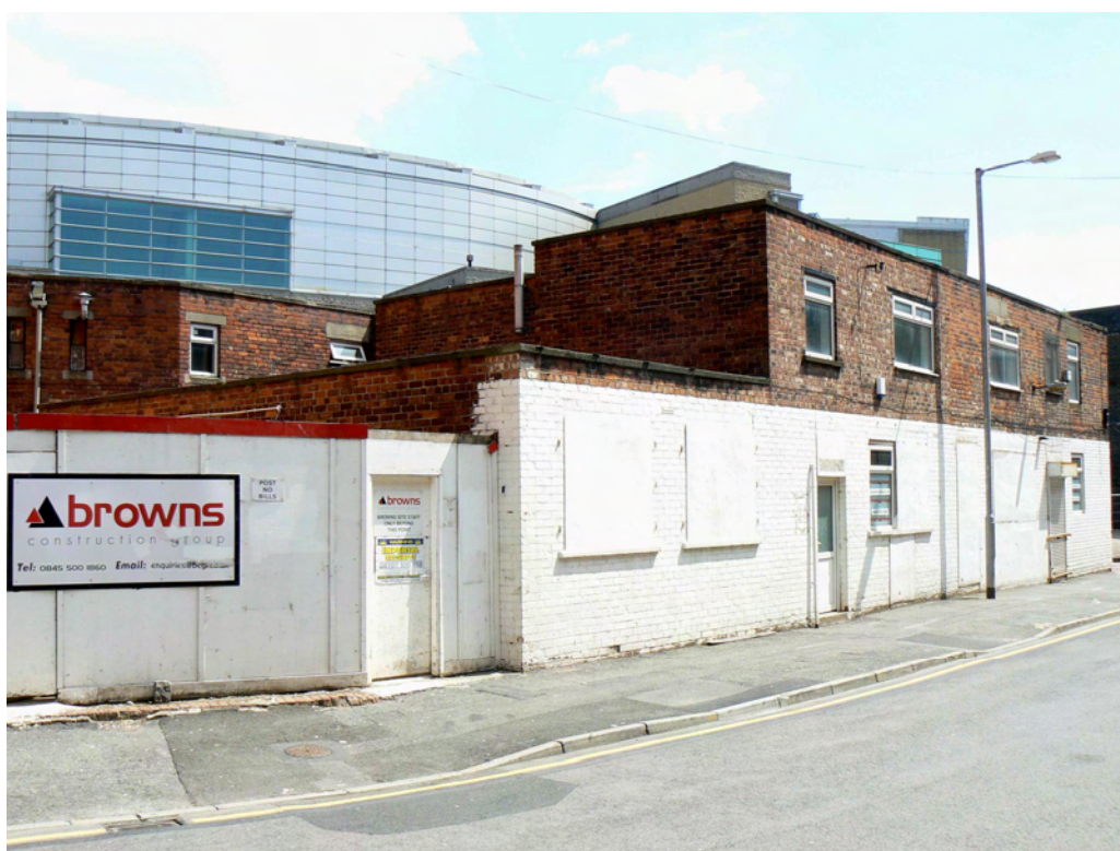
Plate 6: Looking east at 14 – 20 Mirabel (formerly Moreton) Street
