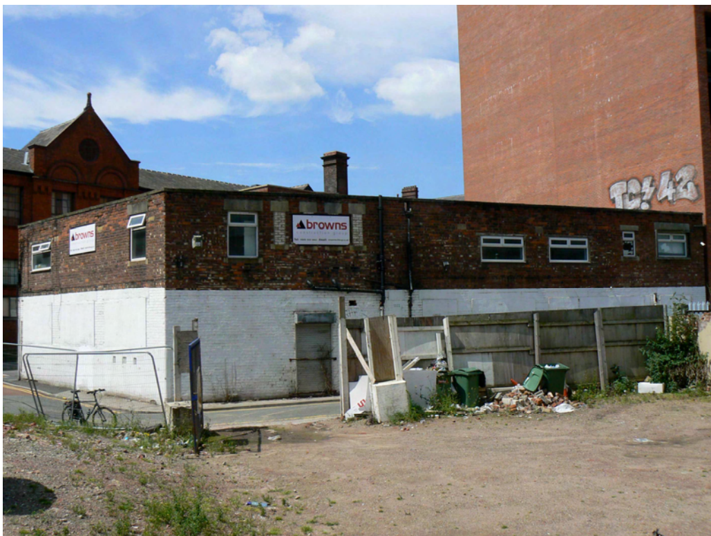
Plate 8: The rear elevation of 14 – 20 Mirabel (formerly Moreton) Street
