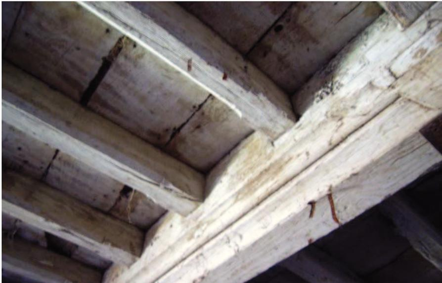
Plate 15 Reused beam in underside of floor in annexe
