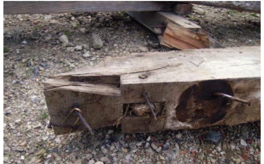
Plate 72 End of tie from dismantled shelter shed
