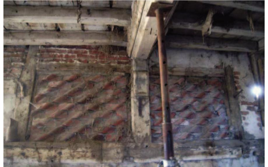
Plate 18 Reused chimney bricks in panel in east gable of barn.
