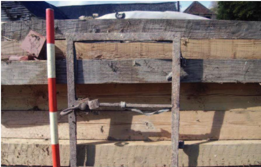
Plate 71 Window frame uncovered after shelter shed demolition
