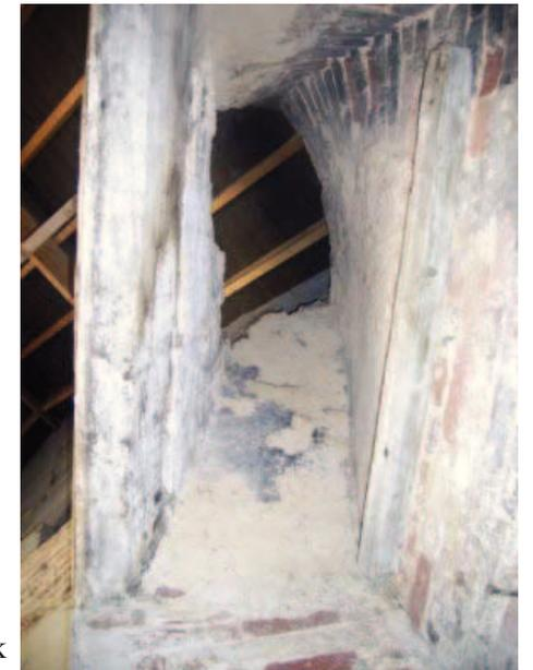
Plate 64 Hearth flue in garage block
