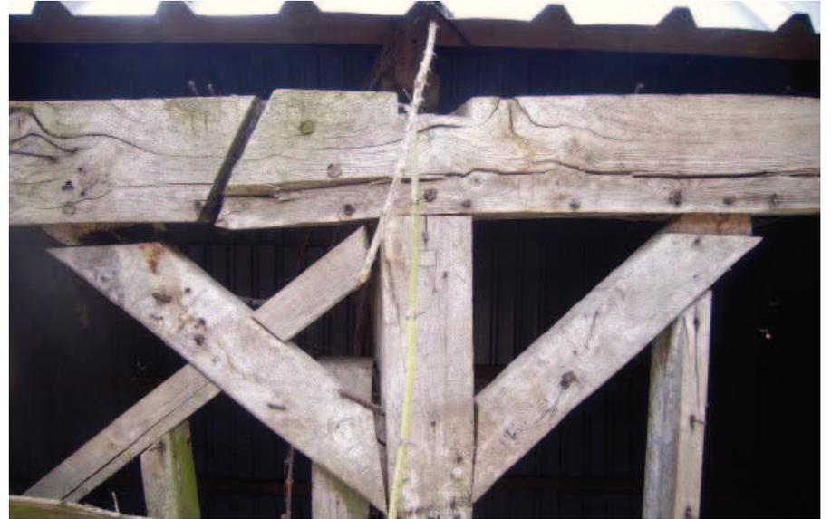
Plate 54 Detail of braces in shelter shed east wall
