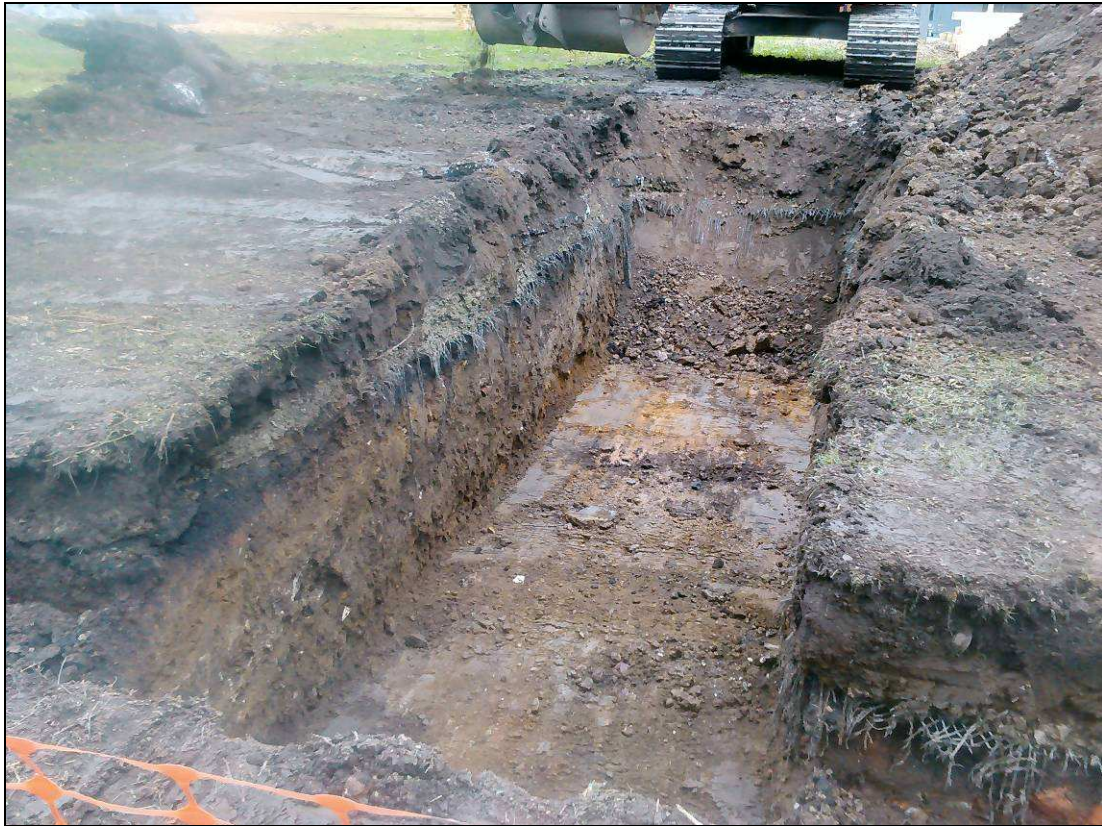
Plate 9: Natural sand observed during excavation of Trench 3
