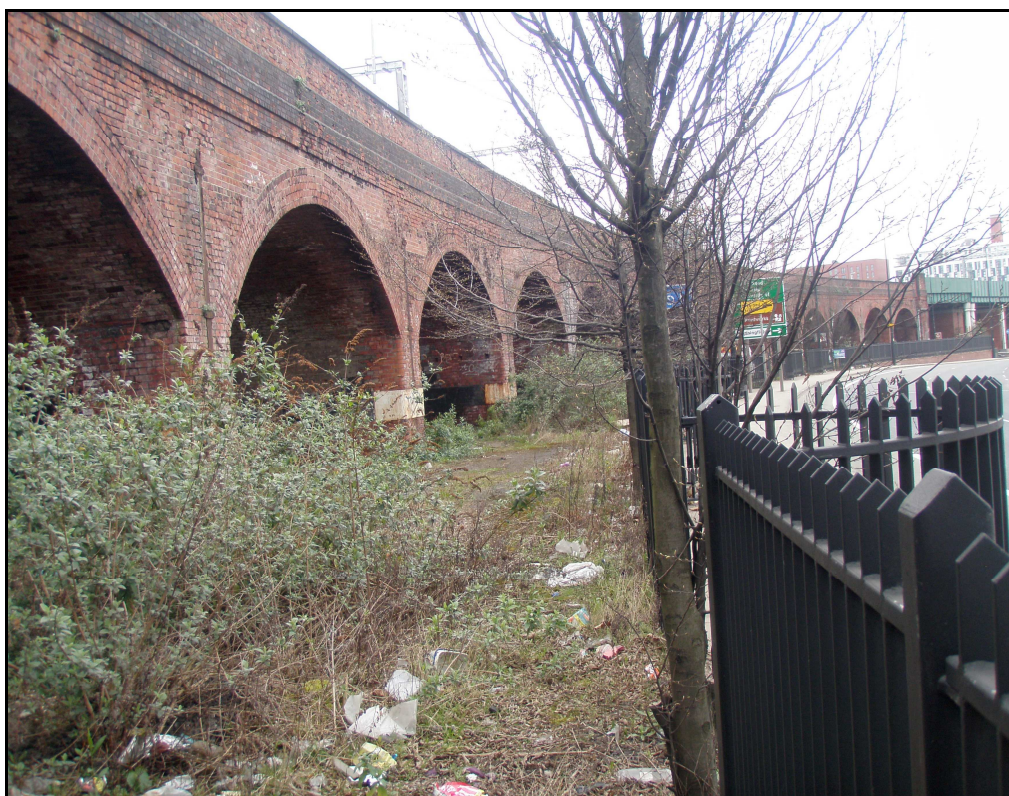
Plate 2. View along the viaduct (OA North, Site 91), leading to Irwell Street
