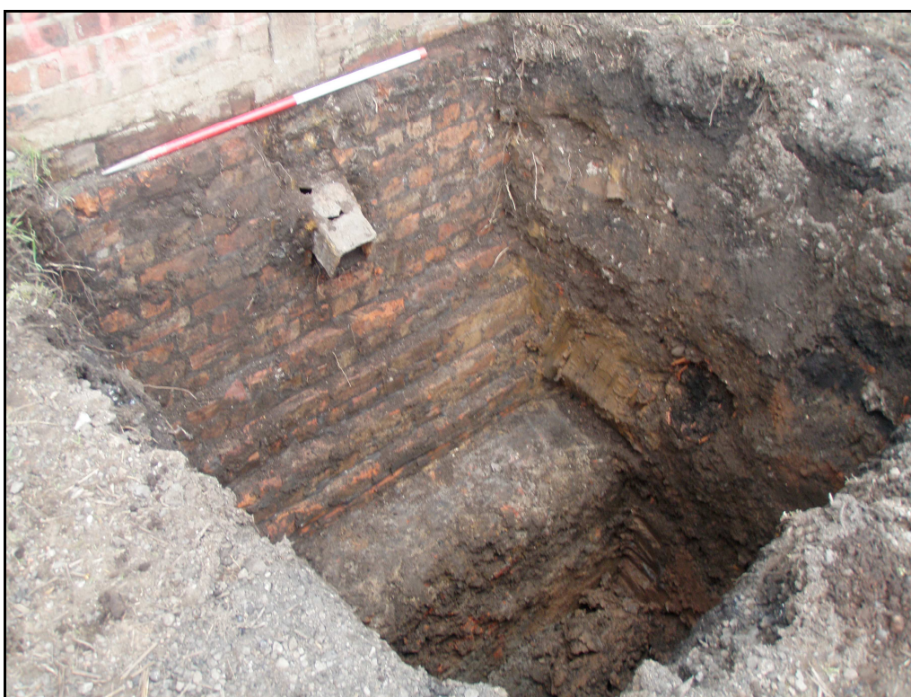
Plate 4. An example of the stepped viaduct arch foundations exposed during test pitting, from pit G4FP06 between arch 13 and 14
