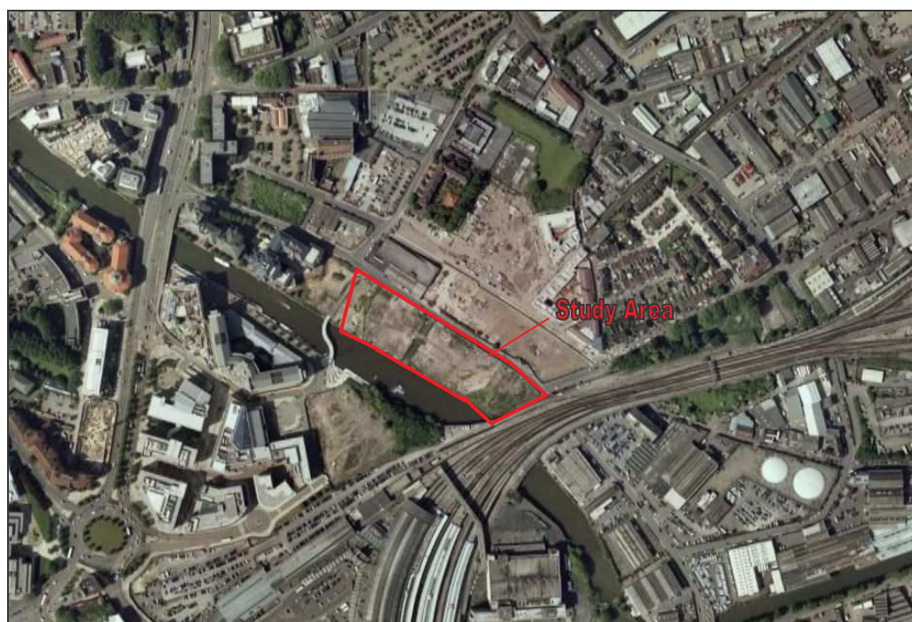
Plate 1: Aerial view of the site prior to development
