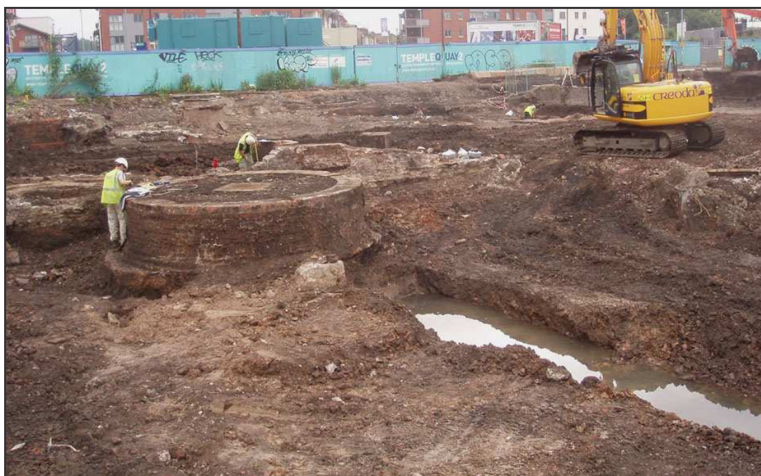
Plate 20: Late circular brick structures, looking north-east
