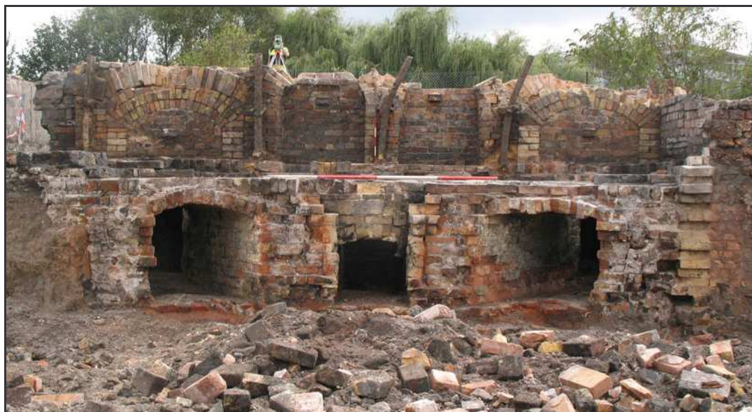
Plate 13: Elevations of flues in Furnace C, looking south
