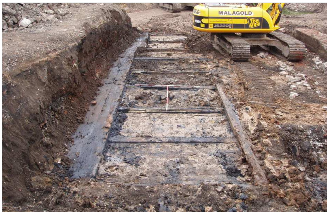
Plate 19: Later timber structure 1090, looking south
