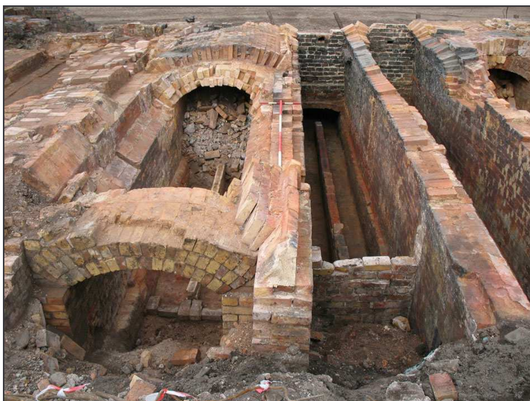
Plate 12: Furnace C regenerative furnace chambers, looking north. The wider chamber carried air and the narrower carried gas
