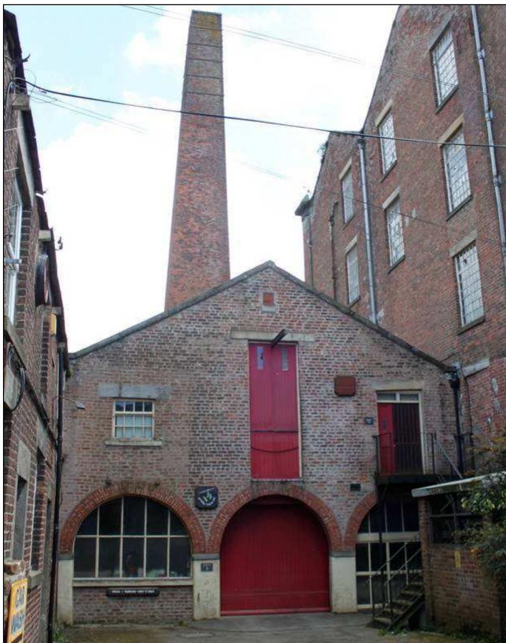
*Plate 25: The two-storey boiler house abutting the north side of the main mill block, with the full-height chimney visible to the rear. The boiler house lies beyond the boundary of the Application Area*
