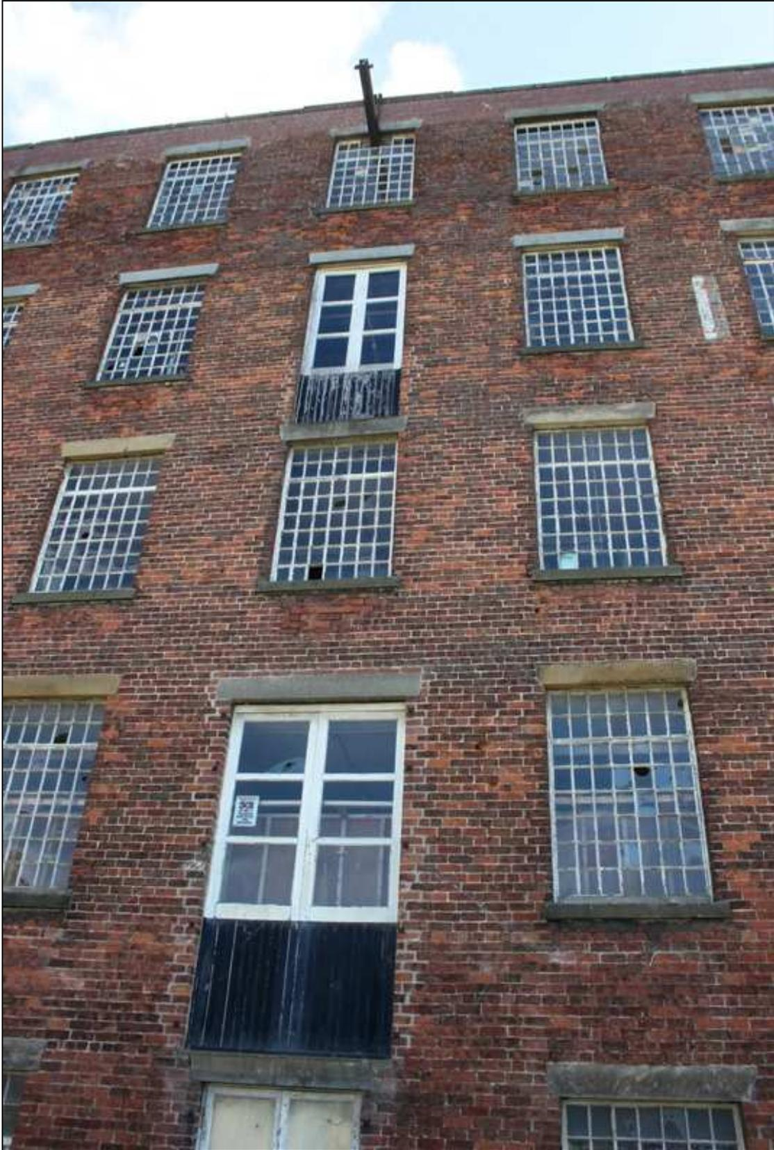
*Plate 7: Central loading loophole in front elevation*
