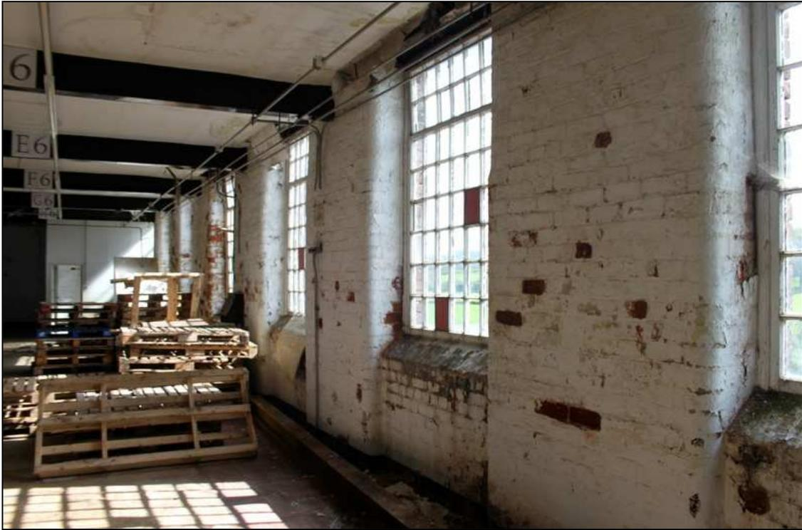
*Plate 8: Interior view of the 56-light windows with top rows on opening swivel tilt*
