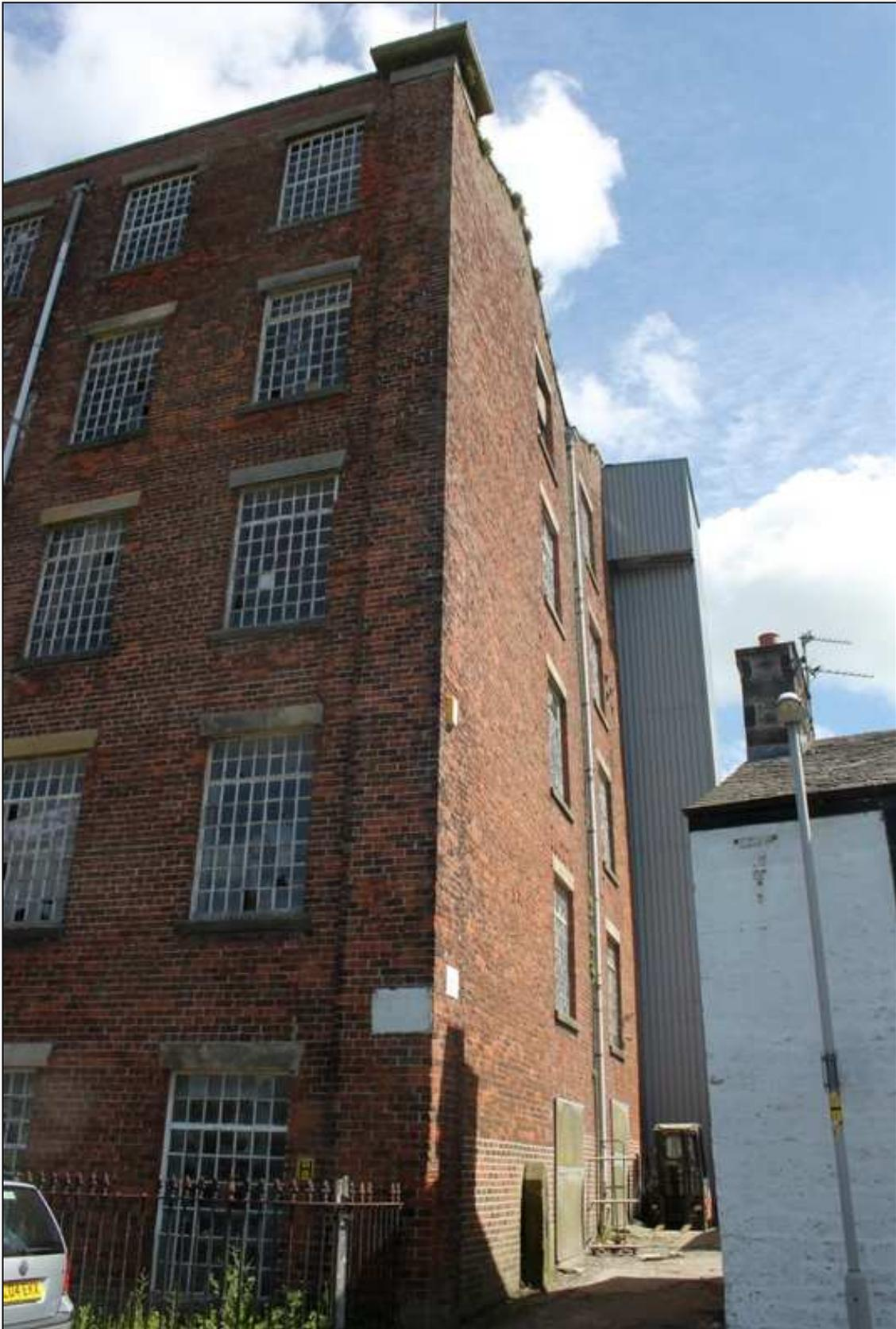
*Plate 13: The southern gable of the mill, with late hoist tower clad in metal sheeting*
