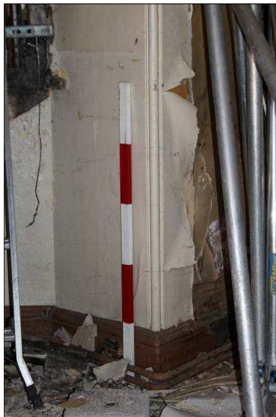
Image 3: Roll-moulded jambs of canted bay window on the ground floor (1m scale)
