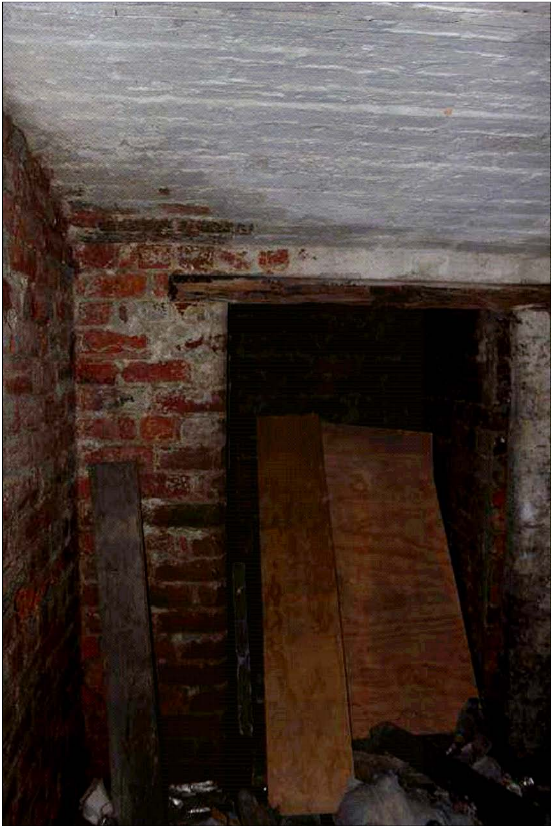
Image 15: Coal chute in eastern wall of the cellar
