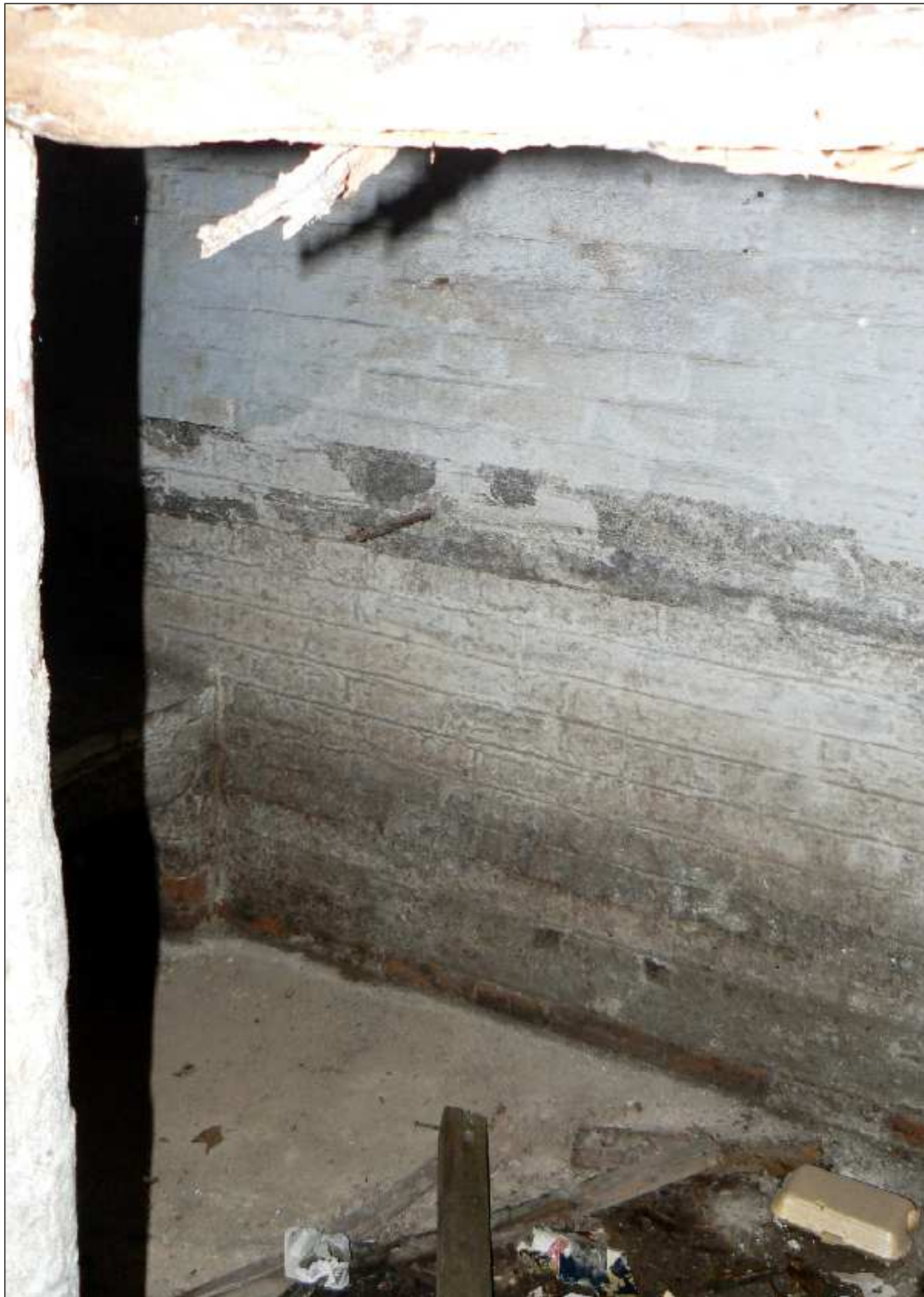
Plate 23: Former location of shelf denoted by projecting flat iron bars and low stone shelf, just visible to left at southern end of cellar
