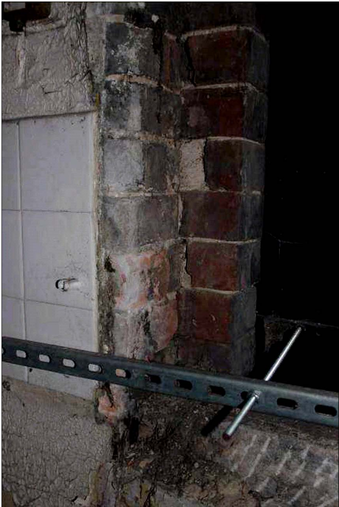
Image 11: Filleted and stopped jambs on kitchen window surrounds at ground-floor level
