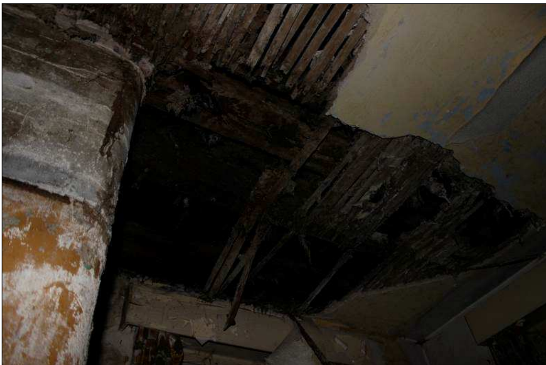
Image 8: Transverse joists above sawn lathes in south-western corner of back room at ground-floor level
