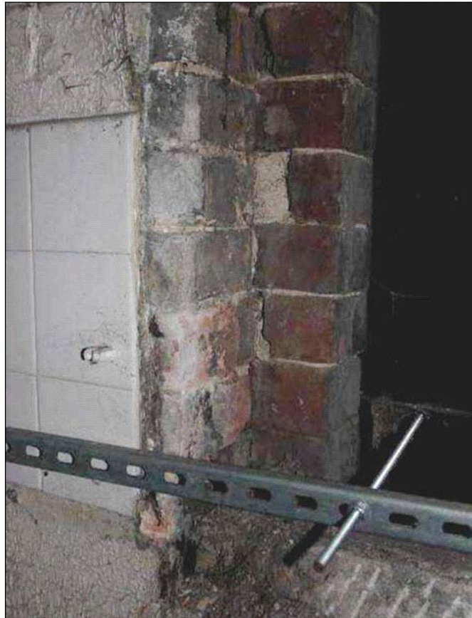
Plate 18: Filleted and stopped jambs on kitchen window surrounds
