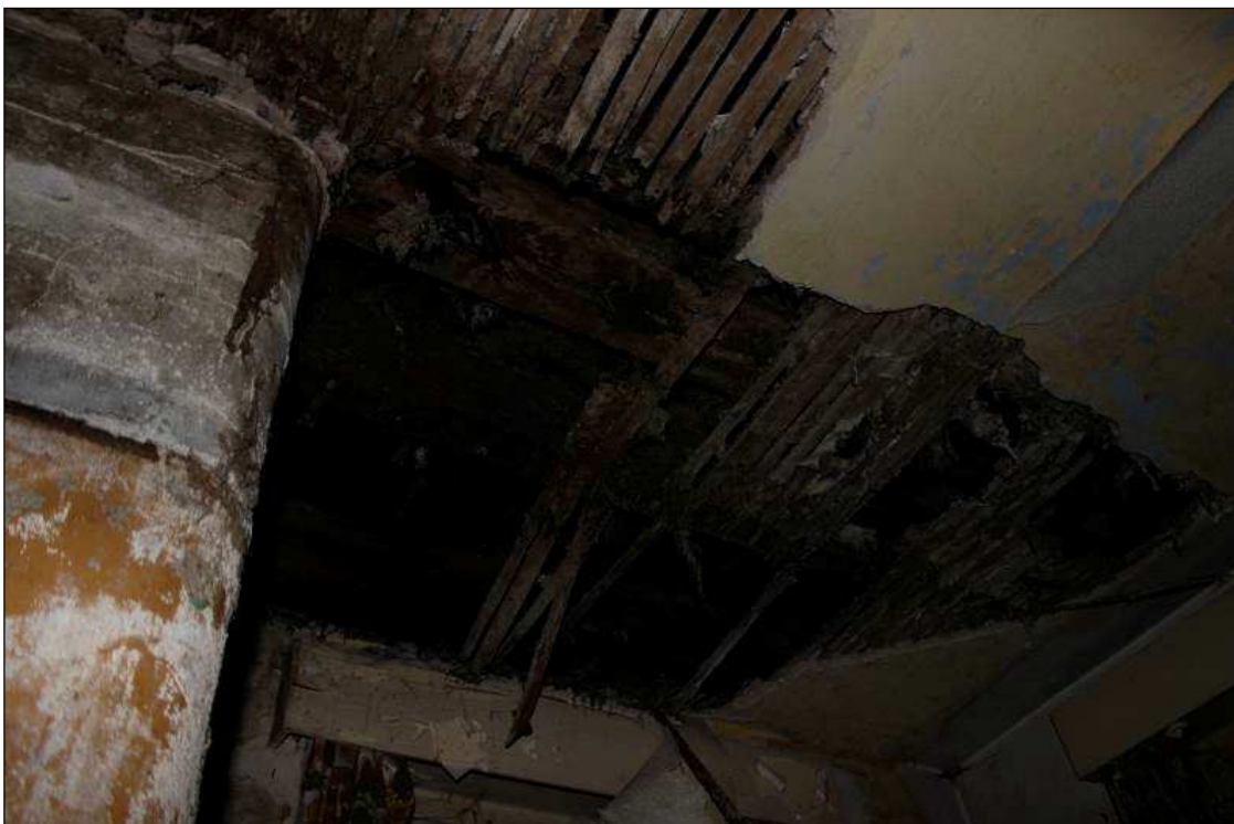
Plate 15: Transverse joists above sawn lathes in south-western corner of the back room
