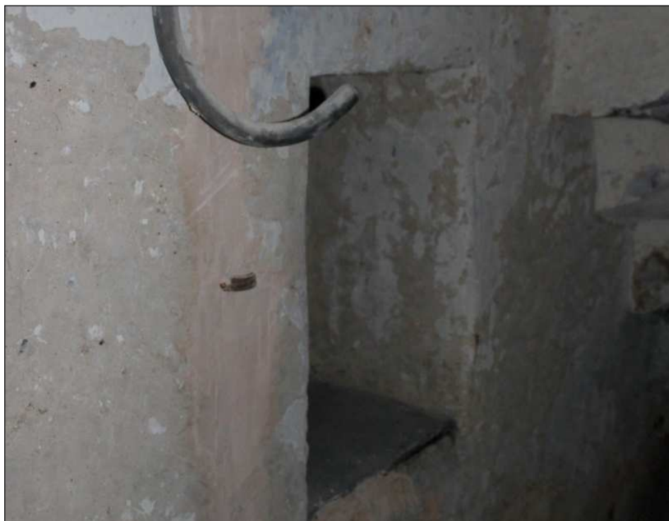
Plate 20: Keeping hole below stairs in Varley Street extension
