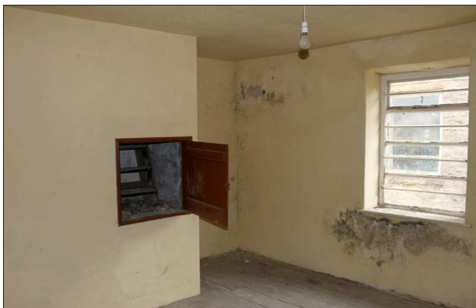
Plate 23: Access hatch to roof space of Varley Street extension
