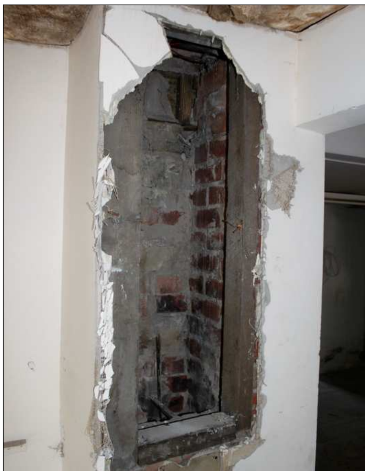
Plate 8: Flue within 33 Trafalgar Street at first-floor level
