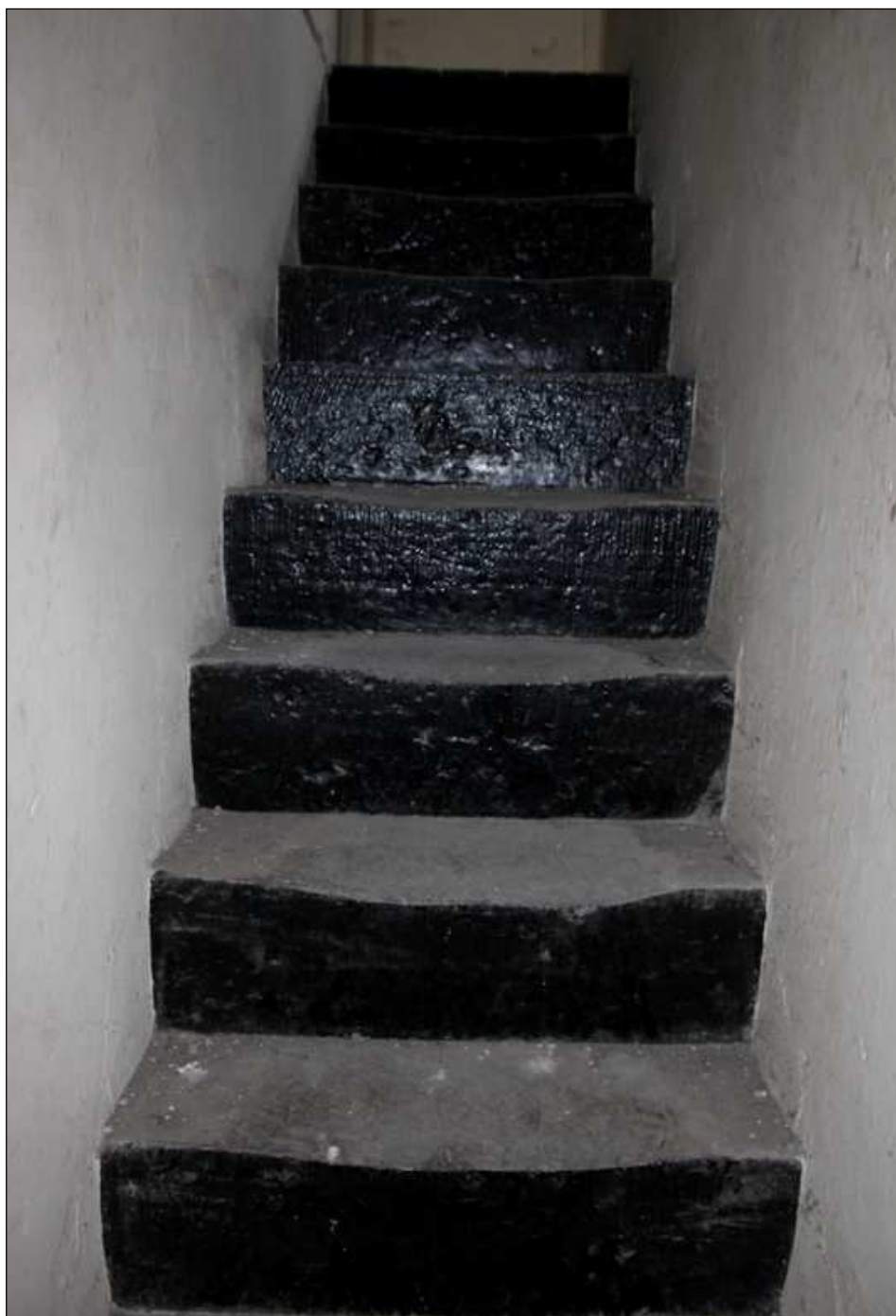
Plate 26: Straight stone stair in Derby Street extension
