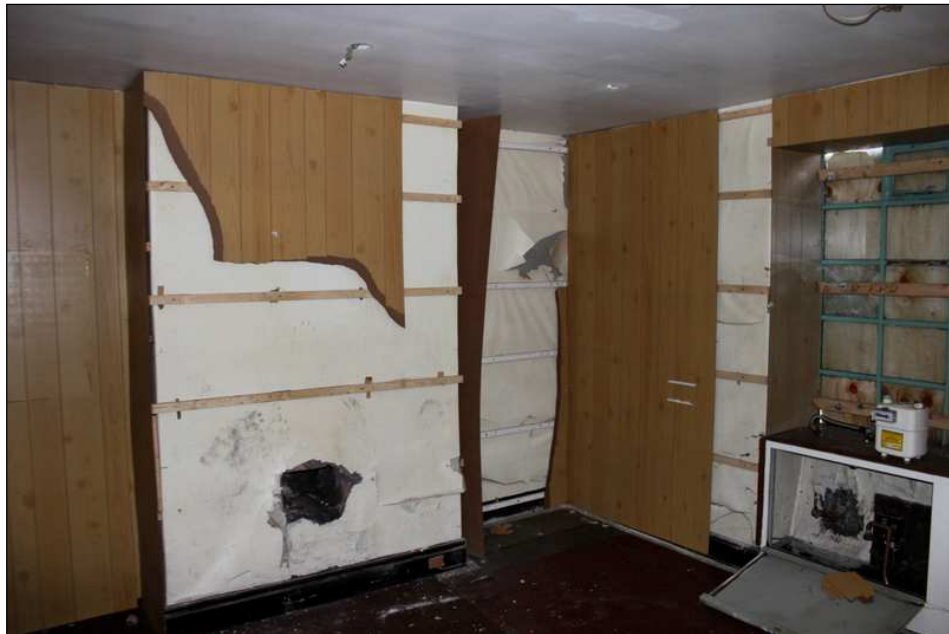
Plate 24: Front room of Derby Street extension
