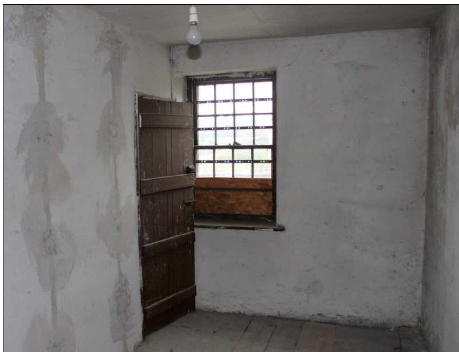
Plate 33: original sash window in small rear room
