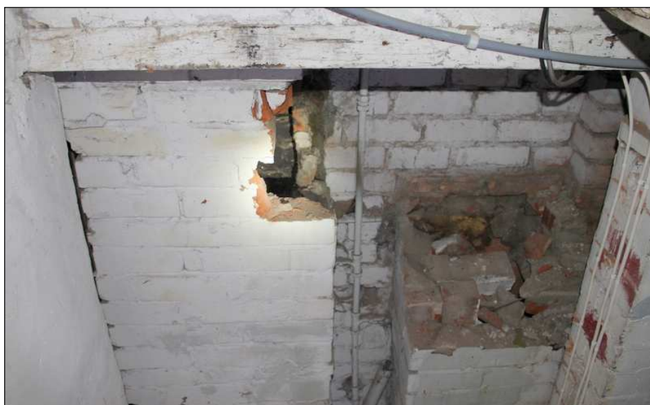
Plate 10: Flues in the south party wall on Derby Street
