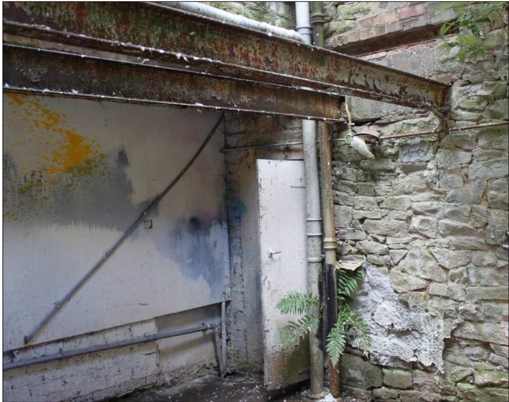
Plate 14: Extant and blocked doorway into courtyard
