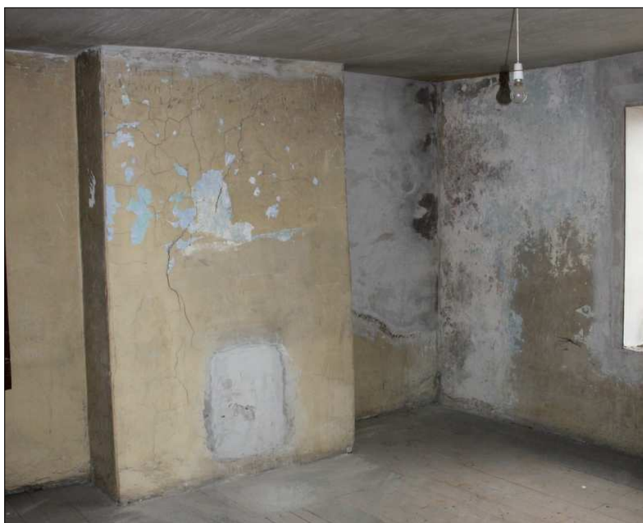
Plate 31: Blocked fireplace in south wall of Derby Street extension
