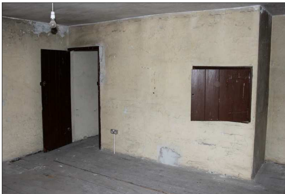
Plate 30: Front room of Derby Street extension, with attic hatch above stairs
