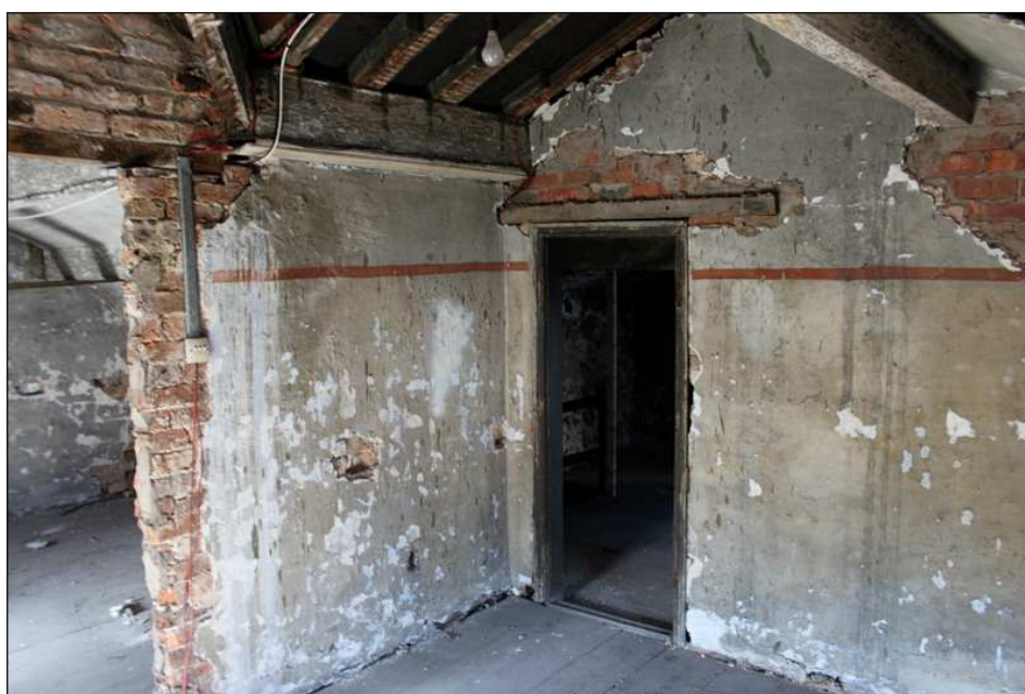
Plate 5: Painted plaster on original partitions
