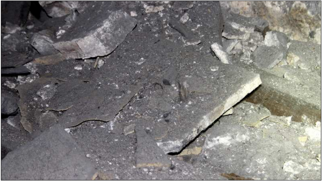
Plate 36: Timber-pegged roofing flagstone in Derby Street extension
