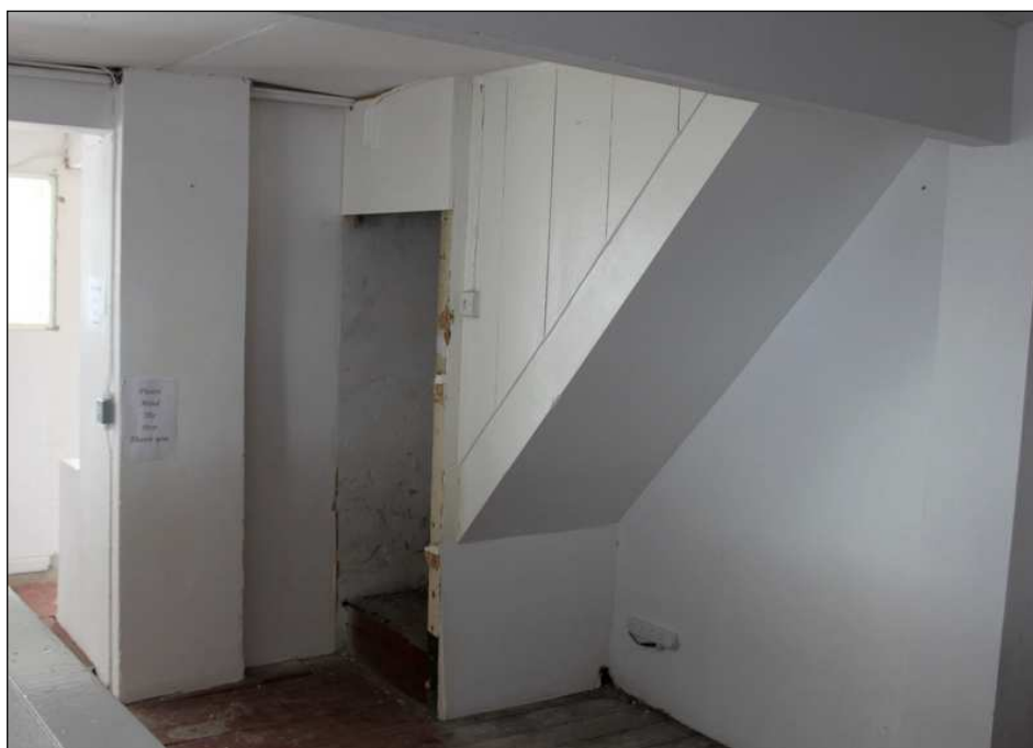
Plate 13: Timber stair to second floor in southern property on Varley Street
