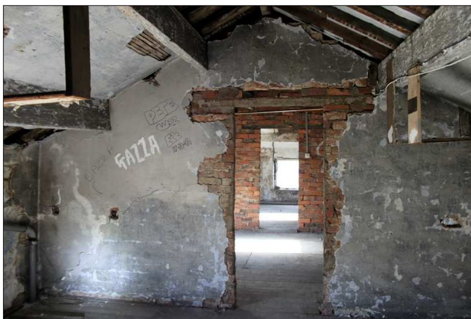
Plate 4: Original partitions at second-floor level
