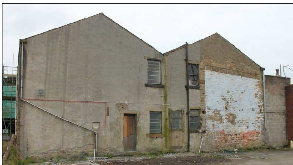
Plate 18: Northern gable of the later extensions
