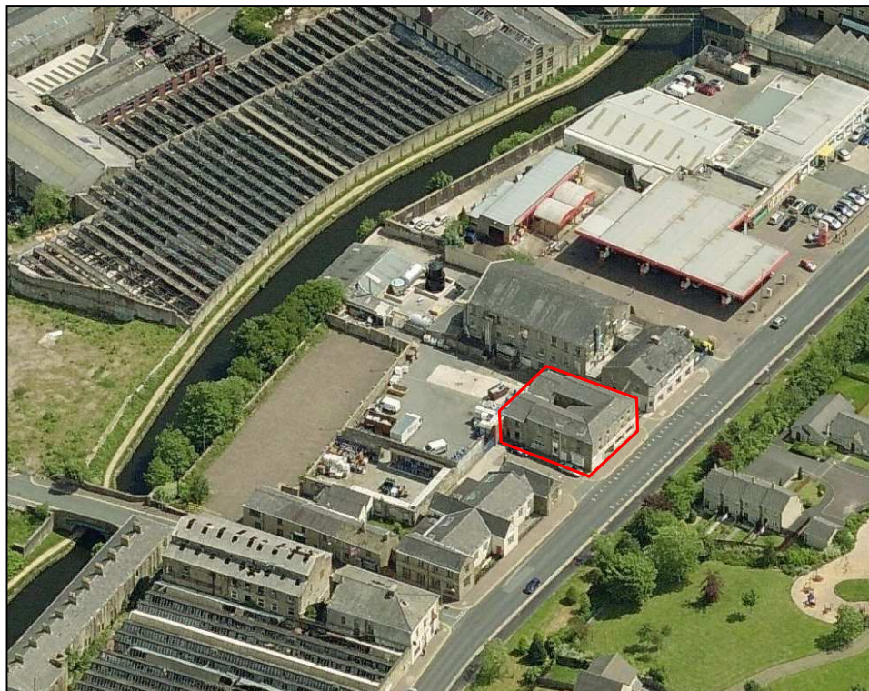
Plate 1: Recent aerial view of the study area, prior to the demolition of the properties adjacent to 29-35 Trafalgar Street
