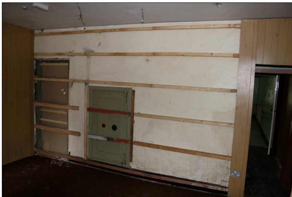
Plate 25: Rear wall of front room of Derby Street extension
