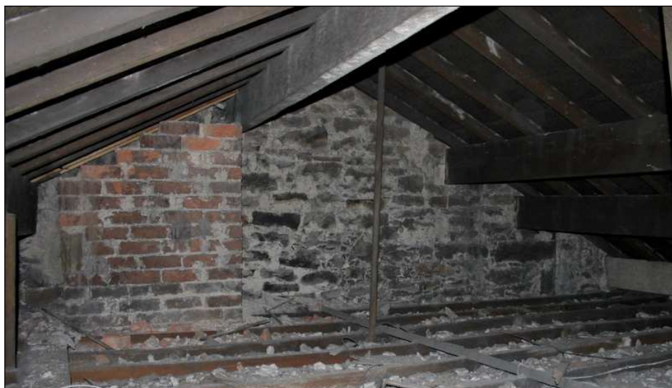
Plate 22: Roof space of extension to Varley Street properties
