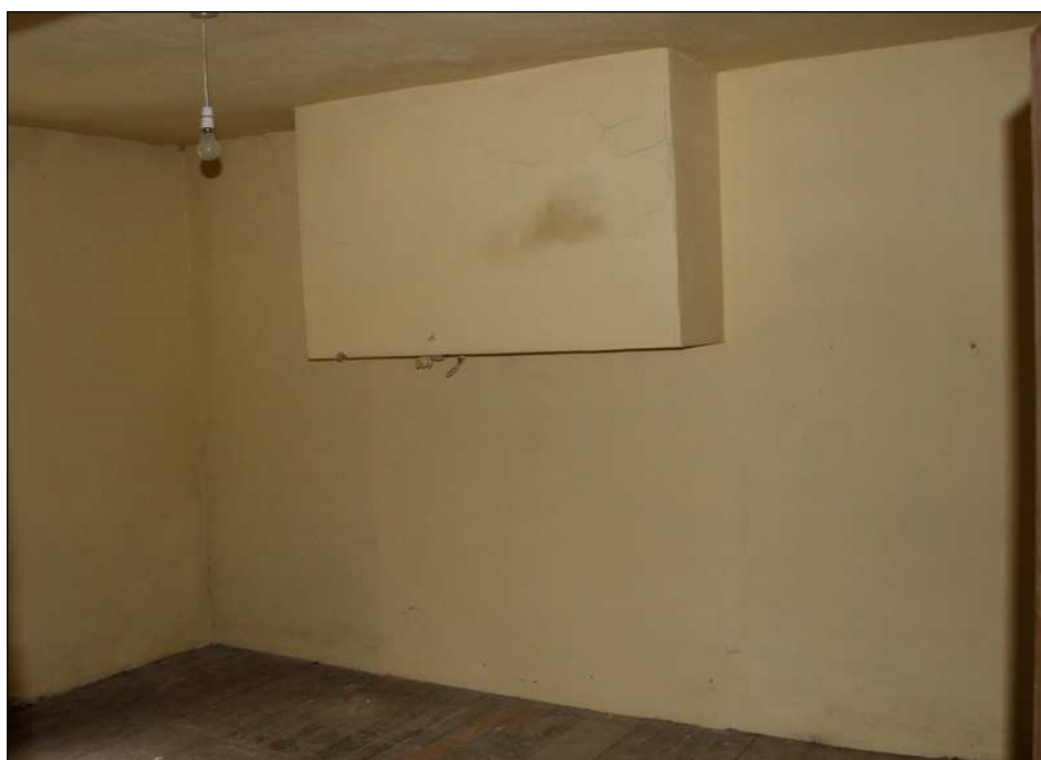
Plate 21: Remains of chimney breast at first-floor level
