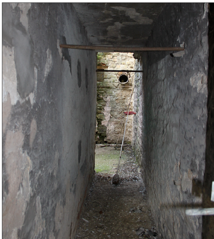
Plate 16: Access passage from Varley Street to the enclosed courtyard
