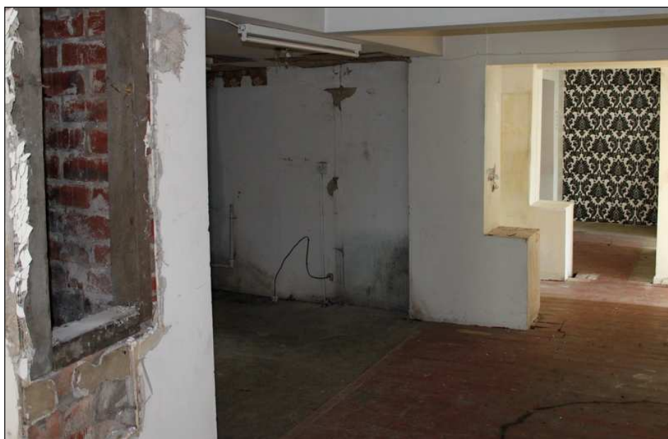
Plate 9: Capped flues within 29 and 31 Trafalgar Street
