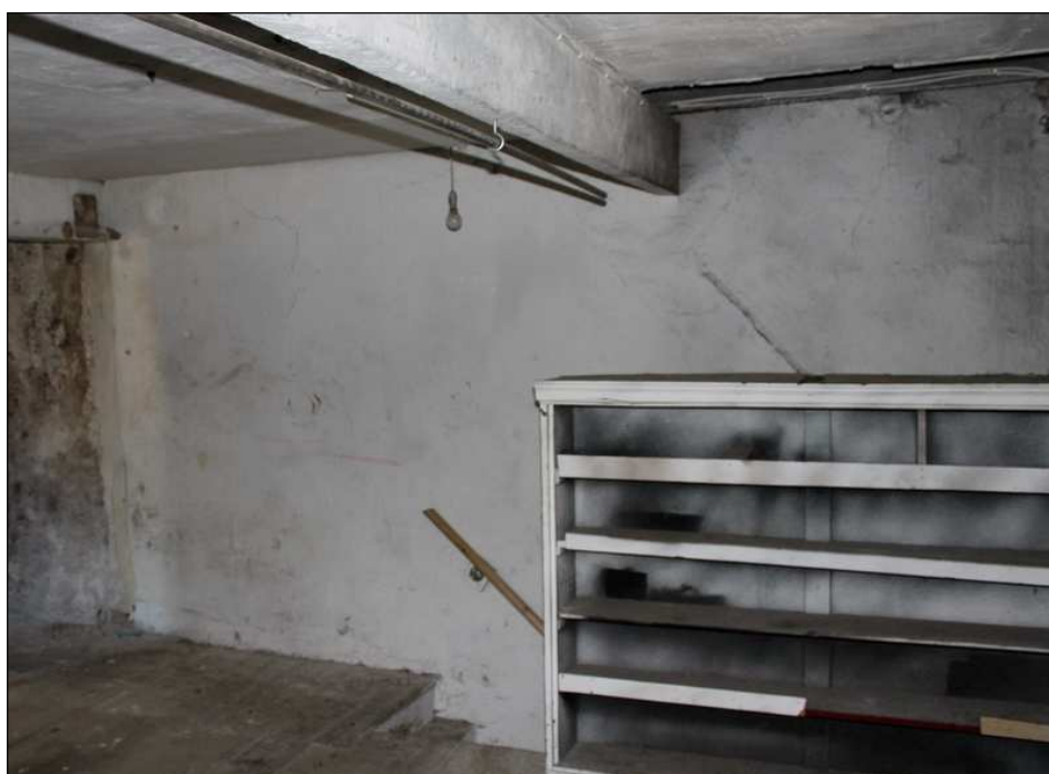
Plate 12: Scar for further stair to second floor in southern property on Derby Street
