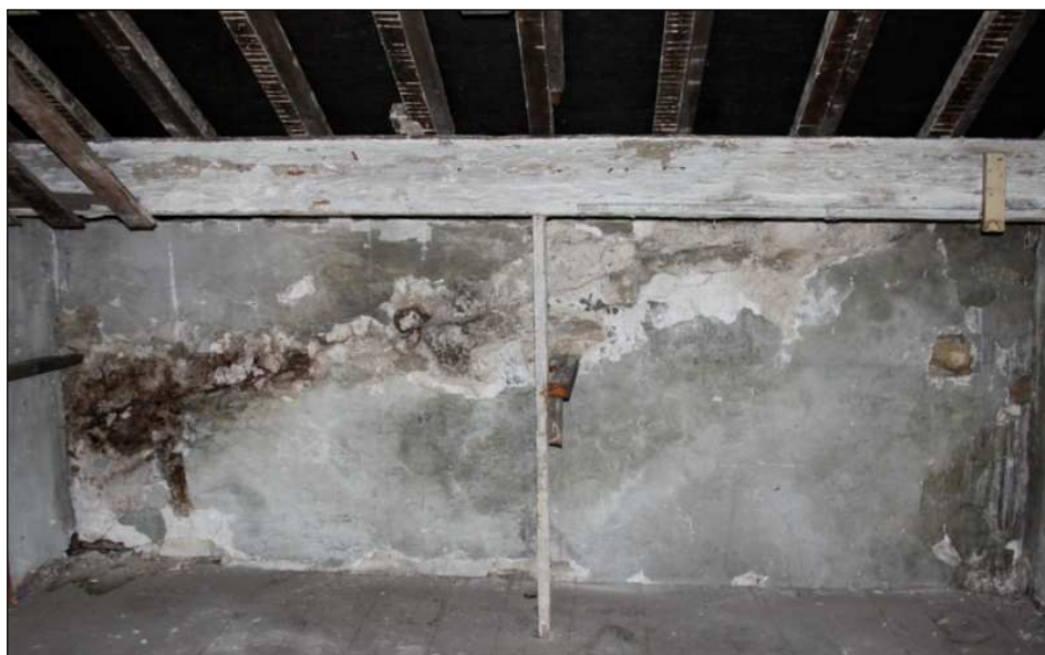
Plate 17: Roof scar for cottage on south side of courtyard
