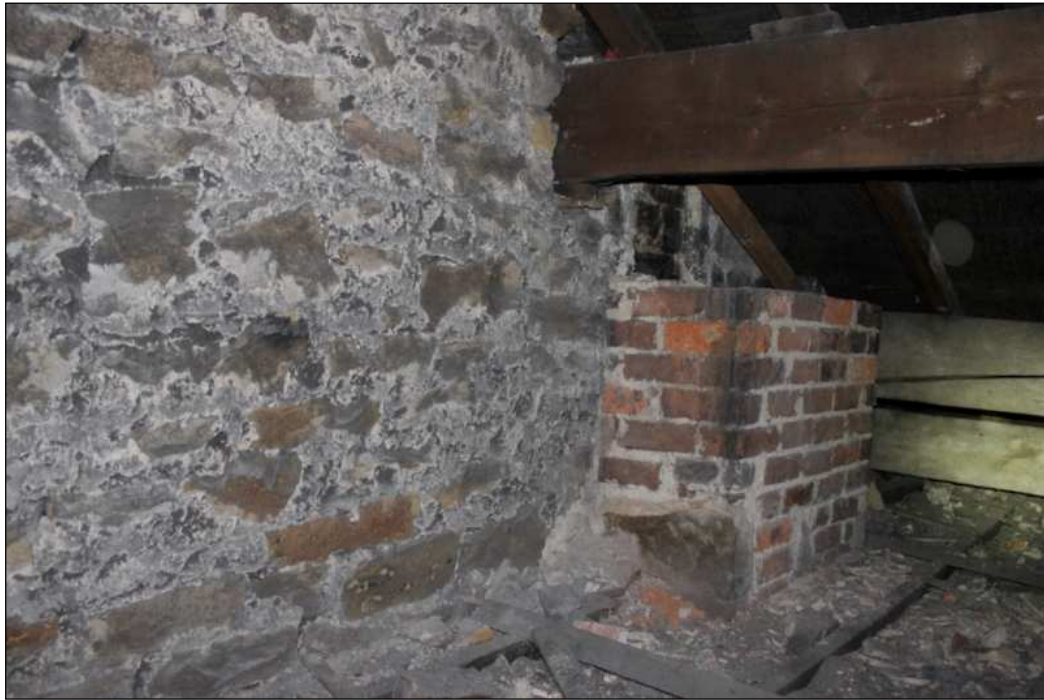
Plate 34: Chimney stack for fireplace in front room
