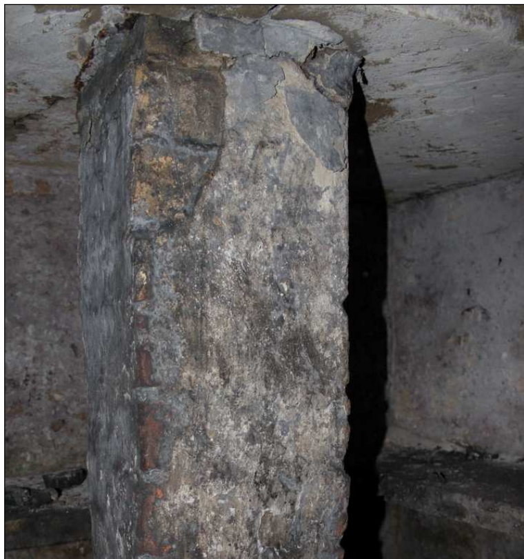
Plate 28: Brick pier with sandstone cappings supporting floor above cellar
