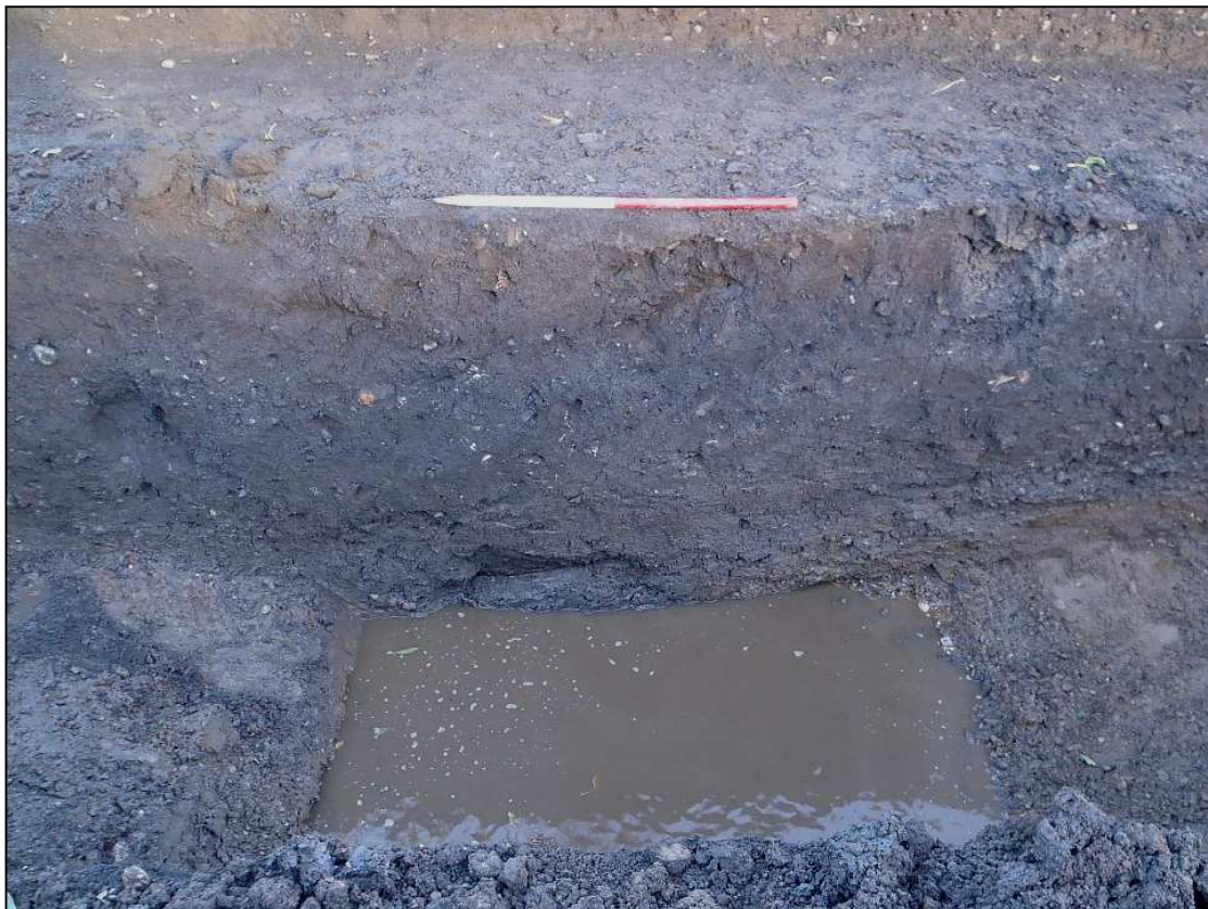
Plate 10: South-facing section of ditch 1807, showing ingress of groundwater
