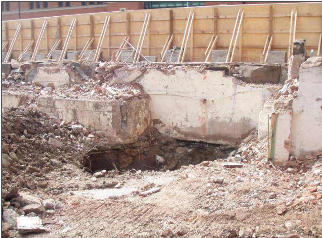
Plate 7: Trial pit 3 through basement, looking south
