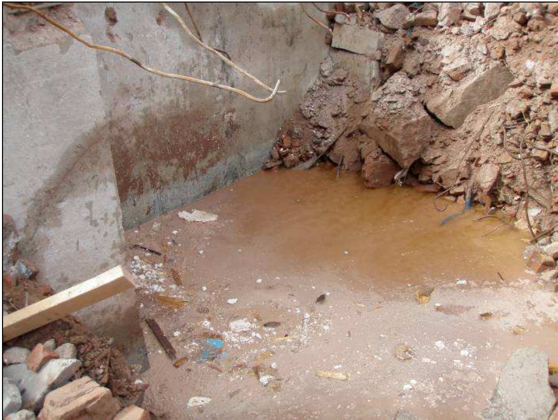
Plate 6: Trial pit 2 below sub-station, looking west
