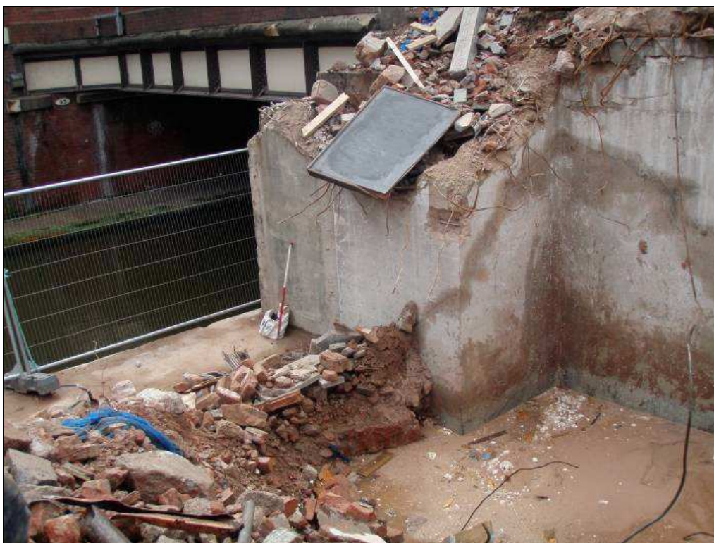
Plate 2: Excavated southern corner of the sub-station, looking south
