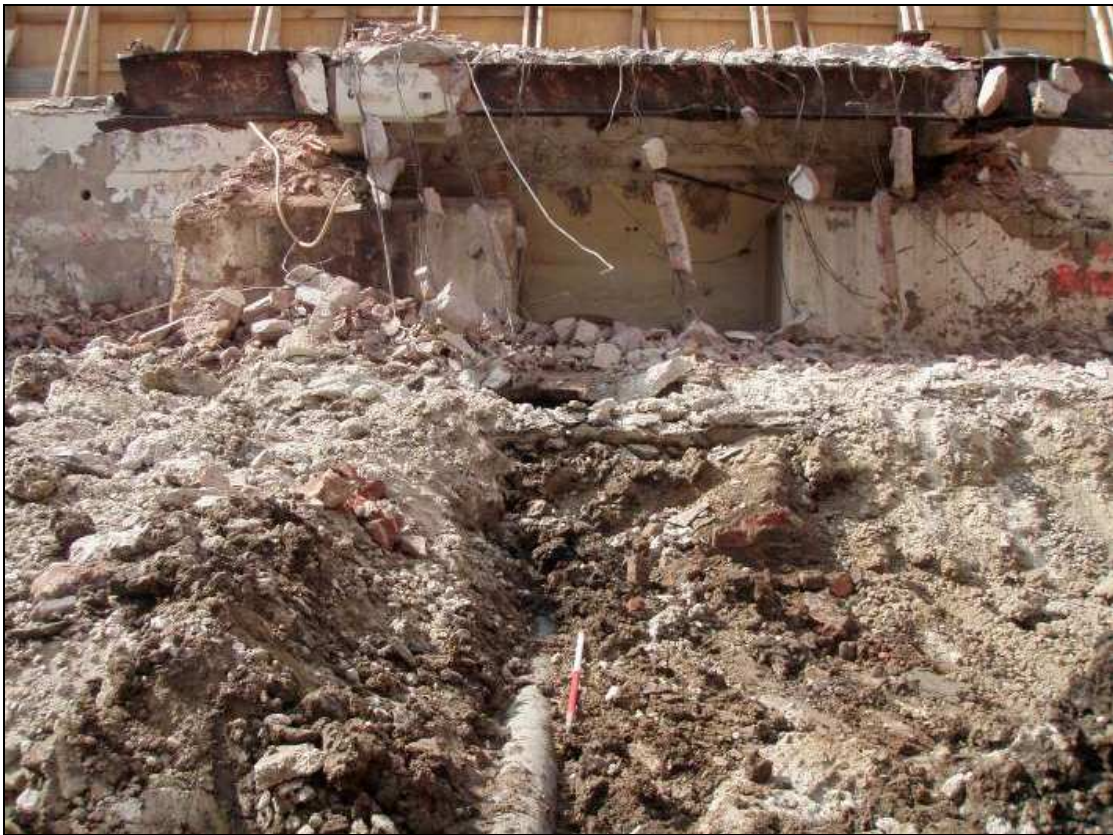
Plate 8: Trial pit 4, including water pipe, looking south-west
