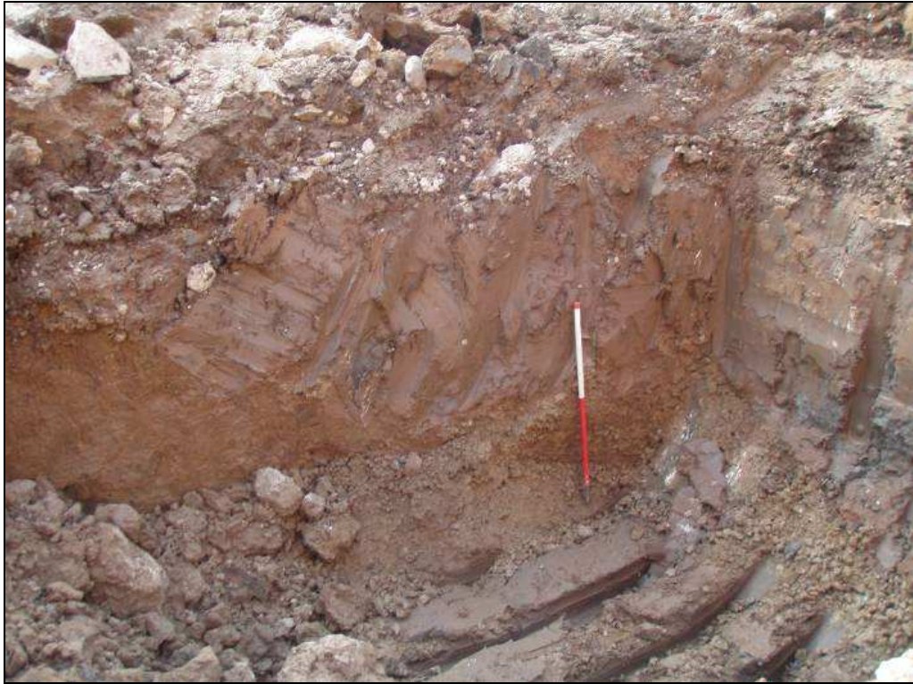
Plate 5: Trial pit 1 below flag surface, showing natural clay, looking north-west
