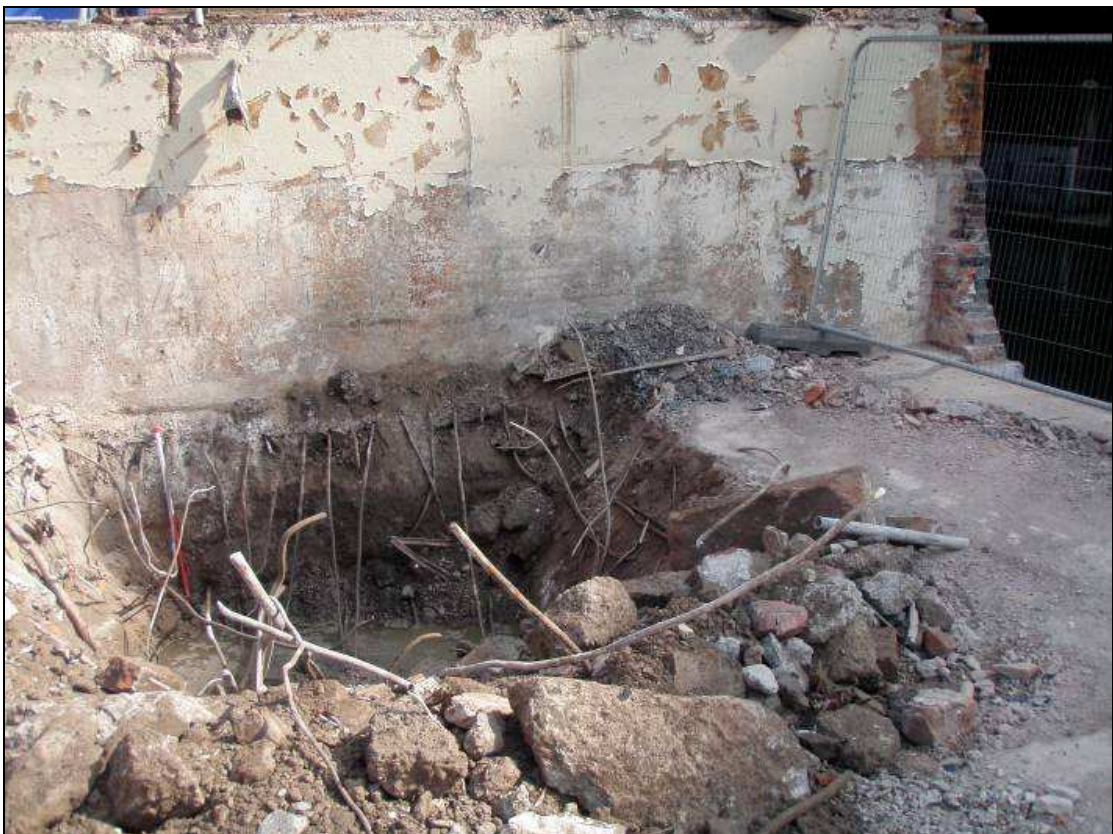
Plate 9: Trial pit 5 through basement, looking north-west
