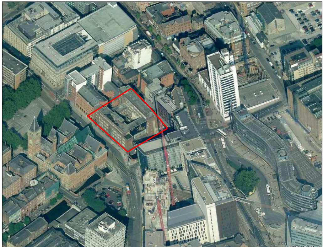
Plate 1: Aerial view across the study area prior to the demolition of the Employment Exchange
