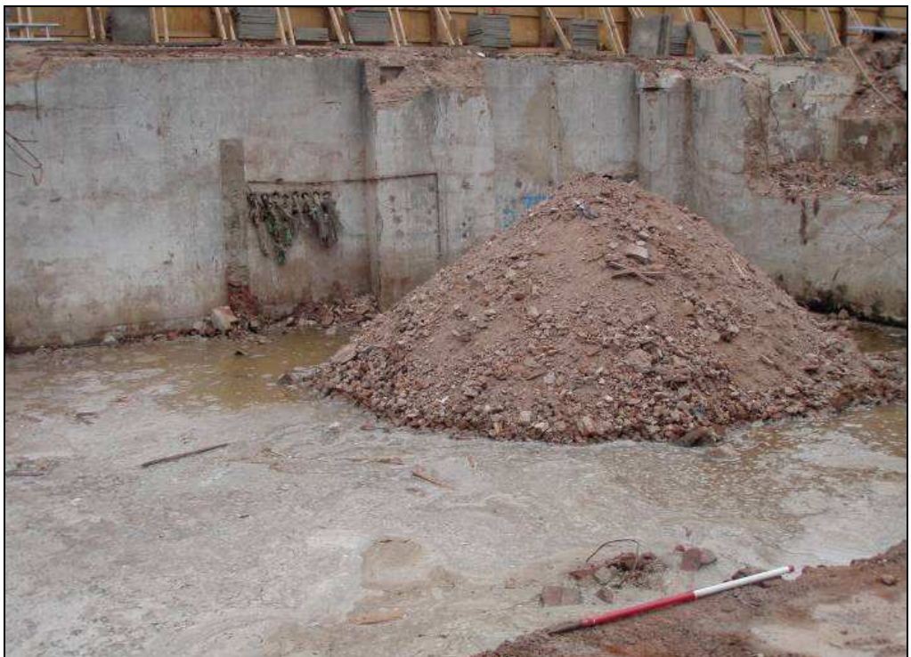
Plate 4: Deep concrete basement, looking north
