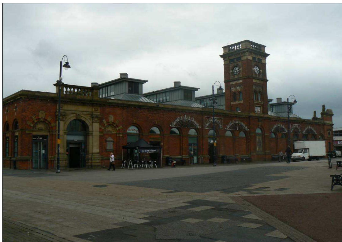
Plate 12: The market hall, a Grade II listed building
