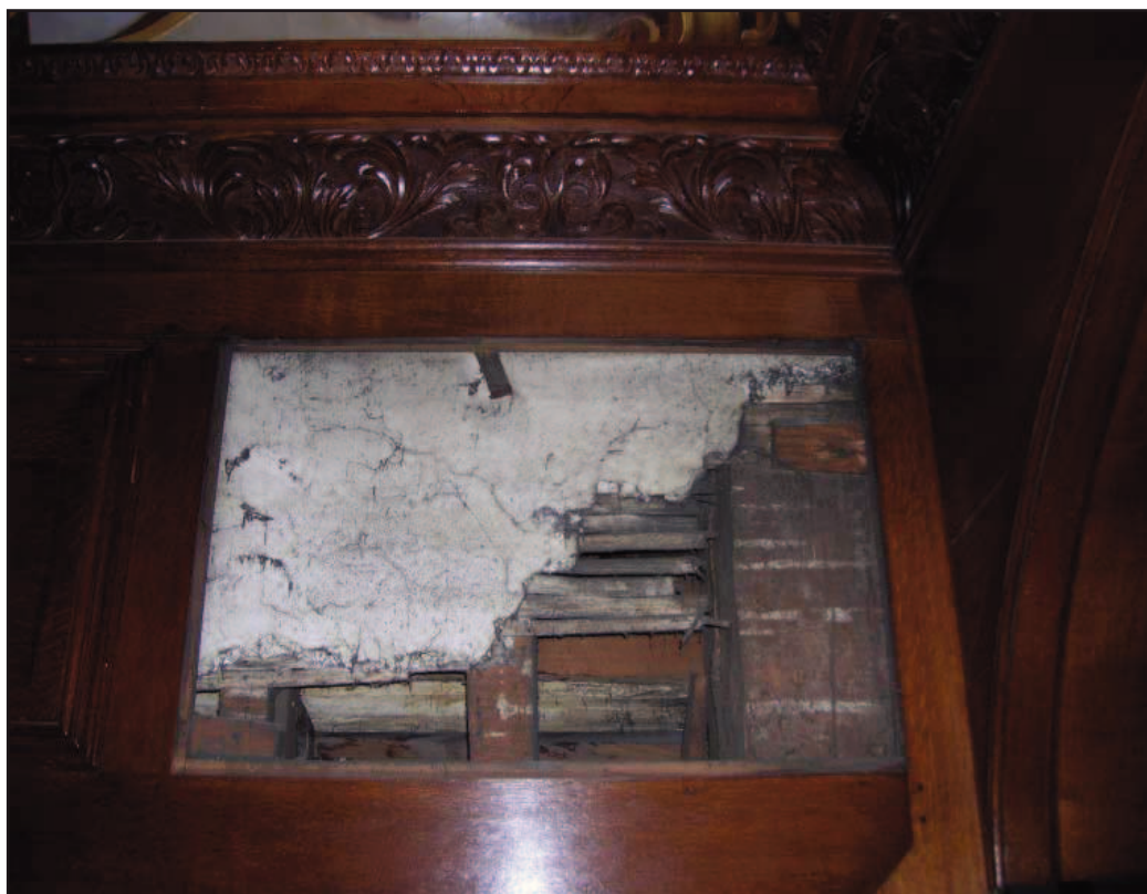
Plate 19: Royal Pew, Chapel Royal, Hampton Court Palace: Royal Pew, lath and plaster and timber framework, south elevation of south partition.
