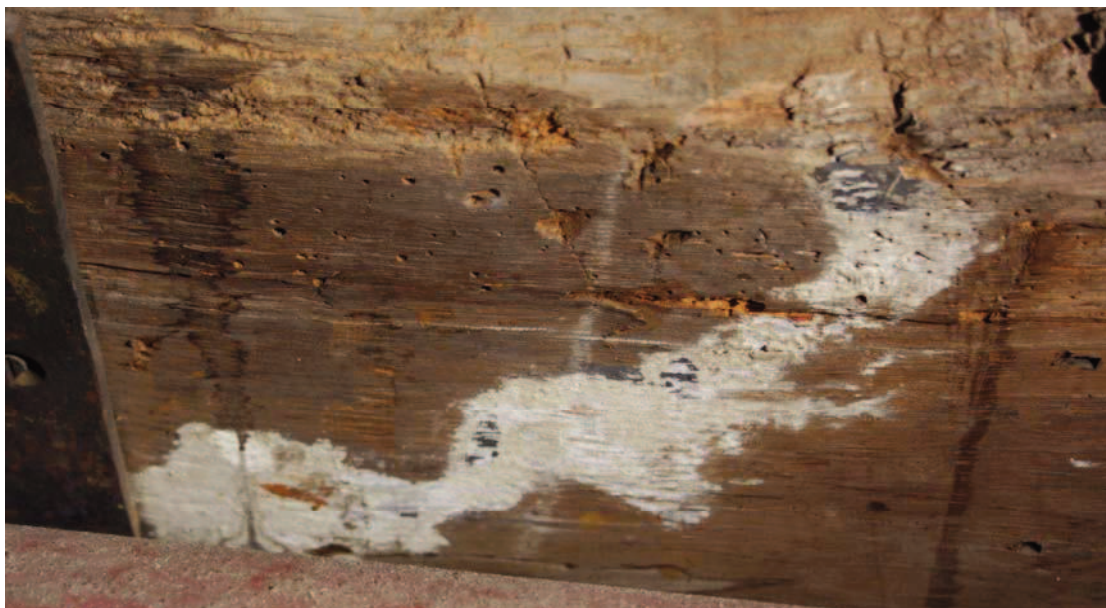
Plate 3: detail of white preparatory layer surviving on the east face of the balcony beam. The remains indicate the outline of a former oriel window - see Plate 1
