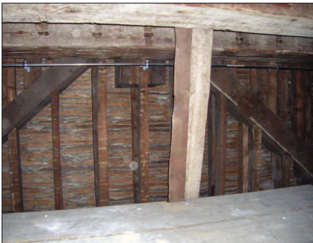
Plate 54: Royal Pew, Chapel Royal, Hampton Court Palace: Small room over Thornhill Ceiling, east elevation, supporting braces and remains of central post (post 4)
