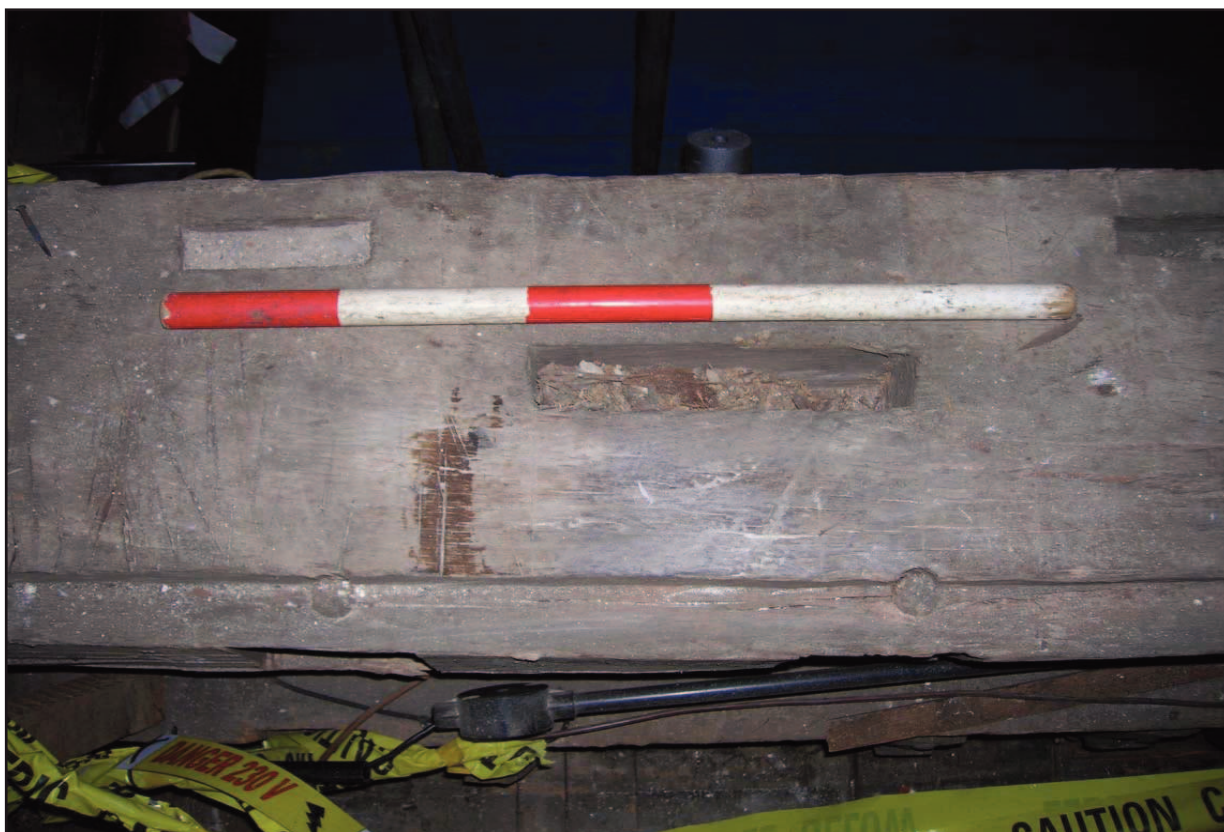
Plate 14: Royal Pew, Chapel Royal, Hampton Court Palace: Royal Pew, further mortices and floorboard rebate surviving on the top surface of the upper primary beam.
