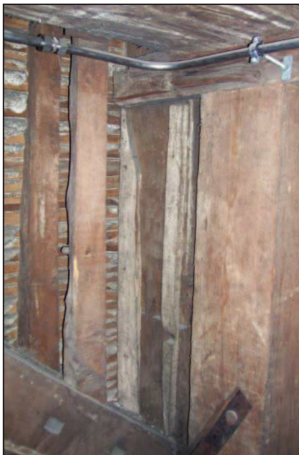
Plate 62: Royal Pew, Chapel Royal, Hampton Court Palace: Void over Thornhill ceiling. Surviving Tudor post and 17th century supporting post strapped in front of it (north side). The Tudor post is chamfered on the closest edge and is recessed in two places halfway up the photograph.
