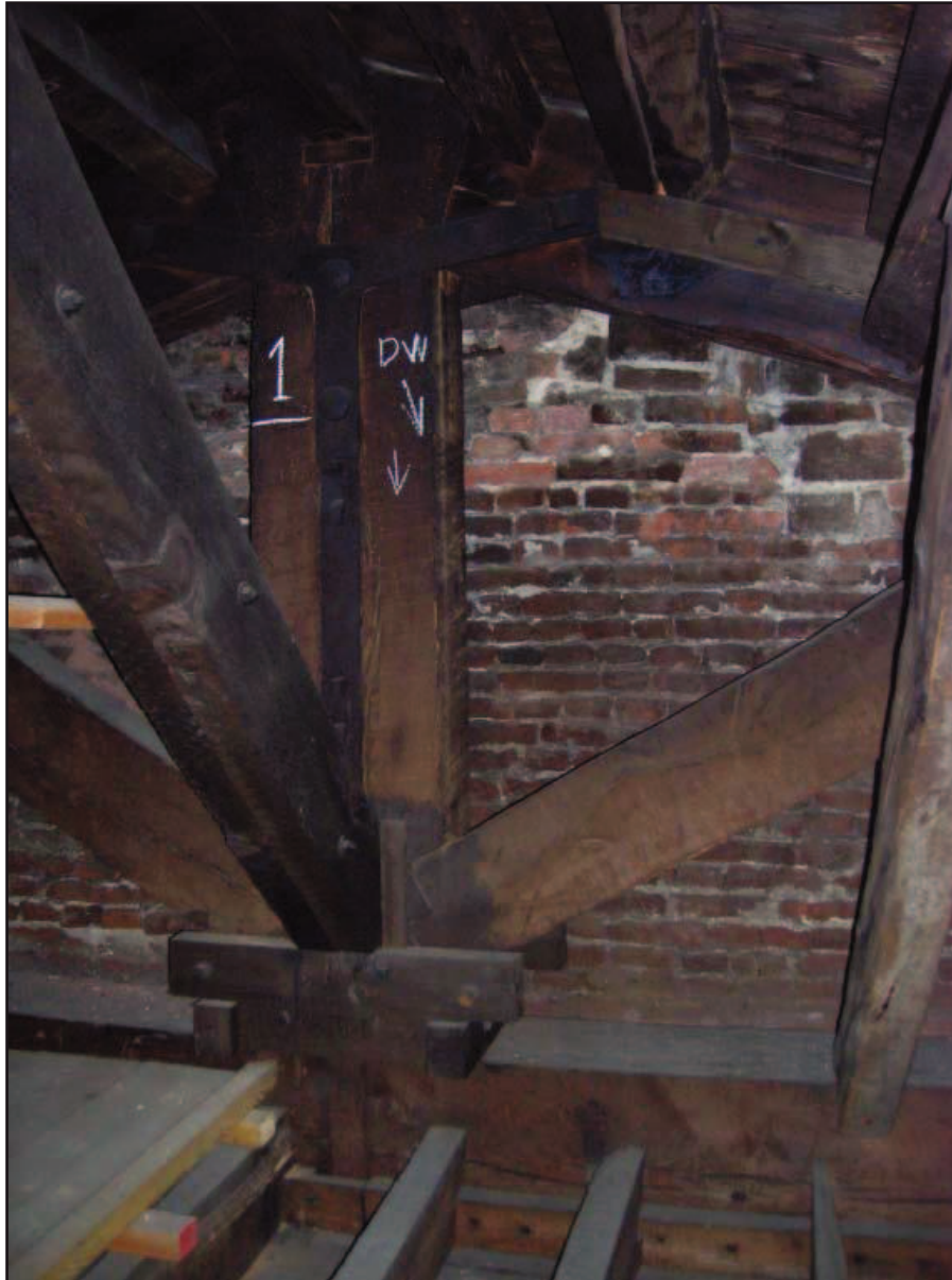
Plate 38: Royal Pew, Chapel Royal, Hampton Court Palace: Roof space over the Royal Pew, south elevation showing brick detail and King post truss.
