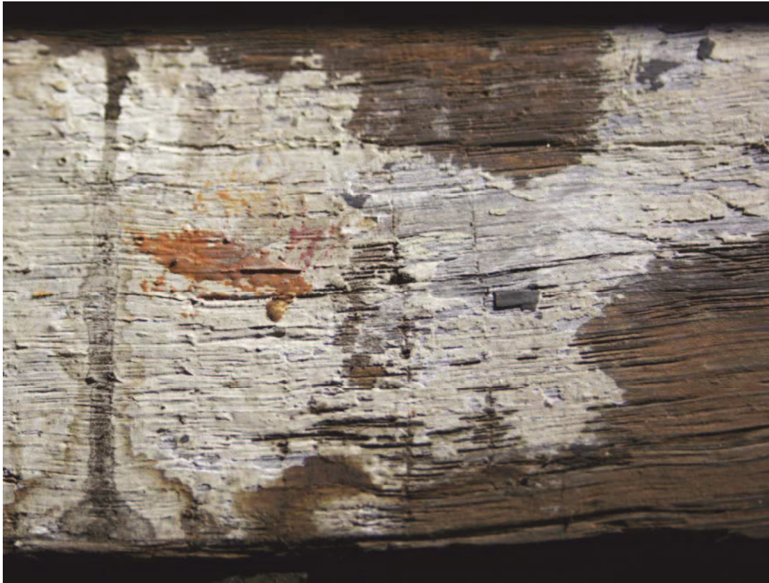
Plates 4 & 5: details of the white preparation surviving on the east face of the balcony beam. The random dribs and daubs of other colours (black, red, dark yellow ochre and gold) are visible. Note widespread losses in the white layer and losses to the black drips.
