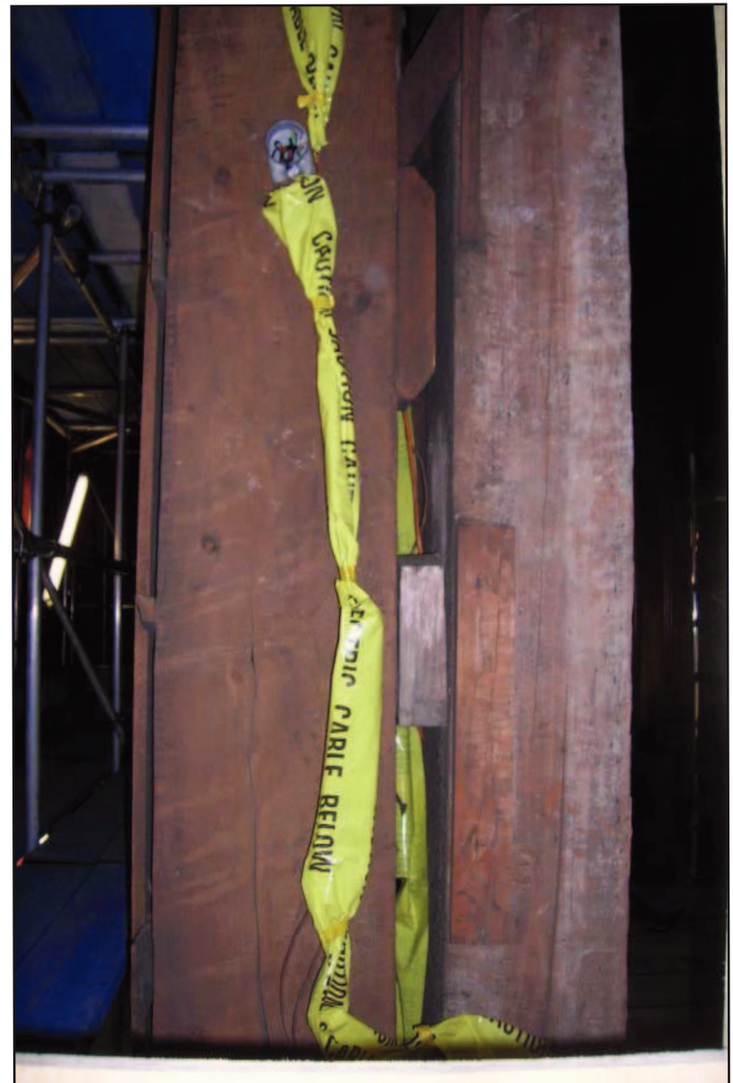
Plate 17: Royal Pew, Chapel Royal, Hampton Court Palace: Royal Pew, detail of 17th century upright and iron brace attached to main pew structure.
