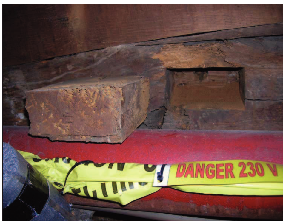
Plate 15: Royal Pew, Chapel Royal, Hampton Court Palace: Royal Pew, detail of a mortice relating to the possible Oriel window (south end).
