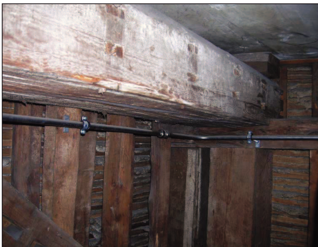
Plate 55: Royal Pew, Chapel Royal, Hampton Court Palace: Void over Thornhill Ceiling, east elevation, substantial re-used timber running in front of east elevation.
