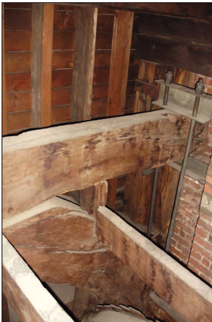
Plate 44: Royal Pew, Chapel Royal, Hampton Court Palace: Roof space over the Chapel Royal, Hampton Court Palace. Detail of the 17th century (?) truss in the north west corner of the Chapel Royal roof space, forming part of the overall framework of the Royal Pew structure.
