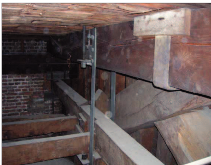
Plate 45 : Royal Pew, Chapel Royal, Hampton Court Palace: Roof space over Chapel Royal. View to the south showing details of truss and 'u' support.
