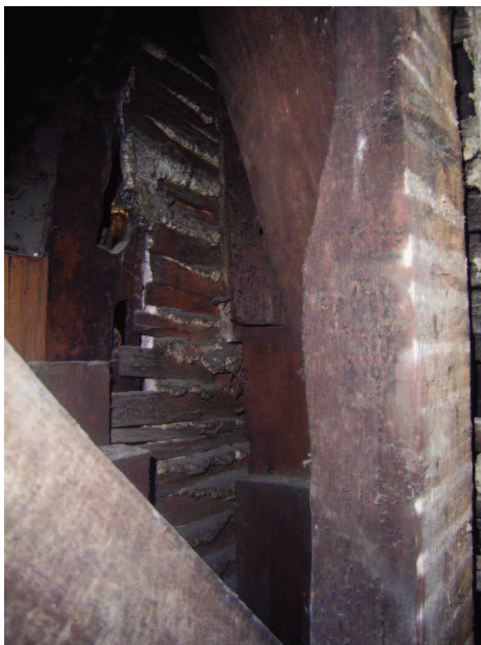
Plate 52: Royal Pew, Chapel Royal, Hampton Court Palace: Hidden room above Winter Pew, east elevation following removal of plaster, rebates on post 3 for possible arch.
