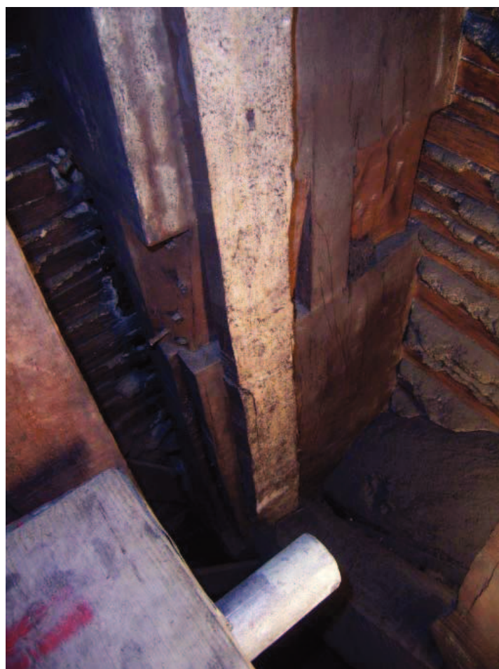
Plate 61: Royal Pew, Chapel Royal, Hampton Court Palace: Void over Thornhill ceiling, rebates for possible arch detail on post 3
