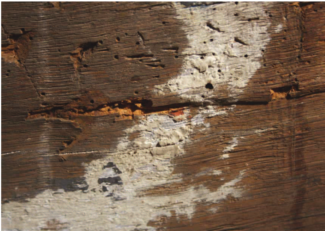
Plates 4 & 5: details of the white preparation surviving on the east face of the balcony beam. The random dribs and daubs of other colours (black, red, dark yellow ochre and gold) are visible. Note widespread losses in the white layer and losses to the black drips.
