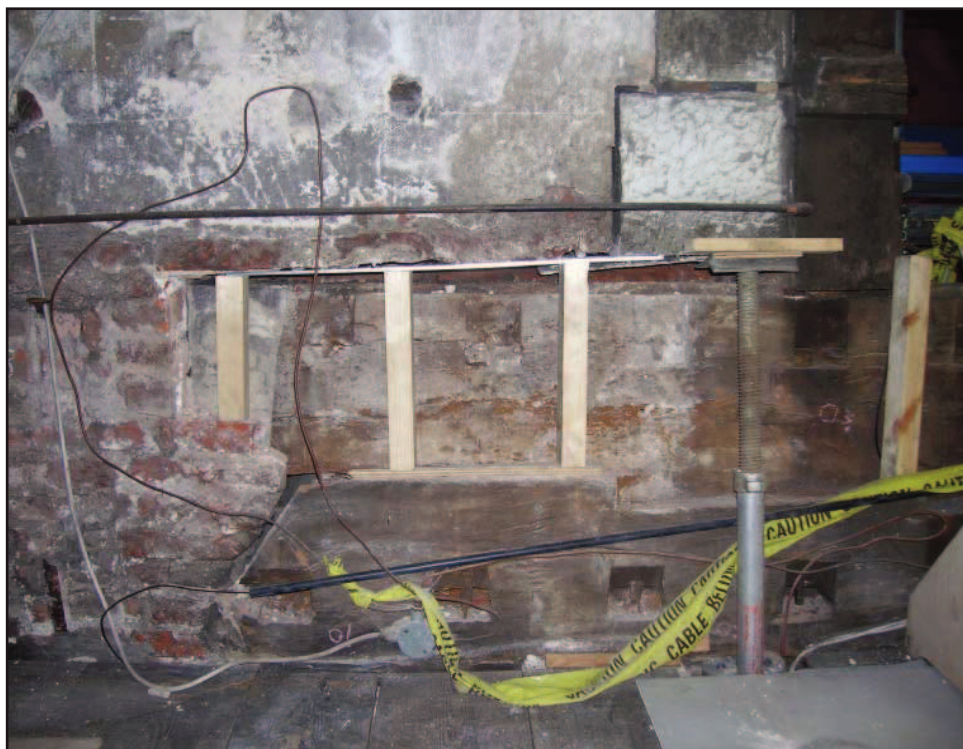
Plate 32: Royal Pew, Chapel Royal, Hampton Court Palace: Royal Pew, west elevation (south), detail of beam in ante chapel wall on removal of brickwork.
