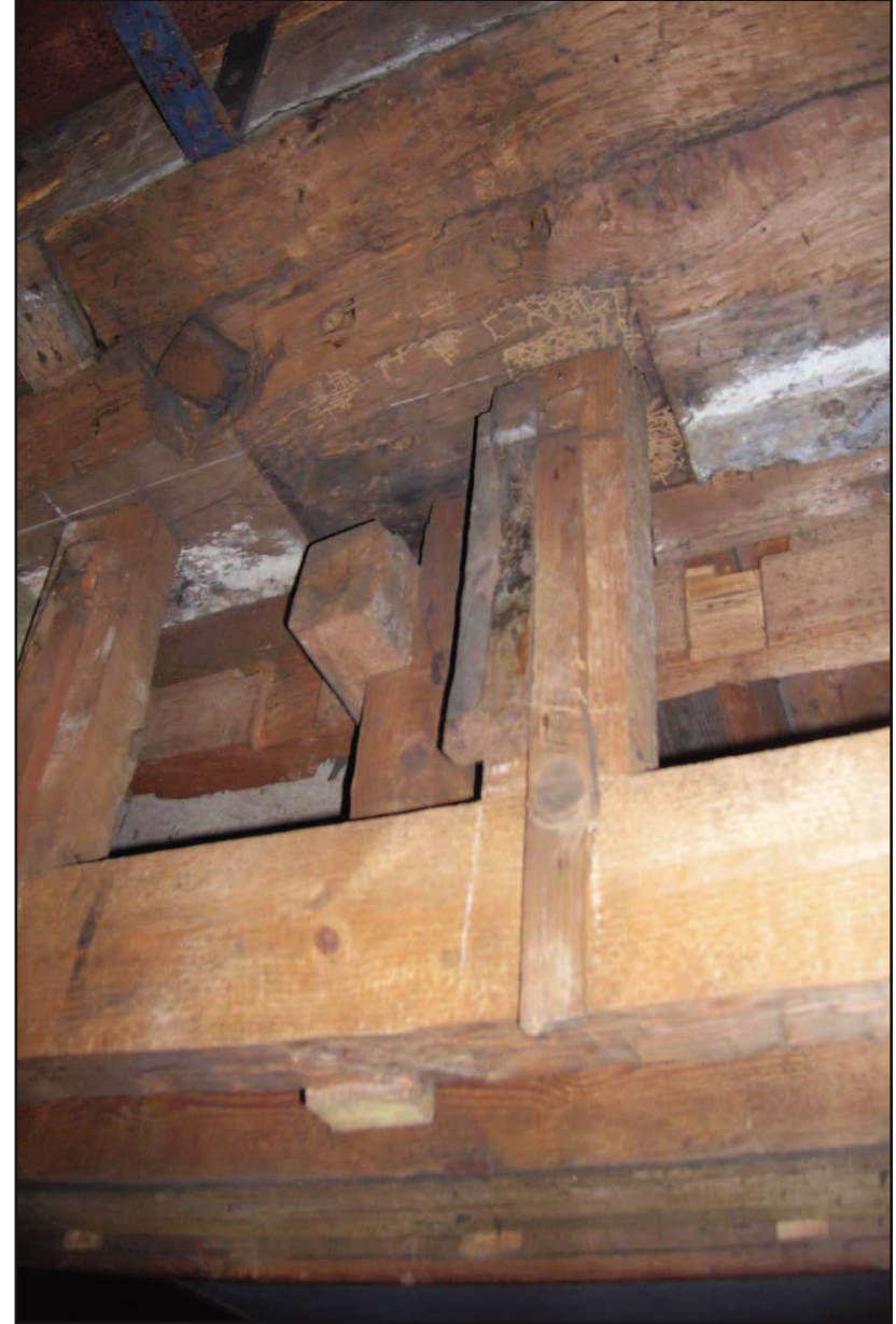
Plate 29: Royal Pew, Chapel Royal, Hampton Court Palace: Royal Pew, soffitt of lower primary beam showing peg holes and mortice for earlier
