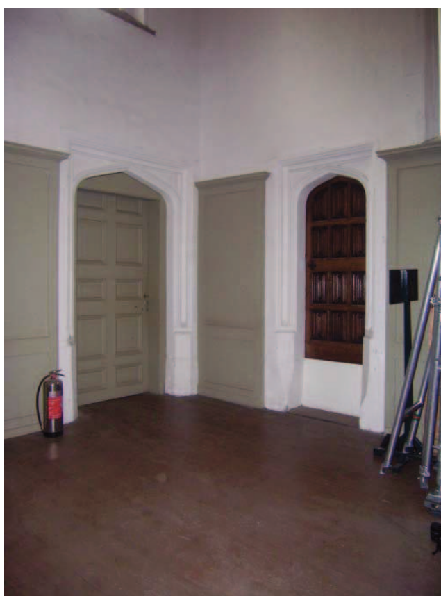
Plate 11: Royal Pew, Chapel Royal, Hampton Court Palace: Royal Pew, model room, primary phase doorways to Royal Pew. The left doorway was the entrance to the pew and the doorway on the right was for the vice stair leading down to the chapel. Note the difference in floor height.
