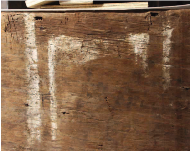
Plate 6: detail of the vertical tracks within the white preparation on the east face of the balcony beam at the base of former post 2. Similar traces are visible on the north side of the beam, at the base of former post 6.
