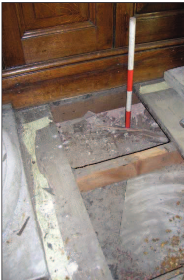
Plate 68: Royal Pew, Chapel Royal, Hampton Court Palace: Royal Pew, lifting of the floorboards on the south side of the ante chapel. Detail of floor joist and marble floor tiles.
