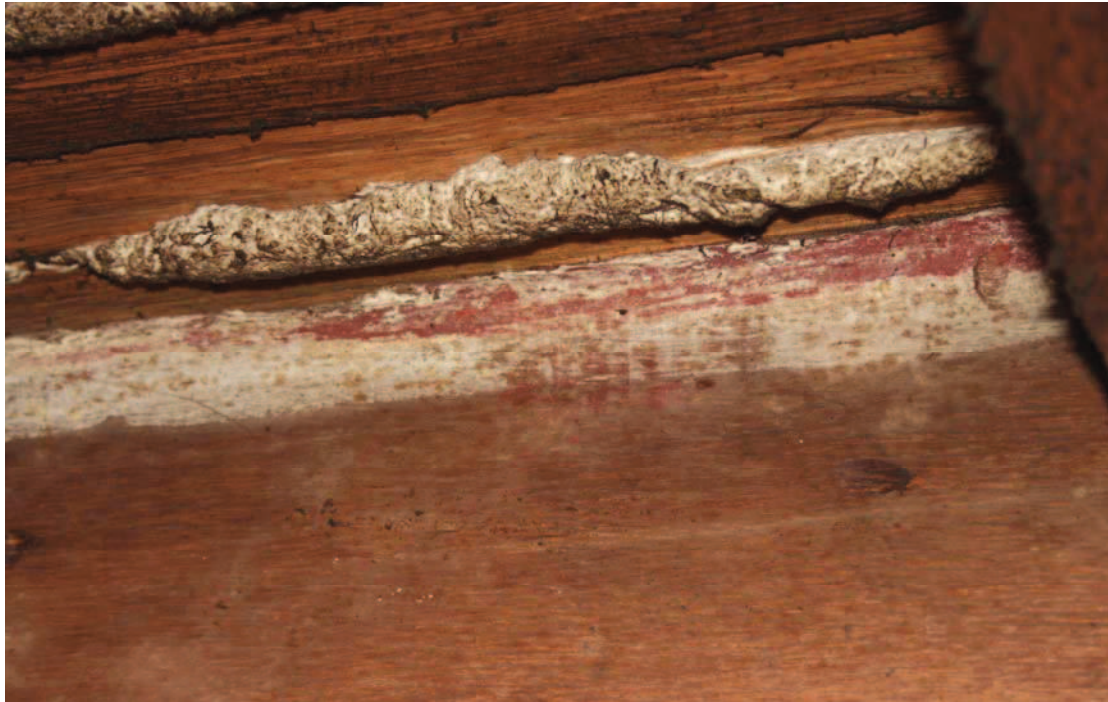
Plate 8: detail of red decoration on the north bracing beam (above the Thornhill ceiling) showing an intentional edge – the limit of the decoration. See Plate 2
