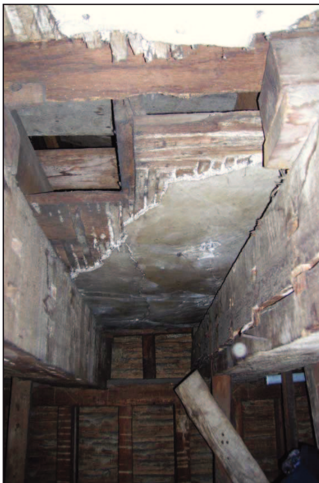
Plate 56: Royal Pew, Chapel Royal, Hampton Court Palace: Void over Thornhill ceiling, view to the north revealing surviving elements of the former plaster ceiling.
