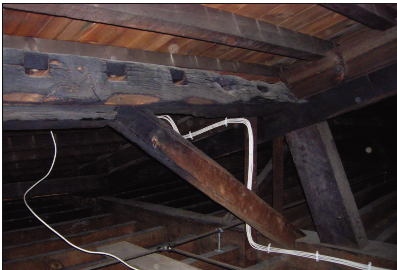
Plate 41: Royal Pew, Chapel Royal, Hampton Court Palace: Roof space over the Royal Pew, east side, detail of re-used timbers as primary purlin.
