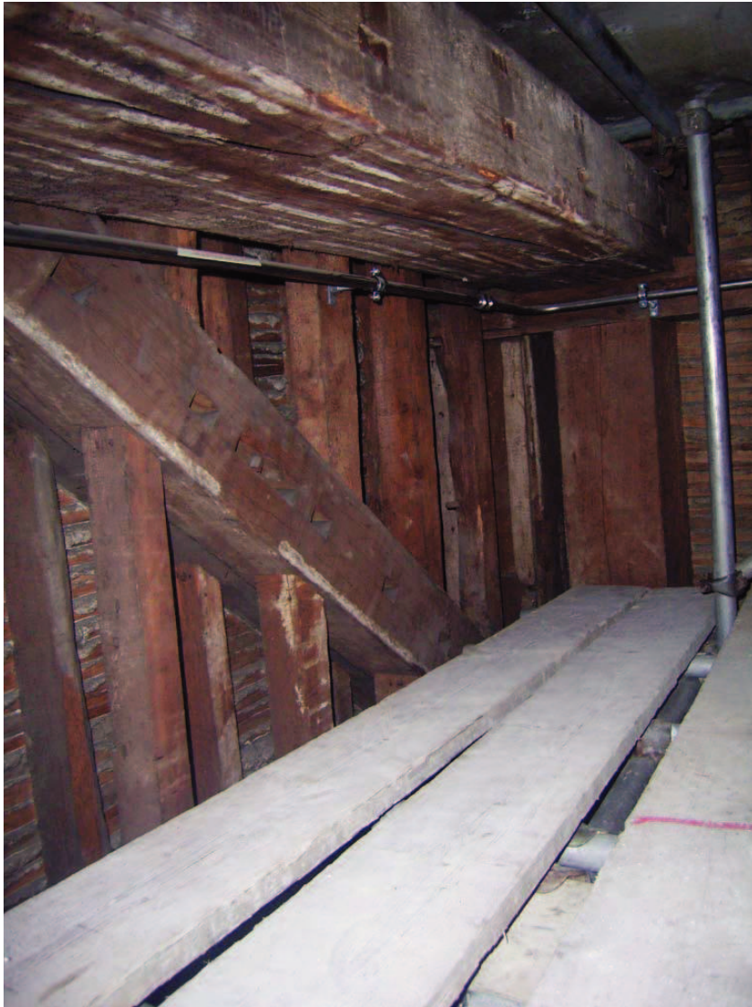
Plate 58: Royal Pew, Chapel Royal, Hampton Court Palace: Void over Thornhill ceiling, west elevation reset brace (south) with empty mortices and paint traces.
