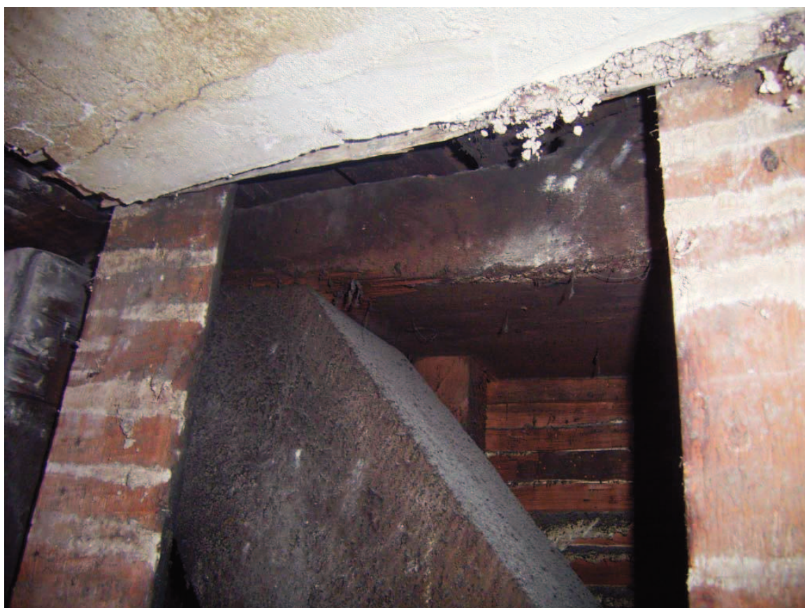
Plate 51: Royal Pew, Chapel Royal, Hampton Court Palace: Hidden room above Winter Pew, east elevation following removal of plaster, reduced Tudor wall plate.
