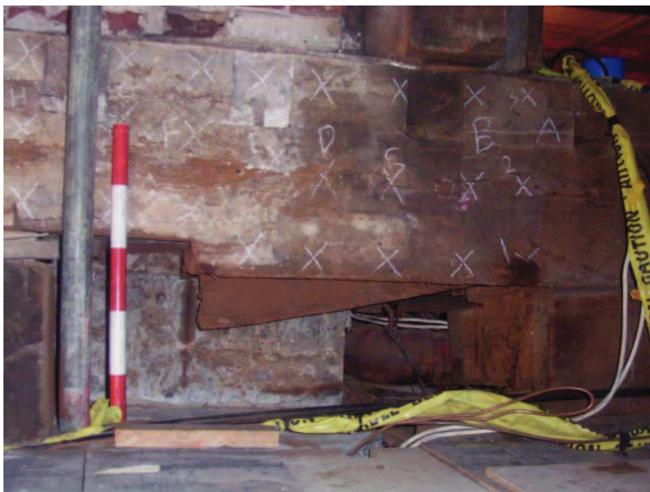
Plate 10: Royal Pew, Chapel Royal, Hampton Court Palace: Royal Pew, west elevation, detail of tenon following removal of lower beam
