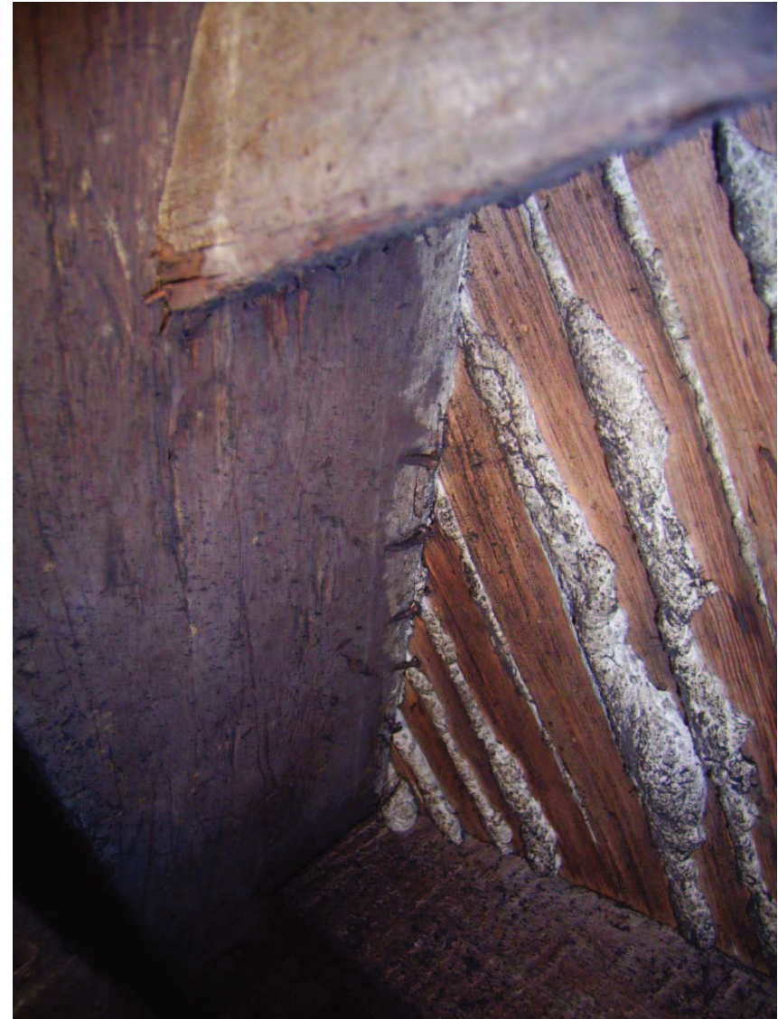
Plate 59: Royal Pew, Chapel Royal, Hampton Court Palace: Void over Thornhill ceiling, detail of paint on inside of northern brace with nails and looping evidence for material fixing.
