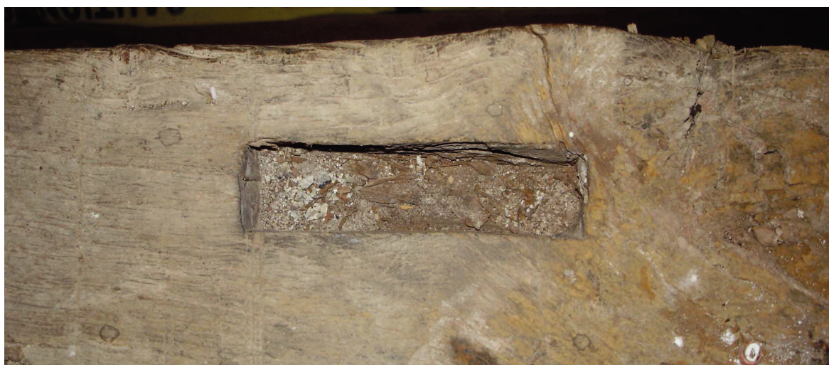
Photograph of mortice in upper gallery beam for missing upright post VI in Lady Chapel (D Miles)
