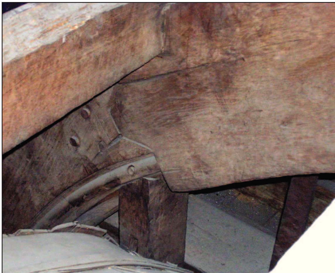
Plate 46: Roof space over Chapel Royal, detail of moulding on underside of truss at the south end.
