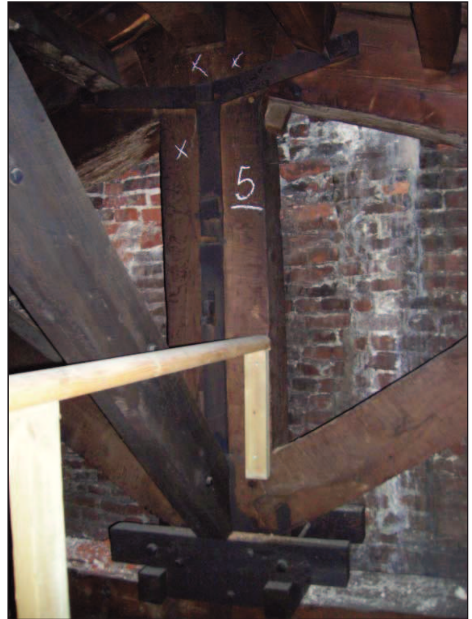
Plate 39: Royal Pew, Chapel Royal, Hampton Court Palace: Roof space over the Royal Pew, north elevation showing brick detail and King post truss.
