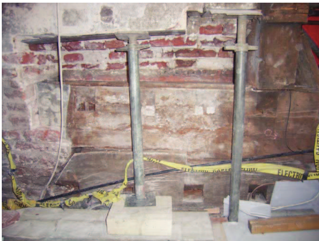
Plate 9: Royal Pew, Chapel Royal, Hampton Court Palace: Royal Pew, west elevation, primary beams extending north into ante chapel wall following removal of lower quoin and brickwork.
