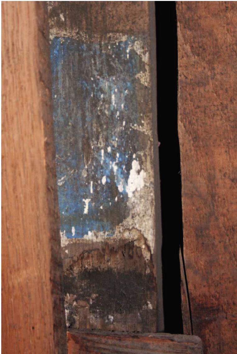
Plate 7: detail of an area of bright blue decoration on the east face of post 5 – see Plate 1. The upper edge appears intentional, suggesting a previous fixture. Note small, fresh-looking paint losses.
