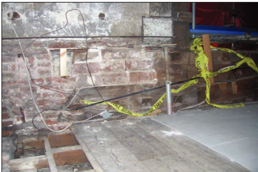
Plate 8: Royal Pew, Chapel Royal, Hampton Court Palace: Royal Pew, west elevation, primary beams extending north into ante chapel wall prior to removal of brickwork.
