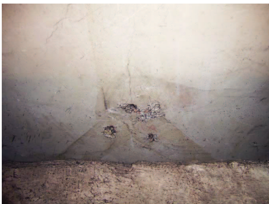
Plate 57: Royal Pew, Chapel Royal, Hampton Court Palace: Void over Thornhill ceiling, detail of ceiling moulding fixing point on former plaster ceiling. The lines are scored and the central boss location is marked with red paint
