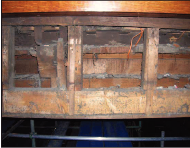
Plate 24: Royal Pew, Chapel Royal, Hampton Court Palace: Royal Pew, east elevation, detail of re-used floorboards at the south end of the main structure.
