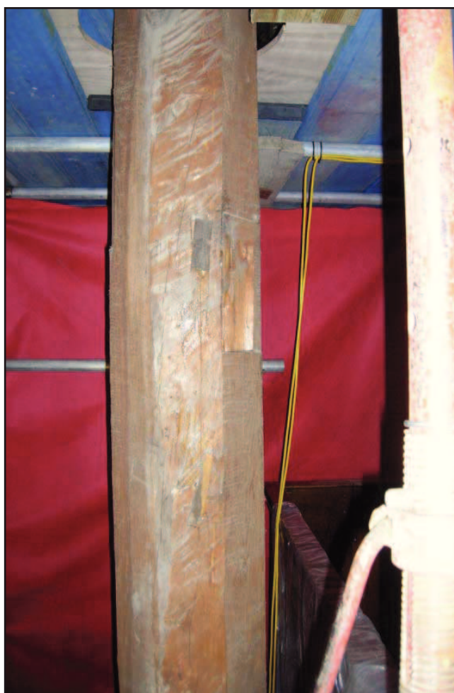
Plate 27: Royal Pew, Chapel Royal, Hampton Court Palace: Royal Pew, octagonal supporting column (south), detail of mortice for screen.
