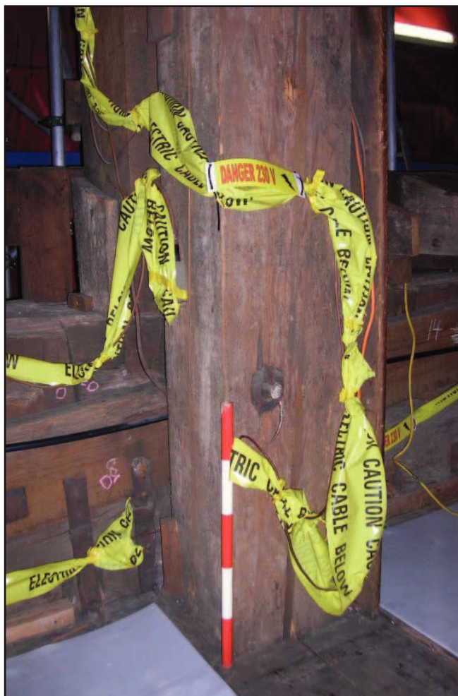
Plate 18: Royal Pew, Chapel Royal, Hampton Court Palace: Royal Pew, detail of forelock used to attached 17th century upright to main pew structure.
