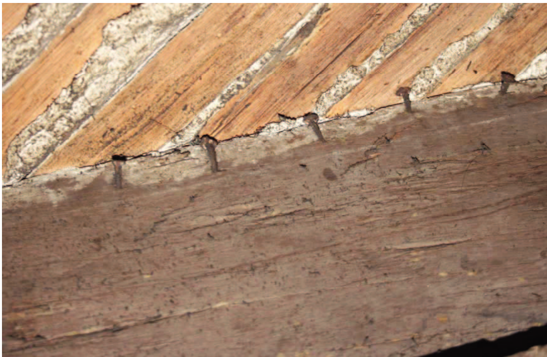
Plate 9: detail of the surviving nails with the outline where a cloth was formerly attached, south bracing beam (above the Thornhill ceiling). See Plate 2
