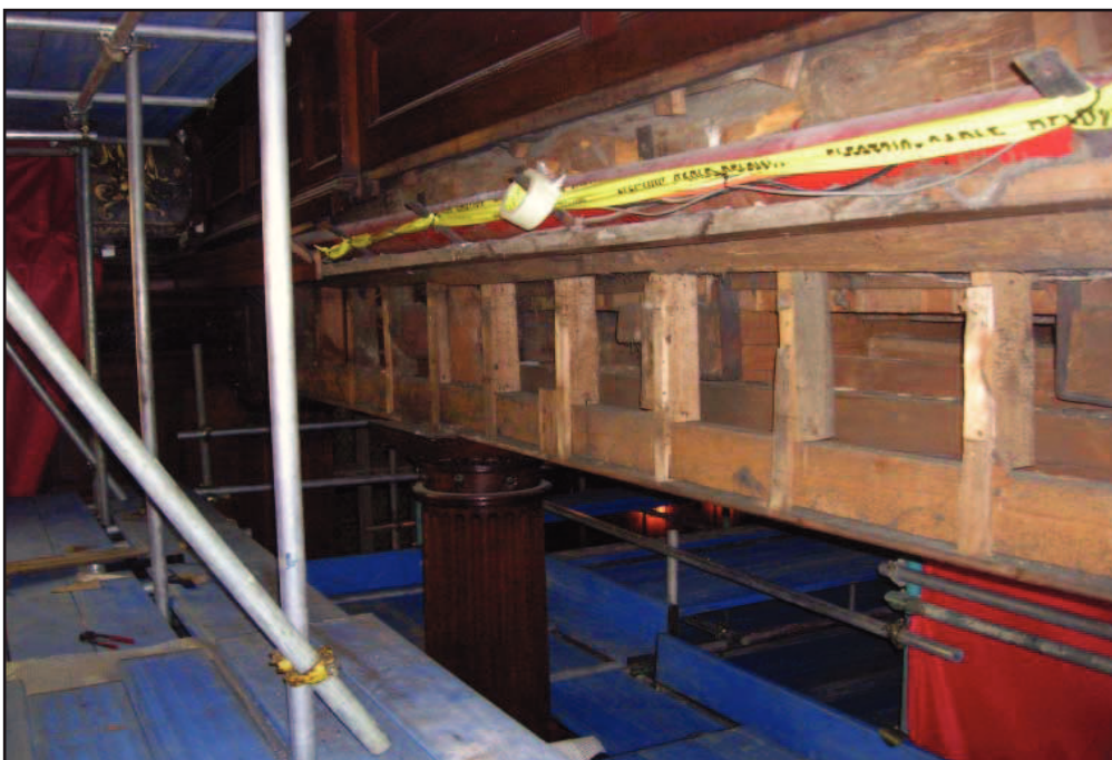
Plate 26: Royal Pew, Chapel Royal, Hampton Court Palace: Royal Pew, east elevation viewed south, overall detail of the lower softwood structure.
