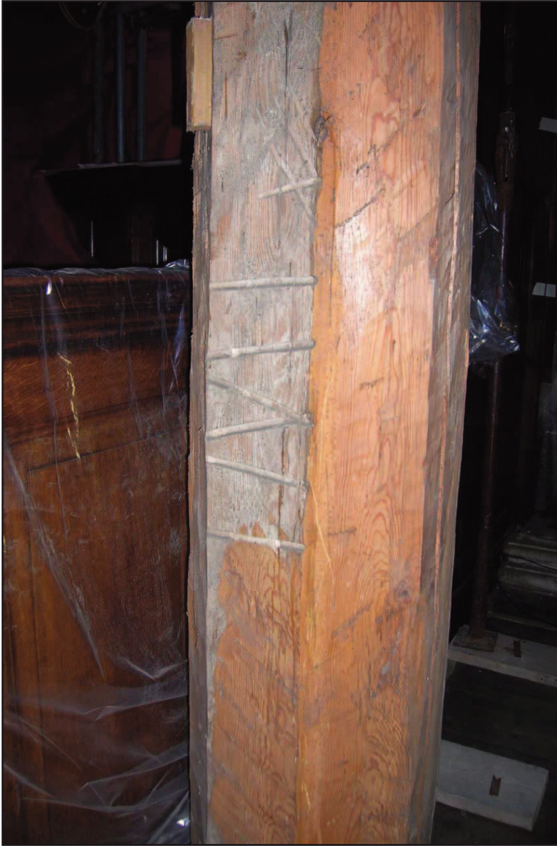
Plate 28: Royal Pew, Chapel Royal, Hampton Court Palace: Royal Pew, octagonal supporting column (north), detail of markings on north face.
